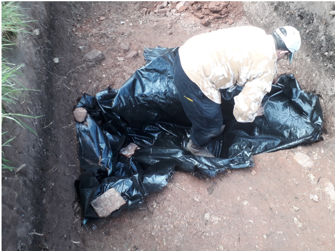
Figure 6: Structural remains being covered with Teram prior to backfilling.
