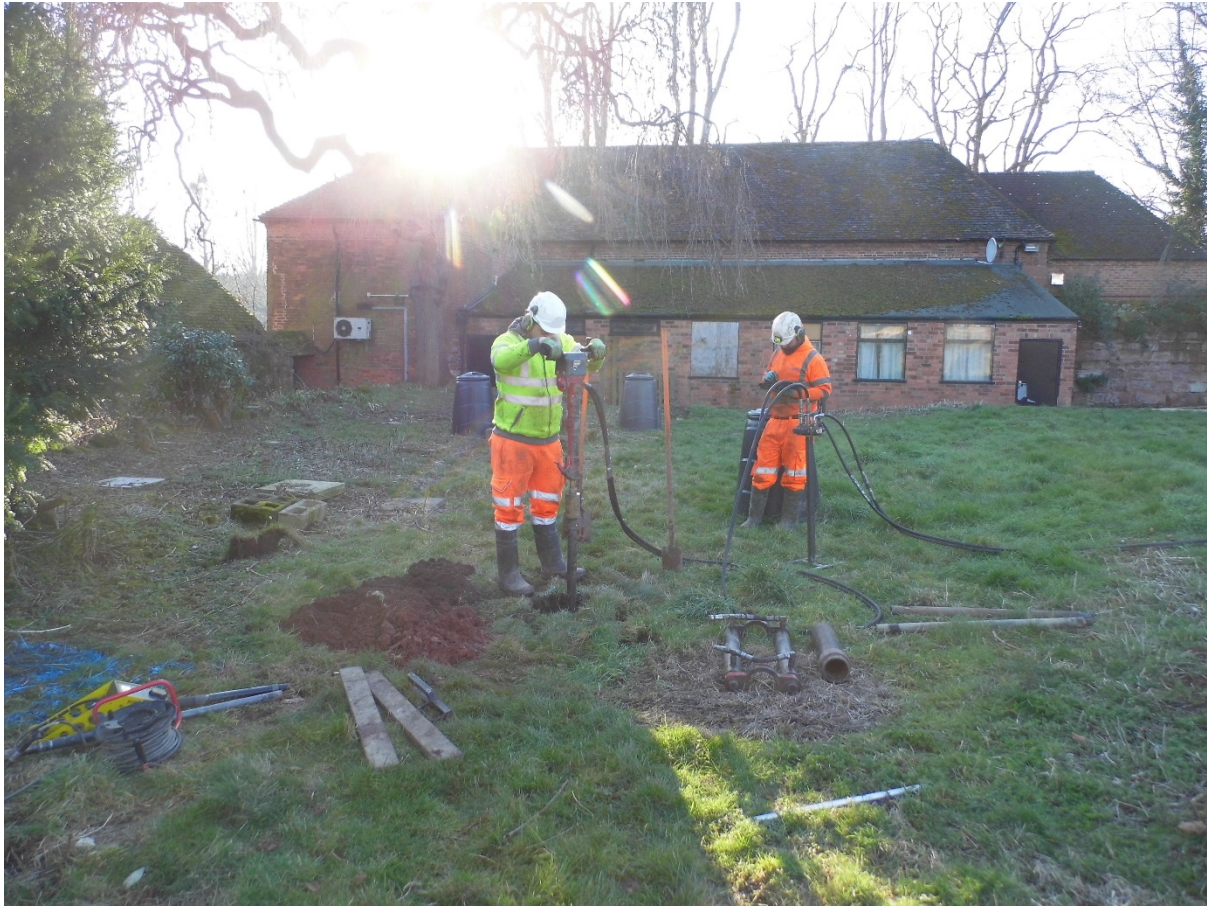
Figure 12: Excavation of Window Sample 4.
