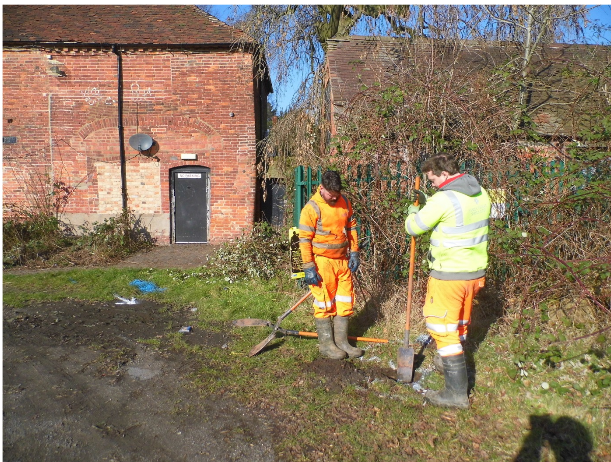
Figure 13: Excavation of Window Sample 5.
