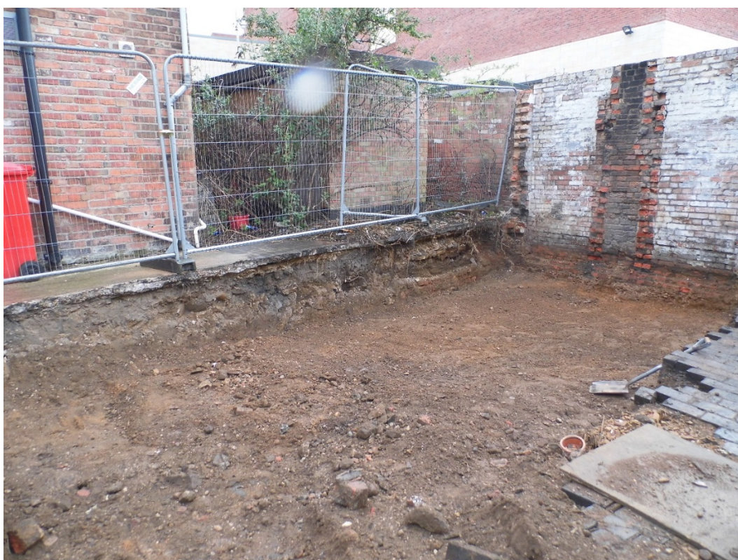
Figure 11: South-eastern corner of site.
