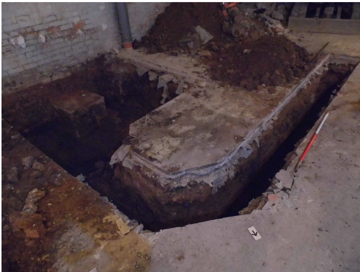
Figure 5: The excavated lift shaft and trench for the wall footing.
