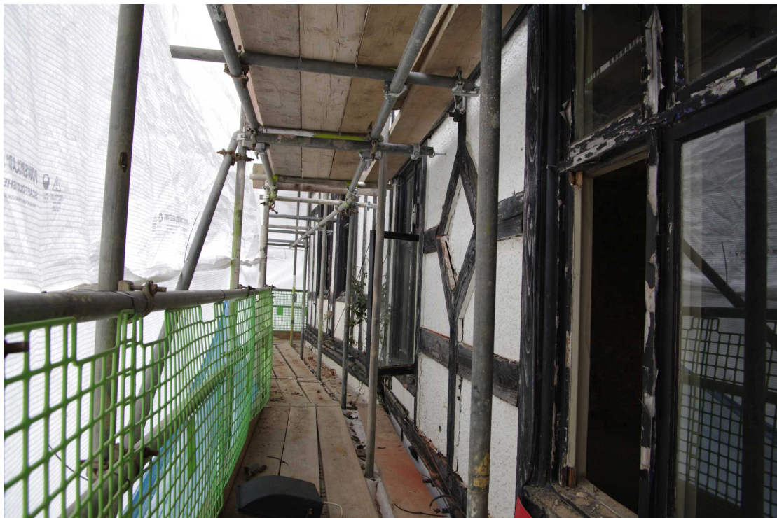
Figure 15 South facing elevation at first floor level Looking west. Note kink in building line. "Tudor" timbers are nailed into the wall
