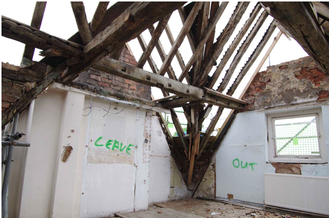
Figure 73 Room 20 Looking south-east. Lots of re-used timbers in this room
