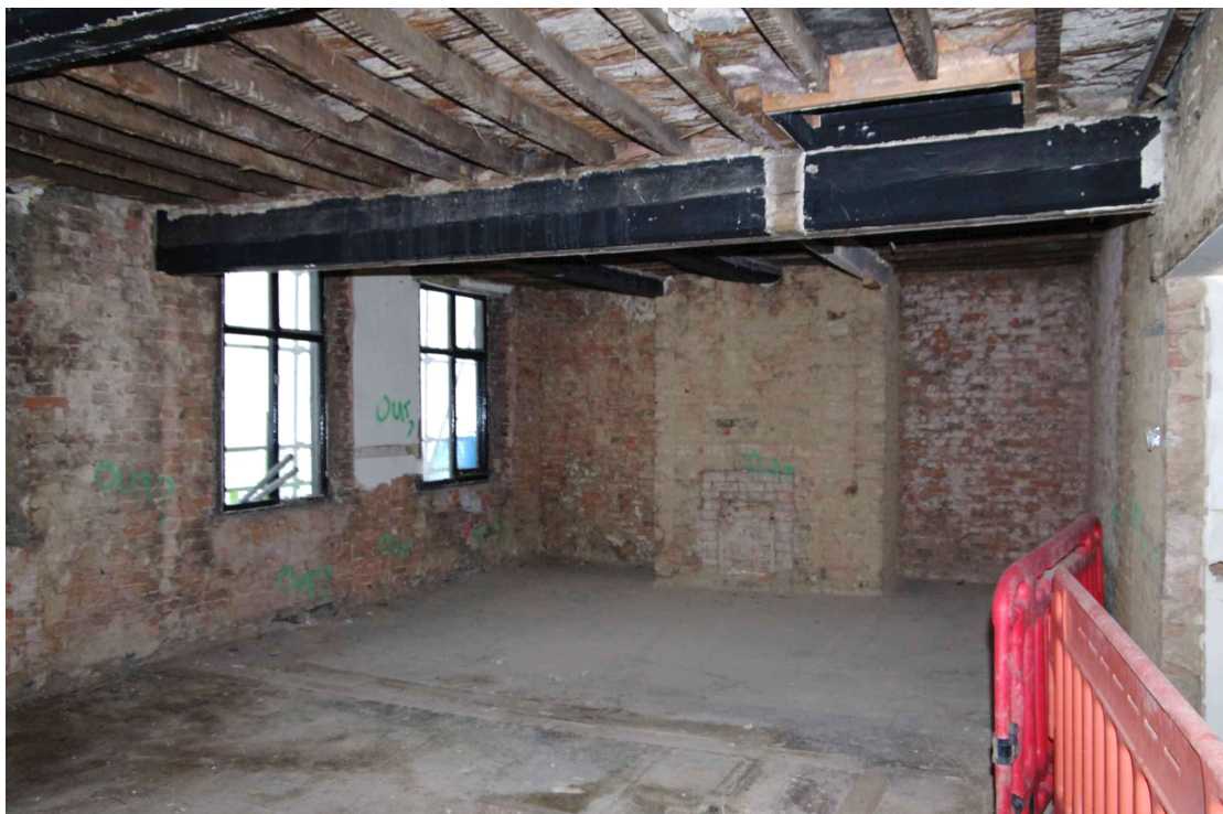
Figure 43 First floor Room 9 Looking north-west
