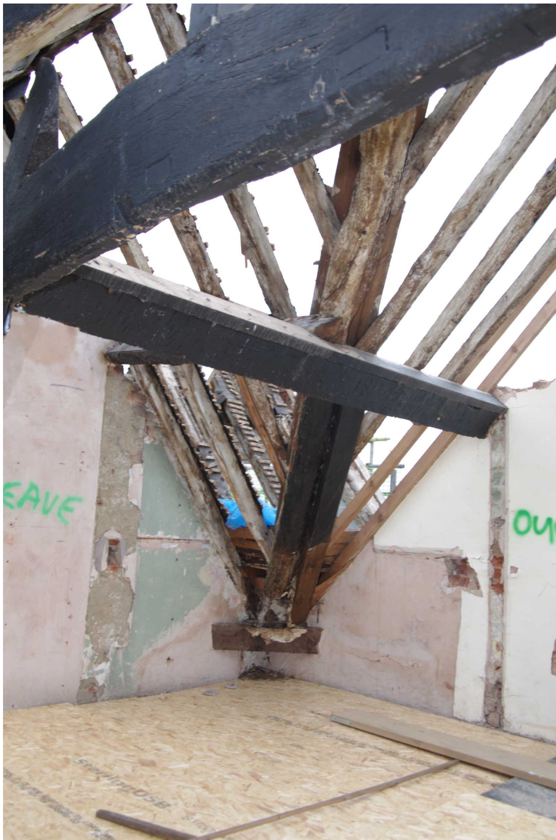
Figure 71 Room 19 corner roof structure Looking south-east
