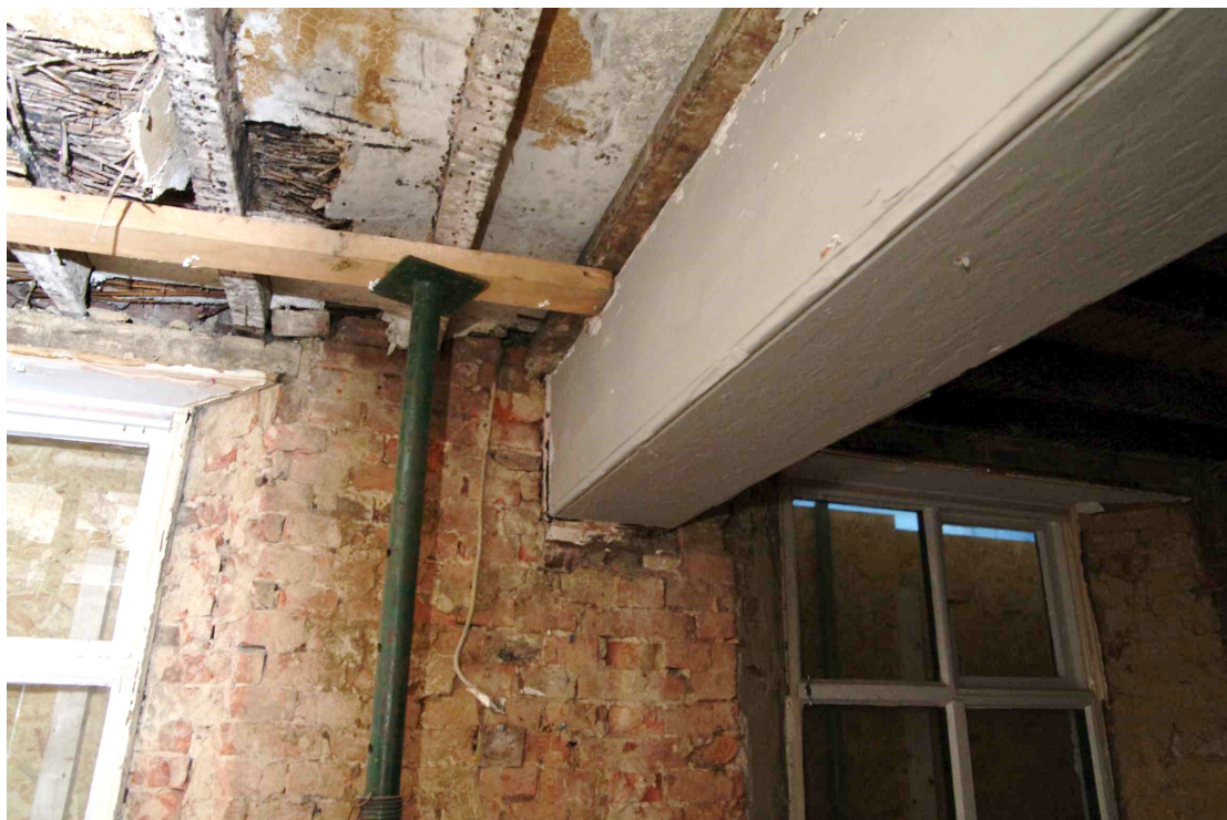
Figure 25 Beaded beam in Room 1 Looking west
