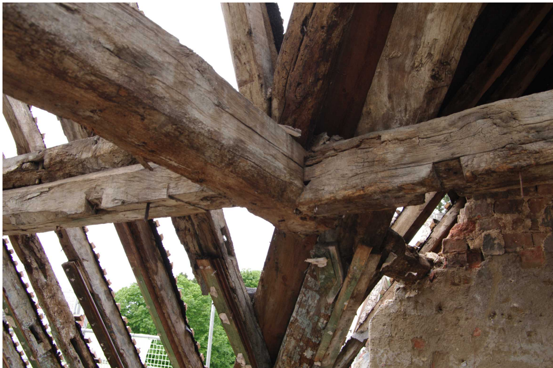
Figure 75 Room 20 joint detail in NW corner Looking west
