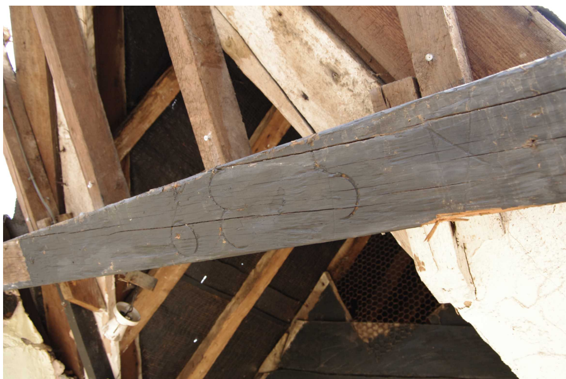
Figure 63 Room 18 marks on purlin Looking north
