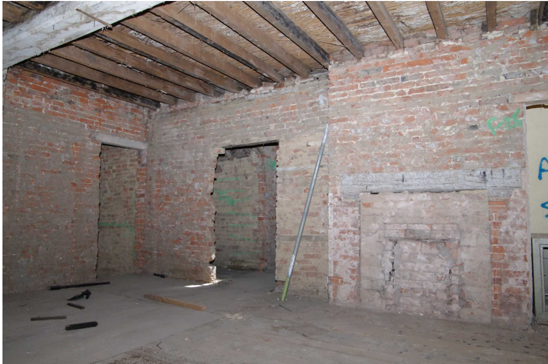
Figure 46 First floor Room 10 Looking south-east
