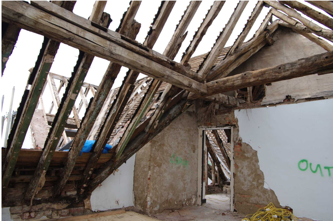
Figure 74 Room 20 Looking north-west. Note circular holes in tie-beam on right
