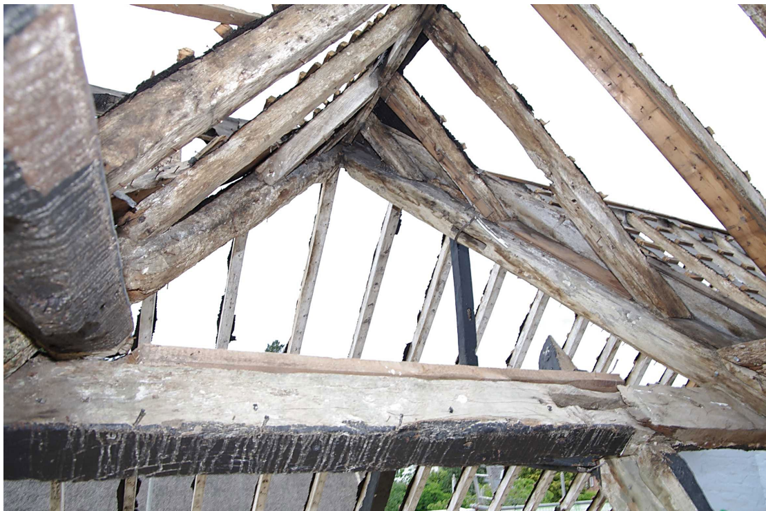
Figure 70 Room 19 roof detail Looking west. See also Figure 69 above
