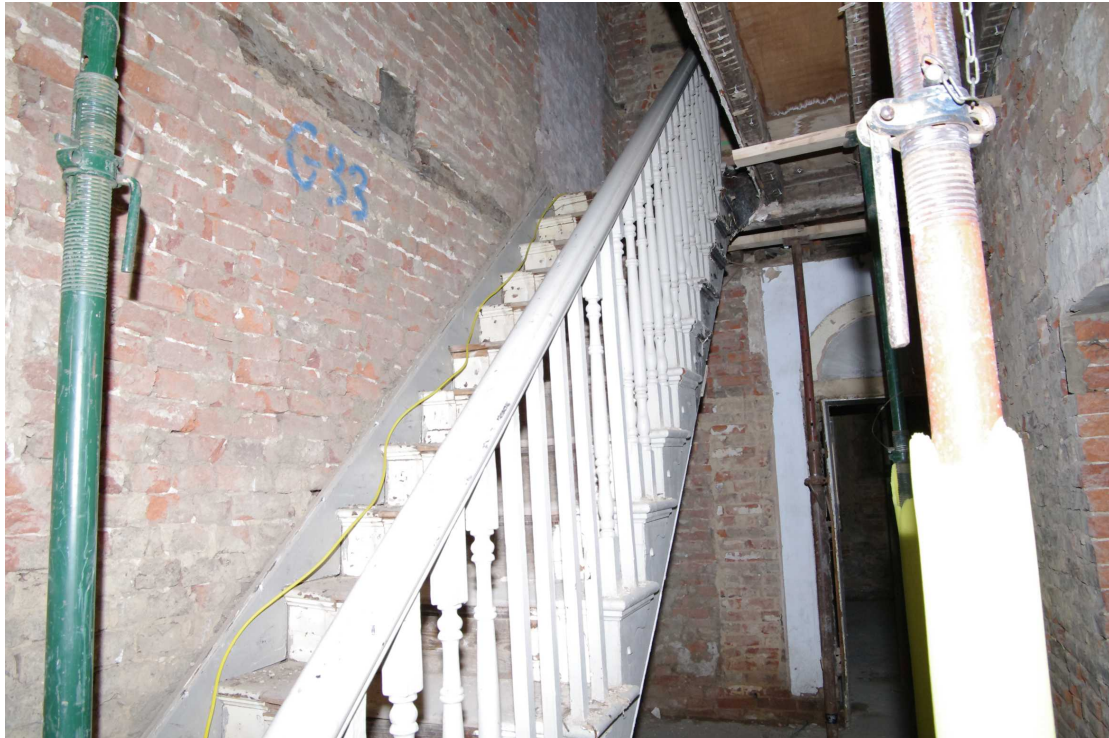
Figure 42 Staircase detail (Room 8) Looking south-west
