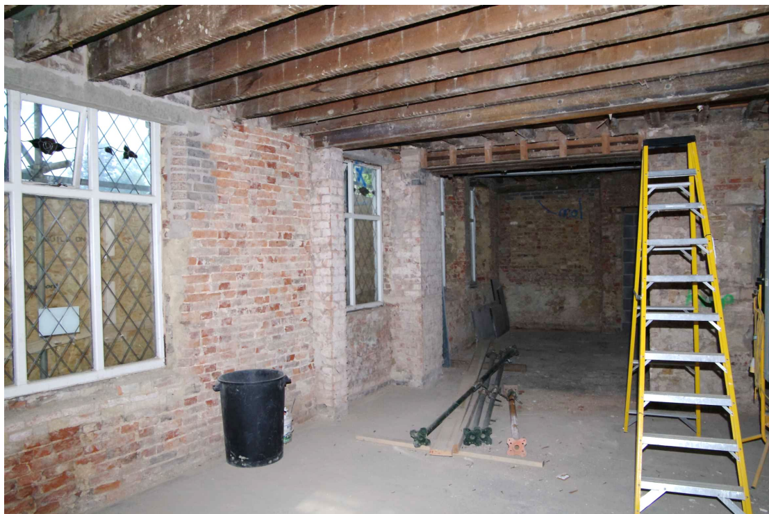
Figure 28 Southern extension Room 4 looking into Room 3 Looking west
