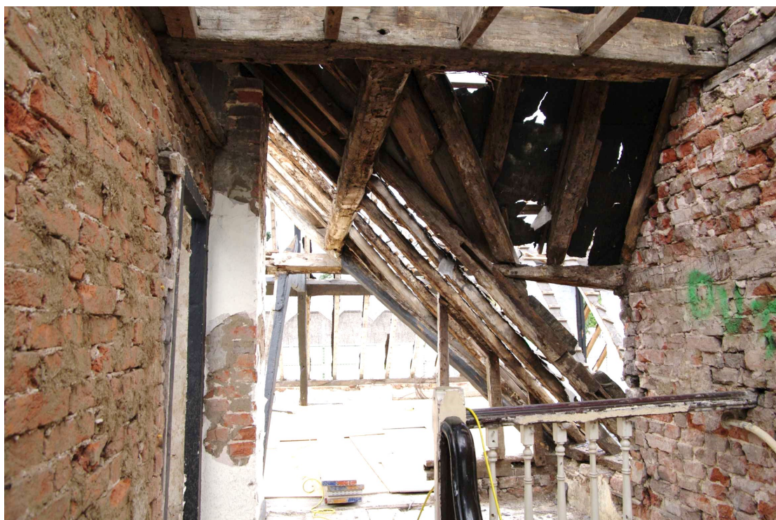
Figure 77 Room 21 top of stairs Looking west into Room 19
