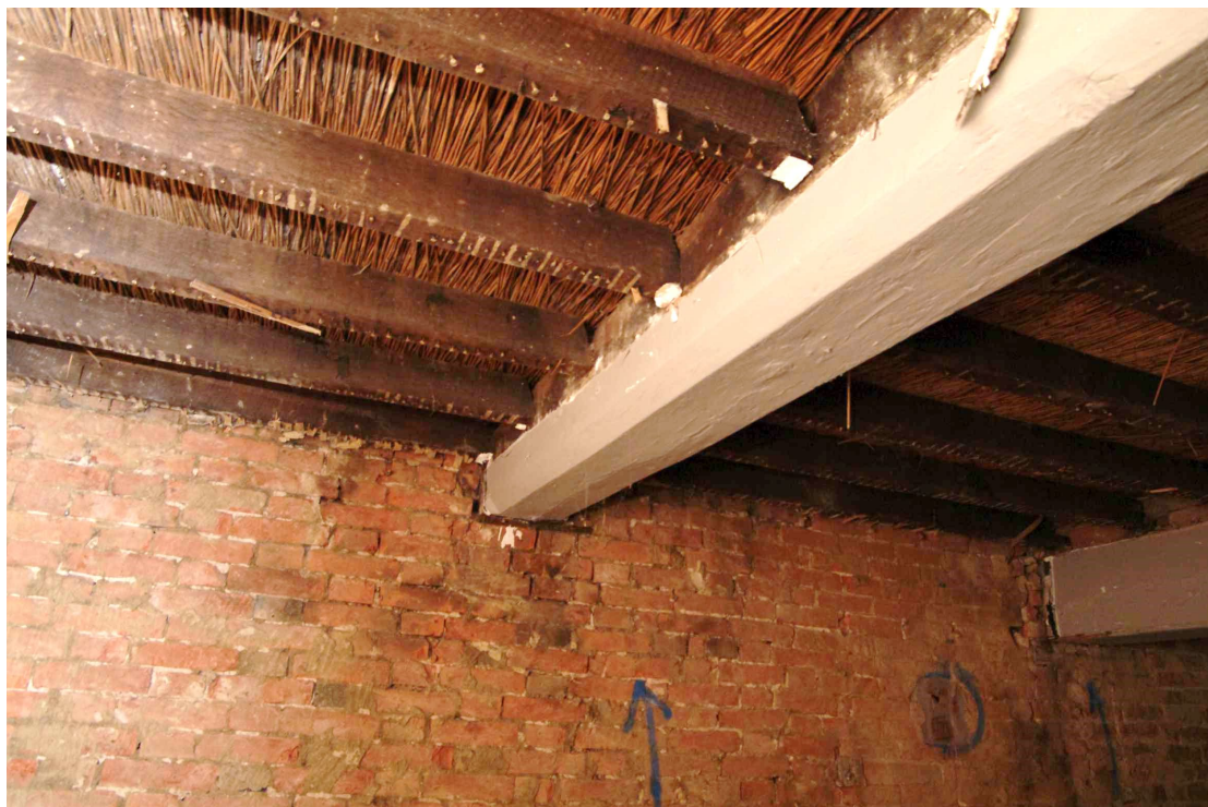
Figure 24 Stop-chamfered beam in Room 1 Looking north-east
