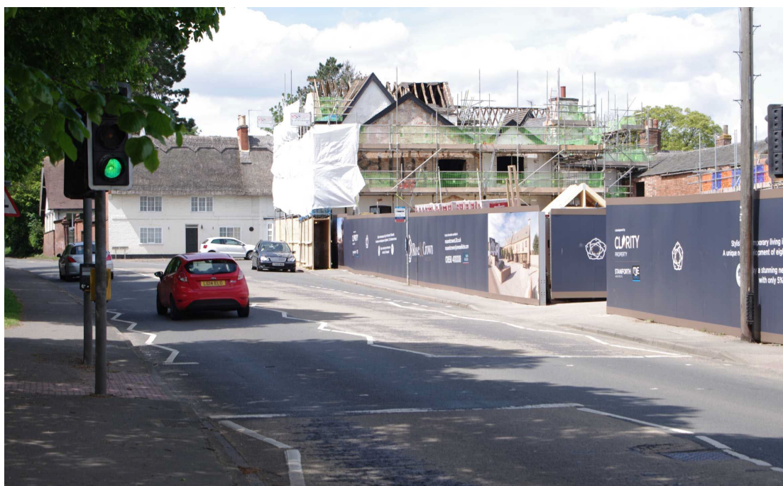
Figure 6 Site seen from Leicester Road Looking north-east
