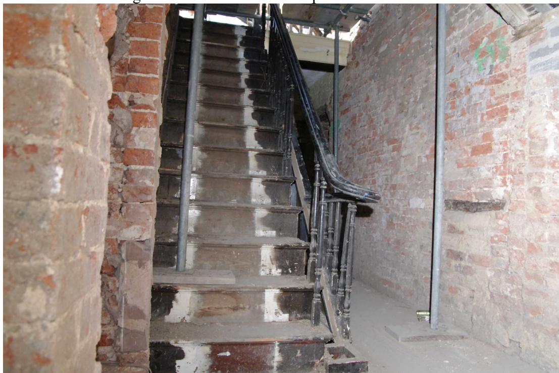
Figure 57 Stairs up to second floor Looking west
