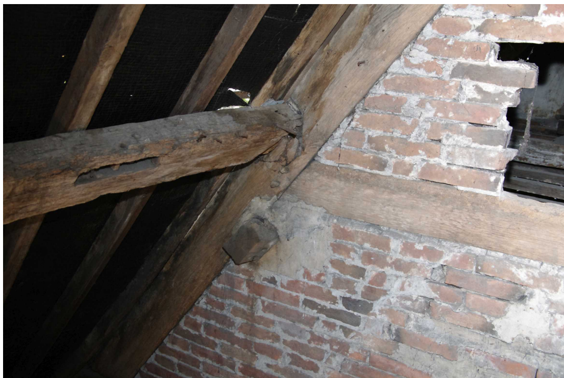
Figure 62 Pegged joints in gable seen from Room 18 Looking north-east
