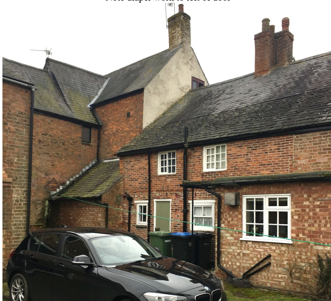
Figure 37 Diaper work and lean-to pantry before refurbishment Photograph taken in March 2018. Diaper work is just above the car roof
