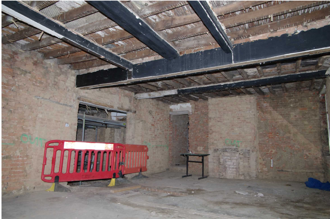
Figure 44 First floor Room 9 Looking south-east. Doorway to Room 10 centre right
