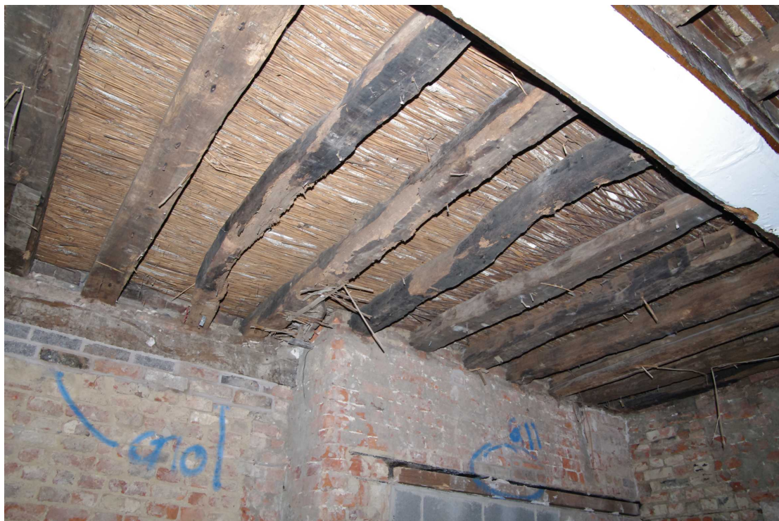
Figure 30 Room 3 ceiling details Looking north-west
