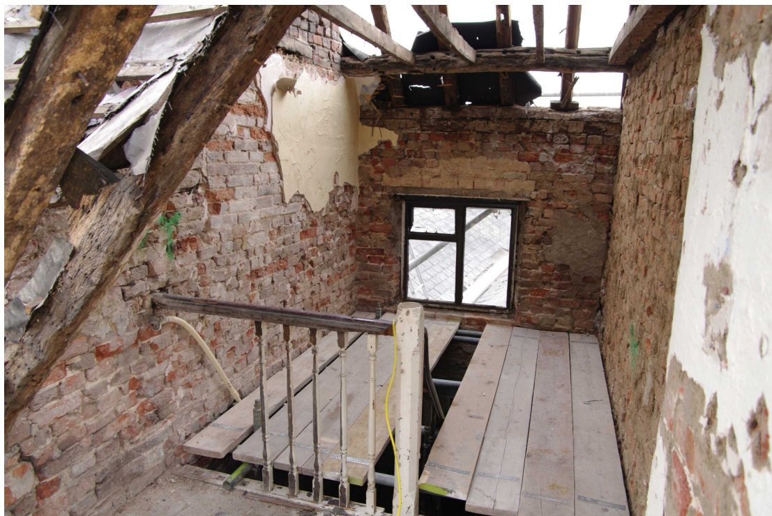
Figure 76 Room 21 top of staircase Looking east
