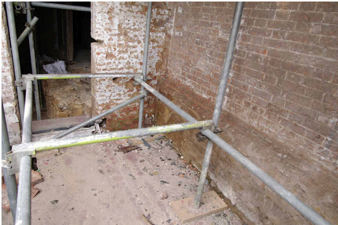
Figure 35 Outside wall of Room 5
