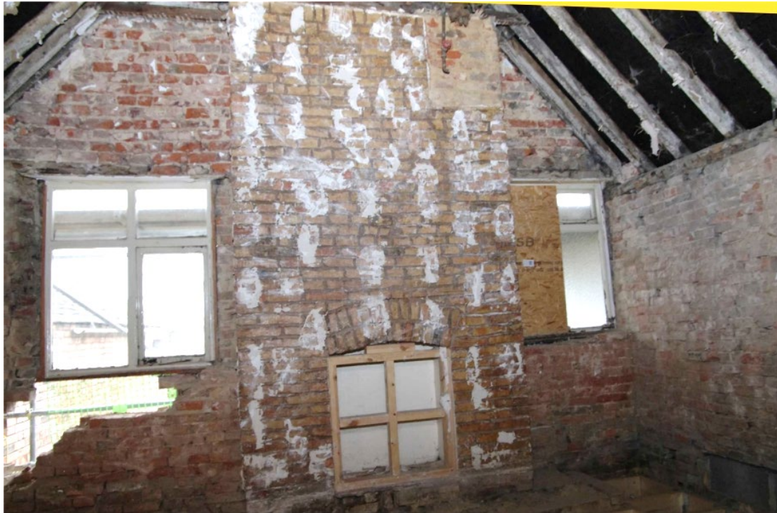
Figure 52 Room 13 after removal of floor and ceiling Looking south-east. New window to be located in central fireplace
