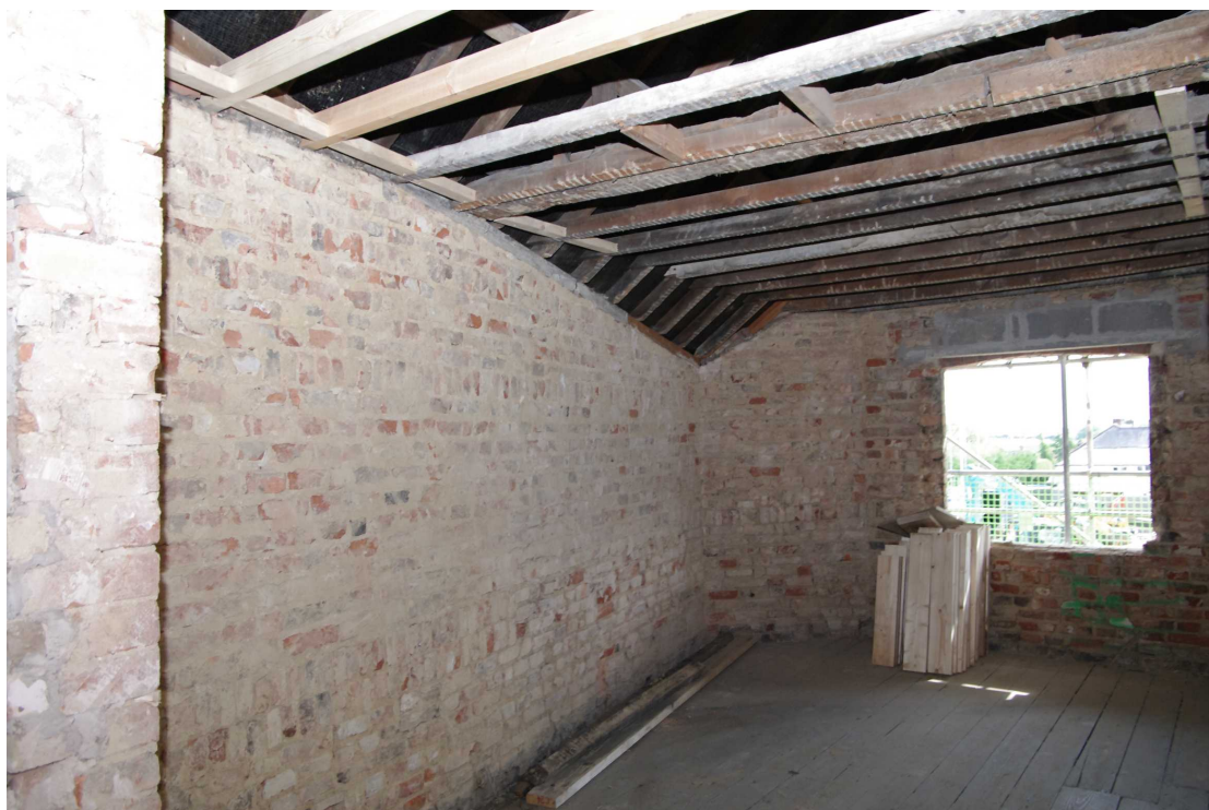
Figure 55 Room 15 Looking north-east
