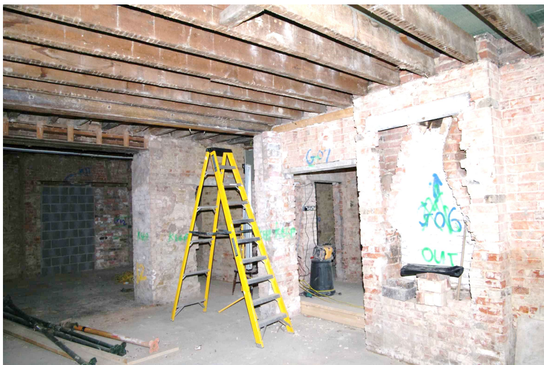
Figure 31 Rooms 3 and 4 Looking north-west from Room 4
