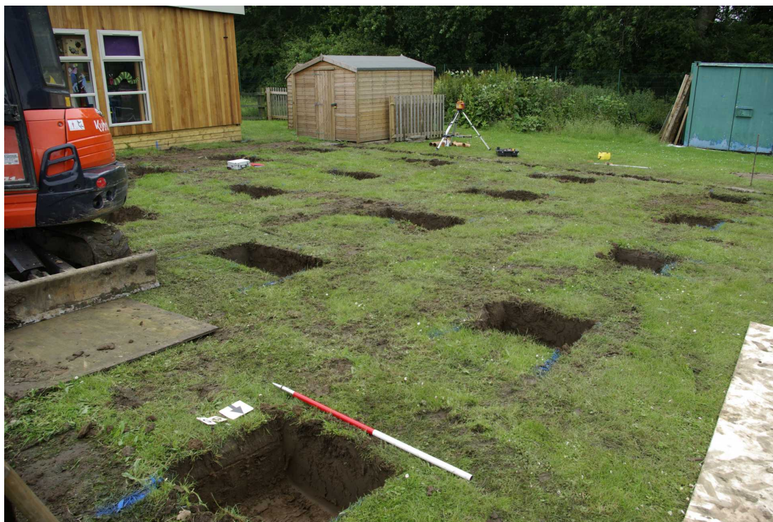
Figure 8 Fully excavated post pad pits Looking south-west
