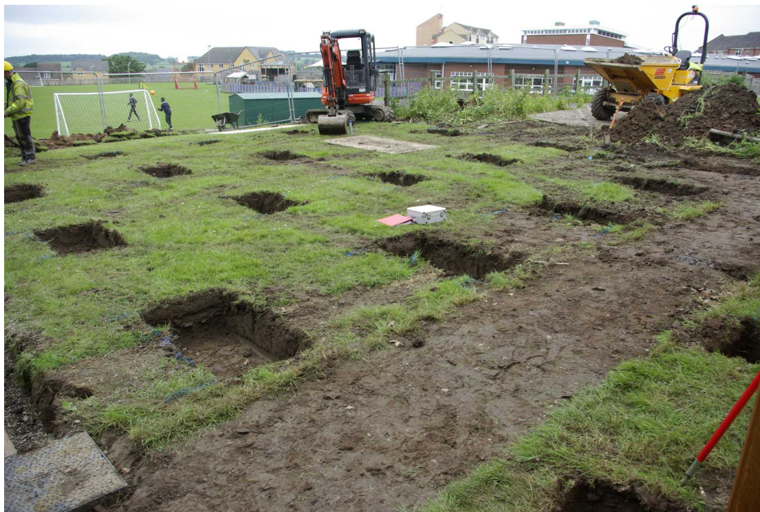
Figure 9 Fully excavated post pad pits Looking north-east
