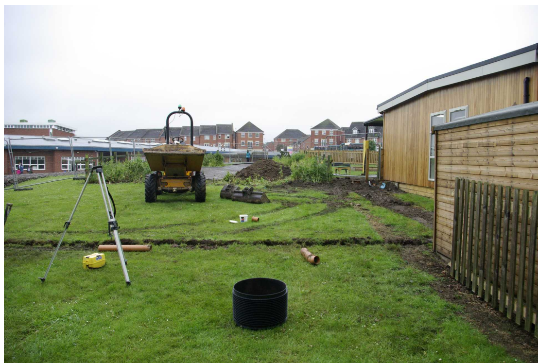
Figure 4 Site of extension before excavation
