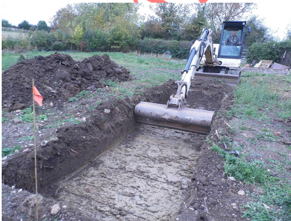
Figure 5: Excavation of the trenches.
