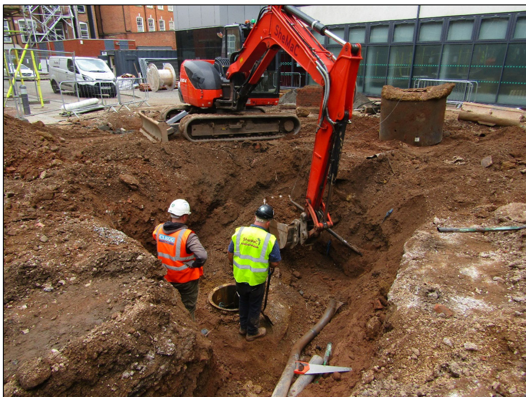
Figure 7: Exposing the large water tank looking south.
