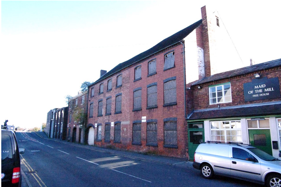
Figure 8 Coleshill Road elevation Looking east towards the canal bridge
