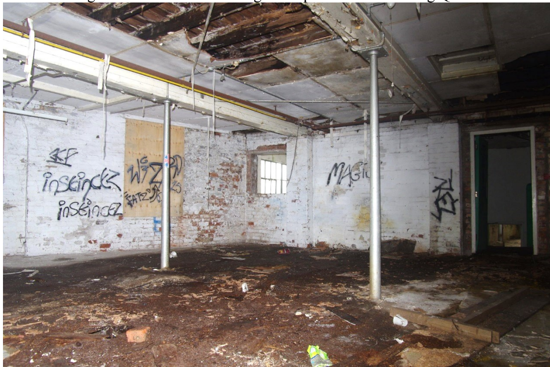
Figure 51 Building N, first floor Looking south-west towards doorway to Building F-L
