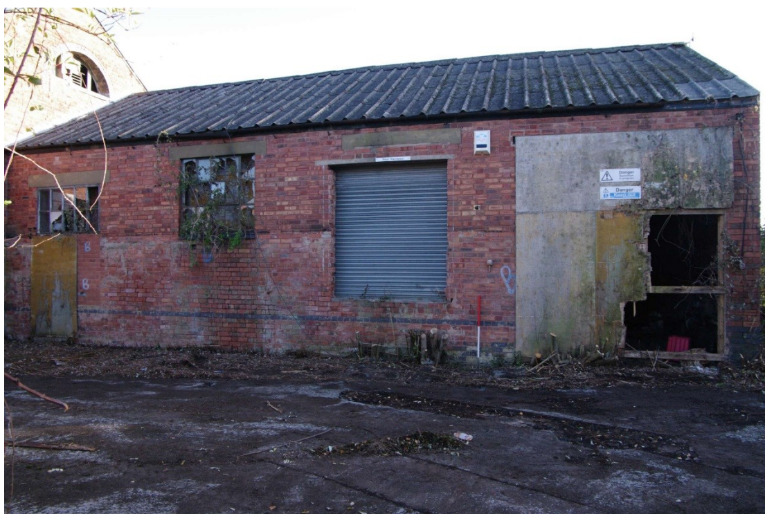
Figure 15 Building A/B south-west facing elevation Looking north-east. 1m scale
