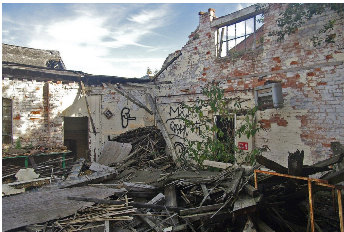
Figure 60 Building Q second floor Looking east from Building R1 doorway
