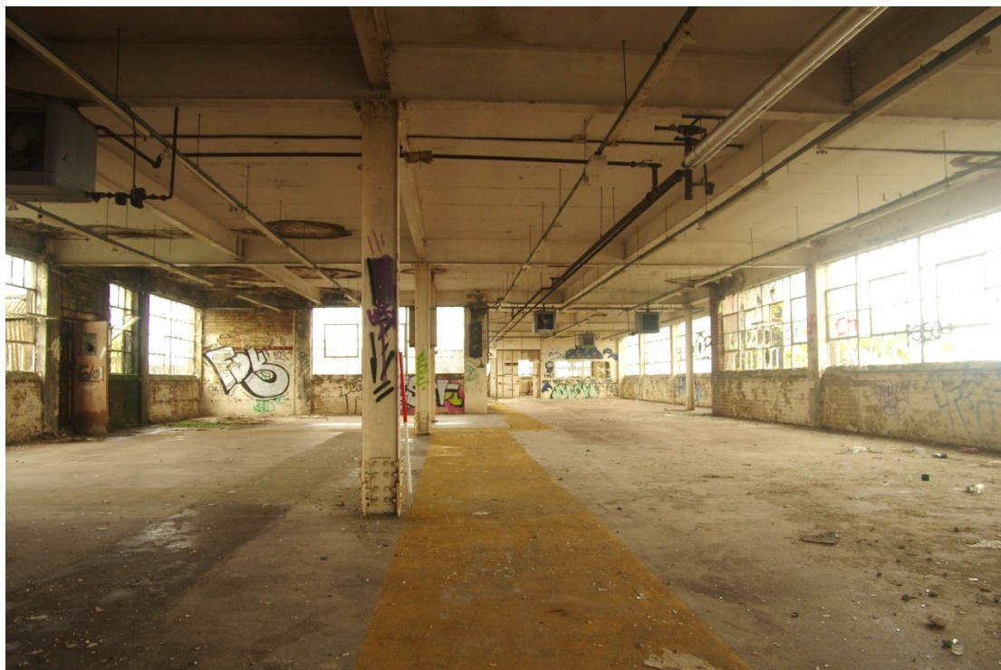
Figure 46 Building F-L second floor Looking north-west. 1m scale
