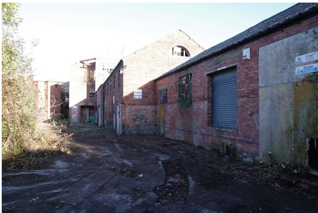
Figure 12 Yard area Looking north along canal-side buildings. Building A/B in foreground
