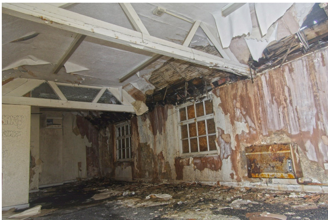
Figure 67 Building R second floor Looking west
