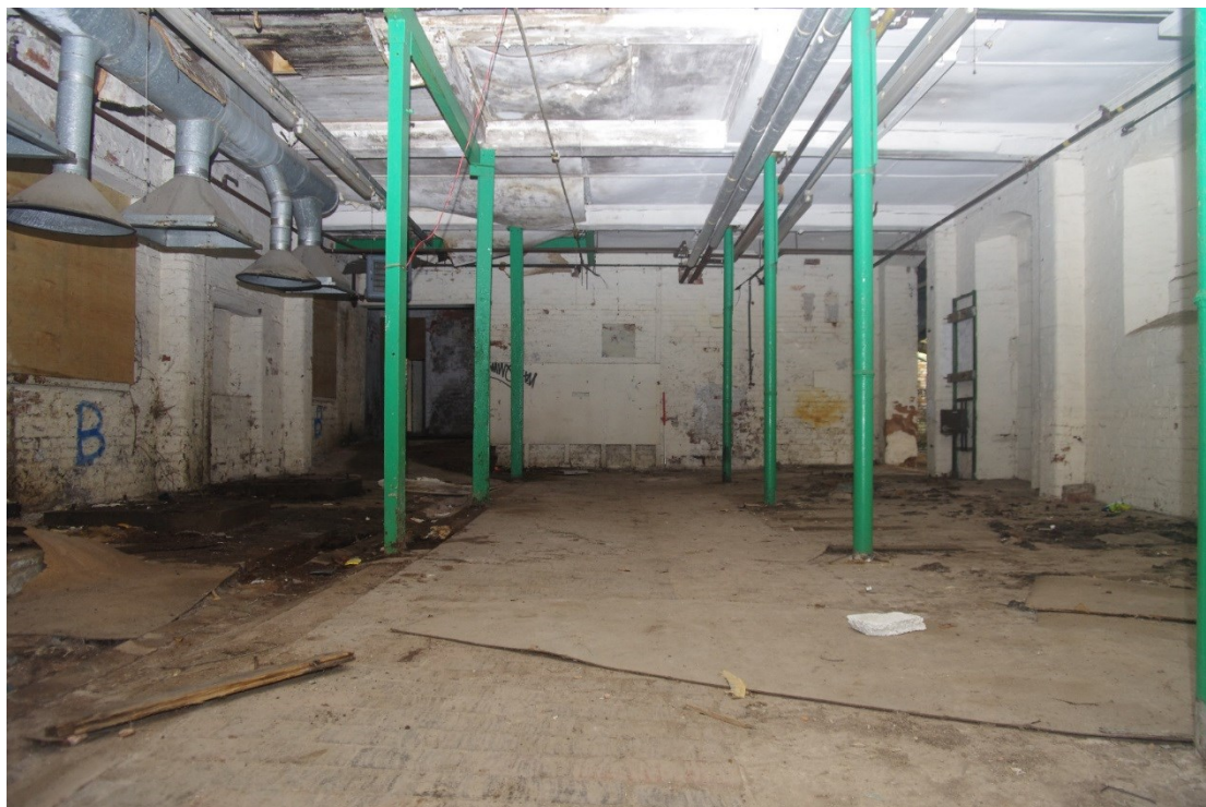
Figure 23 Building C ground floor Looking north-west. 1m scale
