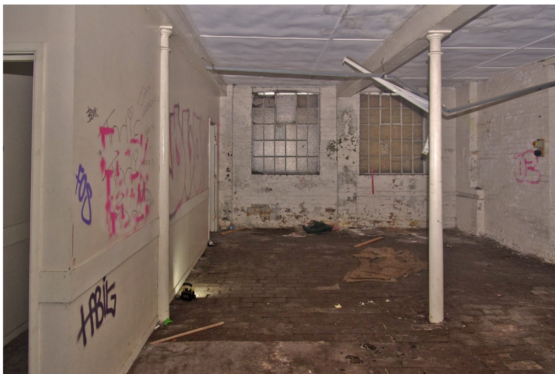
Figure 82 Building U ground floor Looking north-west. 1m scale
