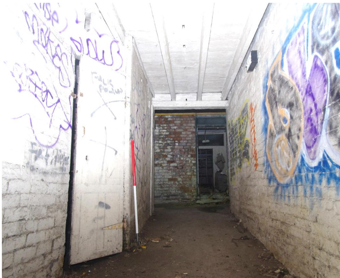
Figure 73 Rear wing R2 ground floor passageway Looking south-west. 1m scale
