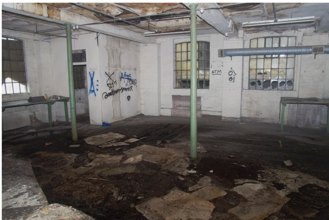
Figure 59 Building Q first floor Looking north from Building R1 doorway
