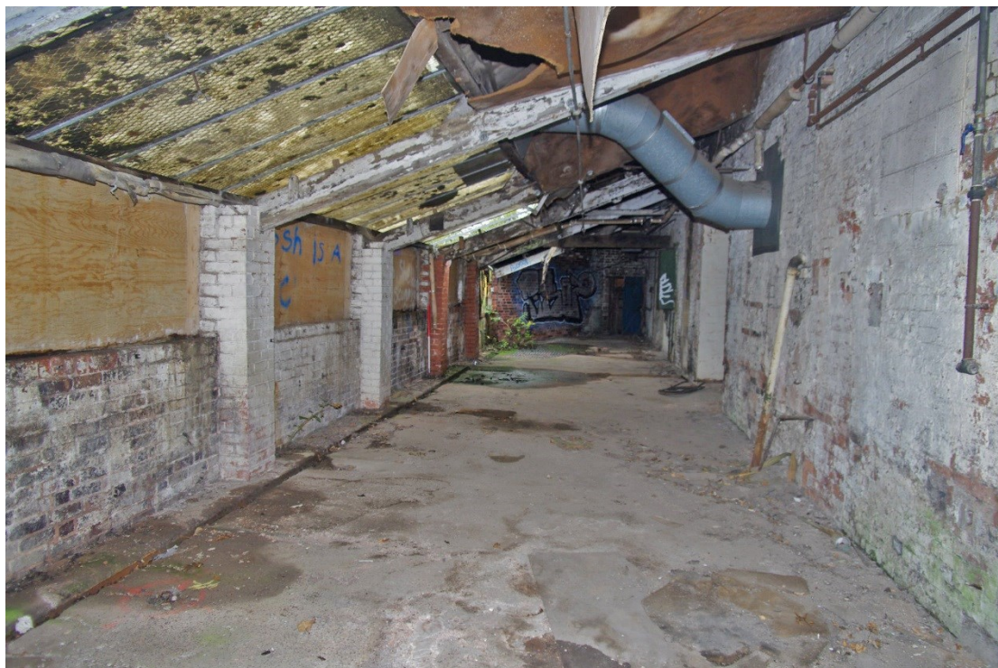
Figure 25 Building D ground floor Looking south-east. 1m scale
