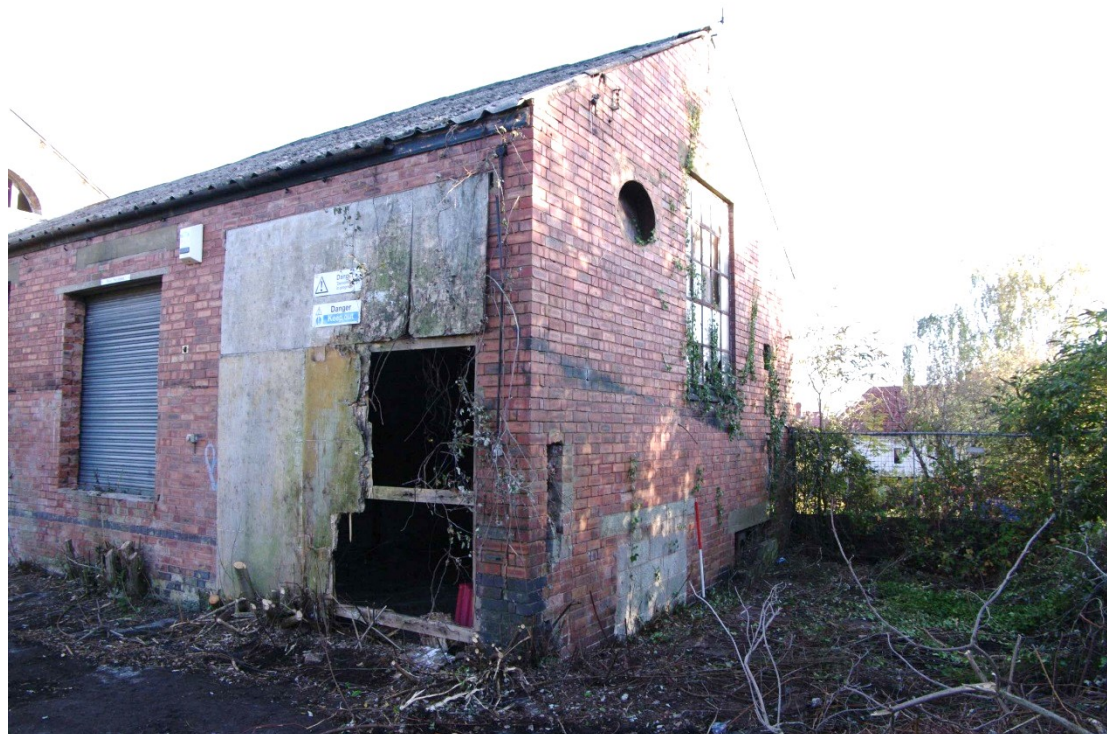
Figure 13 Building A/B south-east facing gable end Looking north. 1m scale
