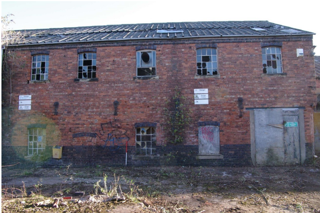
Figure 22 South-west facing elevation of Building C Looking north-east. 1m scale
