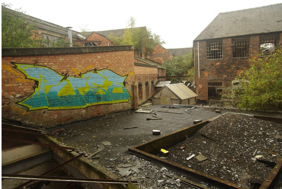
Figure 43 View westwards from first floor of Building F-L Building R2 in centre, Building R1 on right
