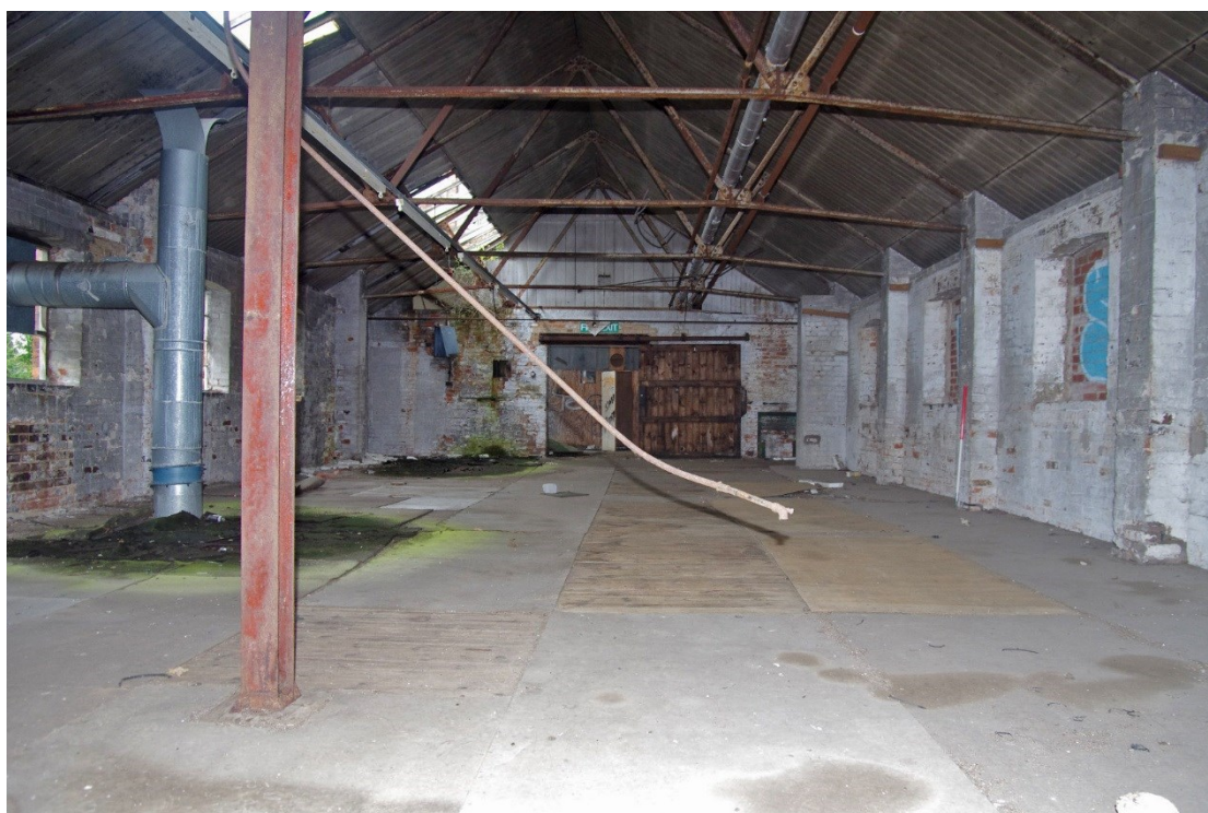
Figure 24 Building C first floor Looking north-west. 1m scale
