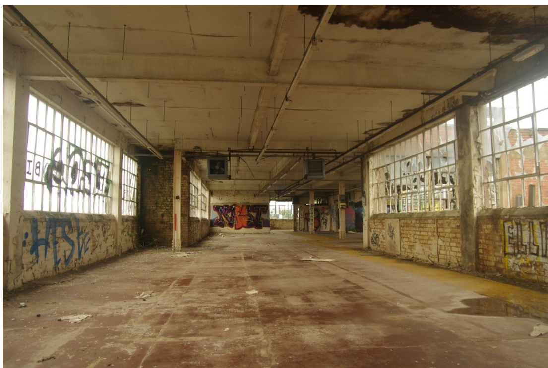
Figure 45 Building F-L second floor Looking south-east. 1m scale
