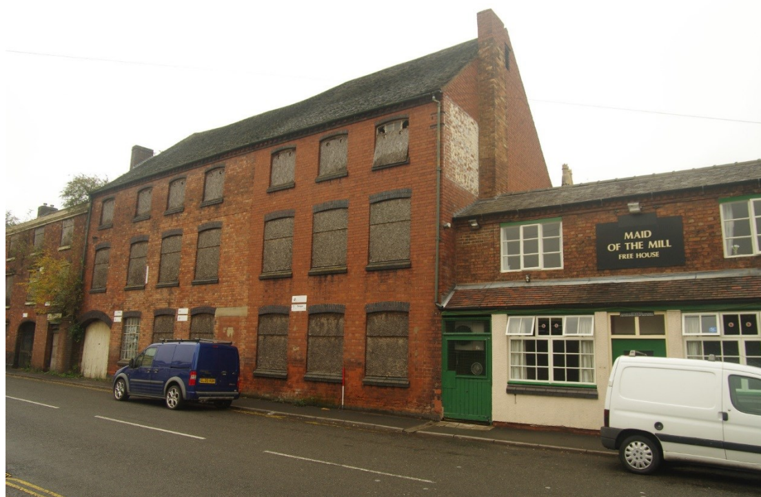
Figure 80 Building U north-west and south-west facing elevations Looking east. 1m scale
