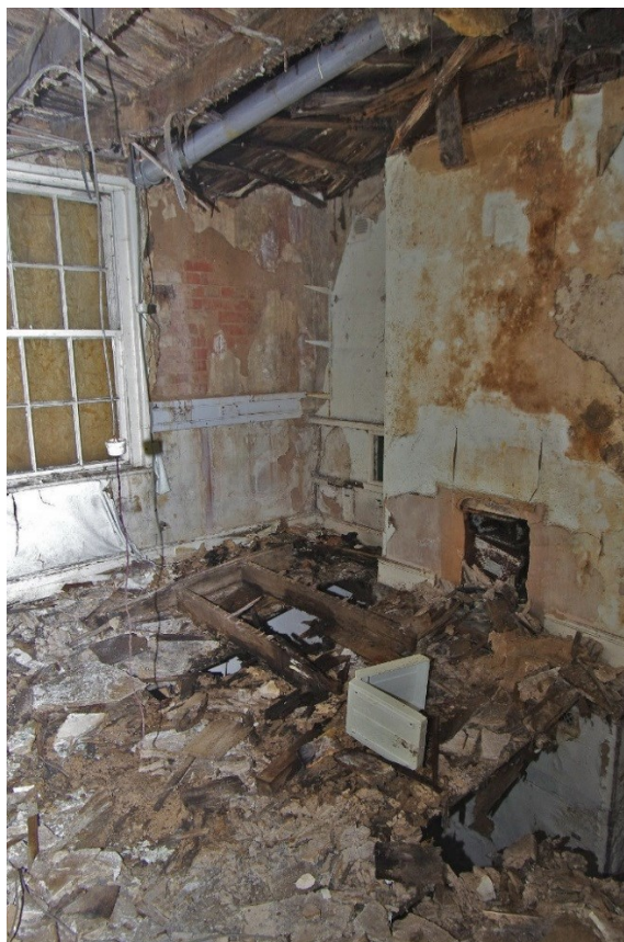
Figure 65 Building R first floor, eastern room Looking north
