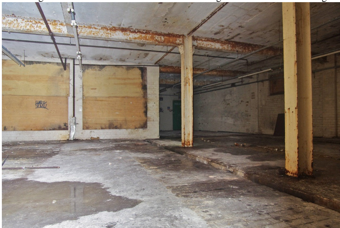
Figure 87 Building V ground floor Looking south
