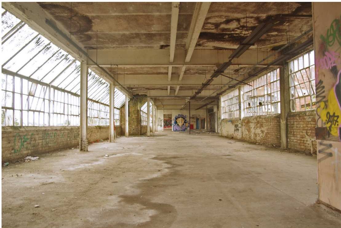
Figure 41 Building F-L first floor Looking south-east. 1m scale
