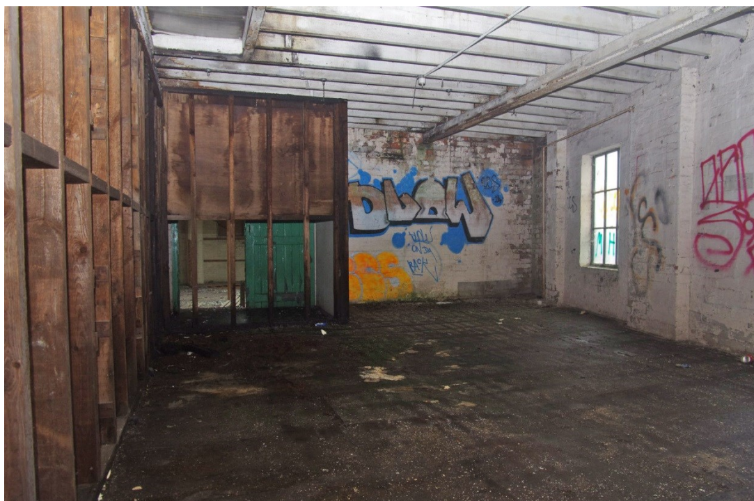
Figure 52 Building N, second floor Looking north from Building F-L
