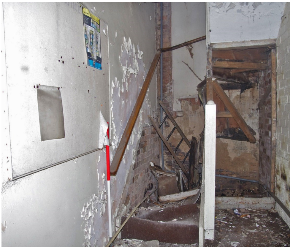
Figure 71 Building R, R2 stairs at ground floor Looking north. 1m scale
