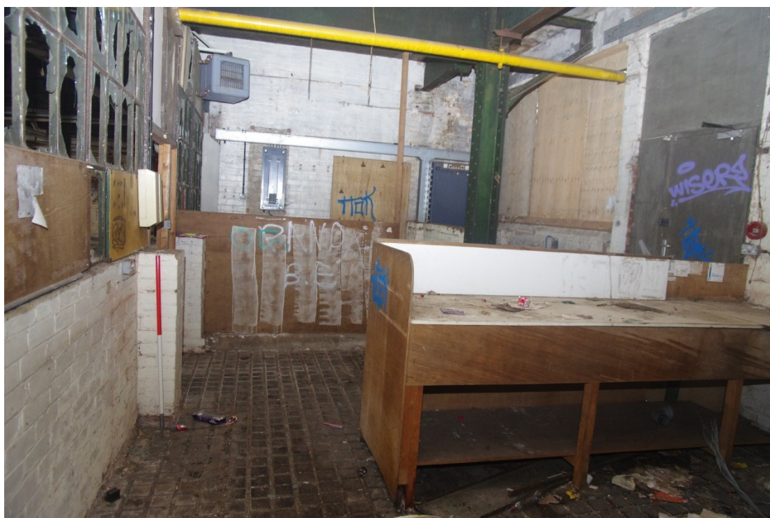
Figure 39 Building F-L ground floor, side rooms Looking west. 1m scale
