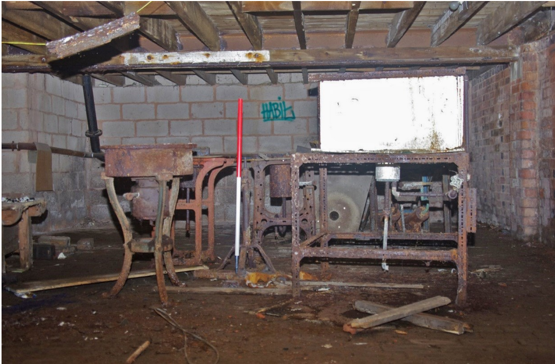
Figure 18 Ground floor of Building A/B Looking south-east. 1m scale
