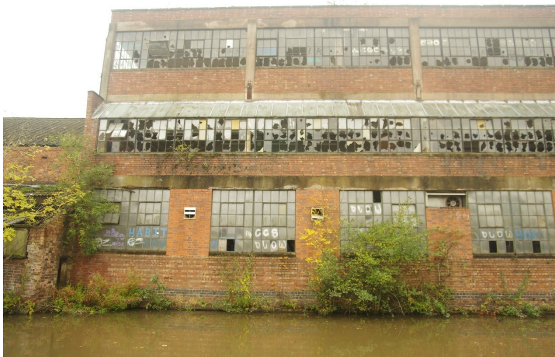
Figure 34 North-east facing elevation of Building F-L (southern end) Looking south-west
