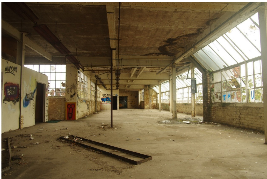
Figure 42 Building F-L first floor Looking north-west
