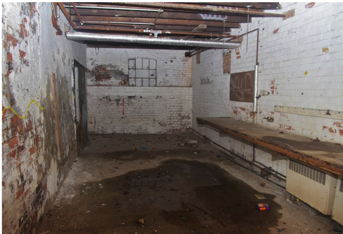
Figure 29 Building E ground floor, middle room Looking north-east. 1m scale
