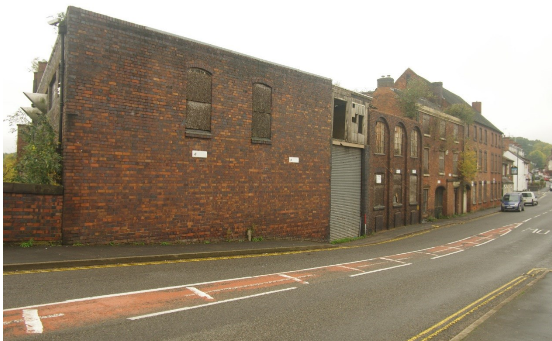
Figure 53 Building O/P Coleshill Road elevation Looking south. Building O/P on left of roller-shutter doors to the vehicle access
