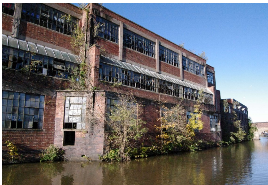
Figure 33 North-east facing elevation of Building F-L (northern end) Looking north-west
