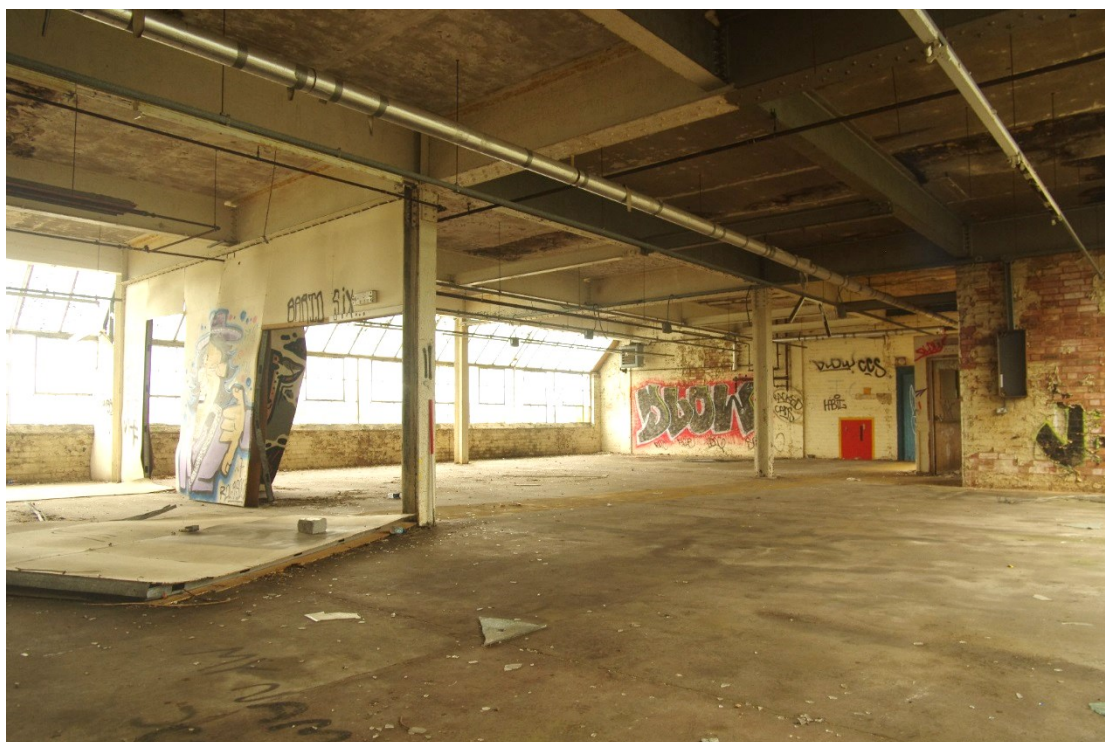
Figure 44 Building F-L first floor, southern end Looking east. 1m scale. Main staircase on far right. Blue door to Building C in centre
