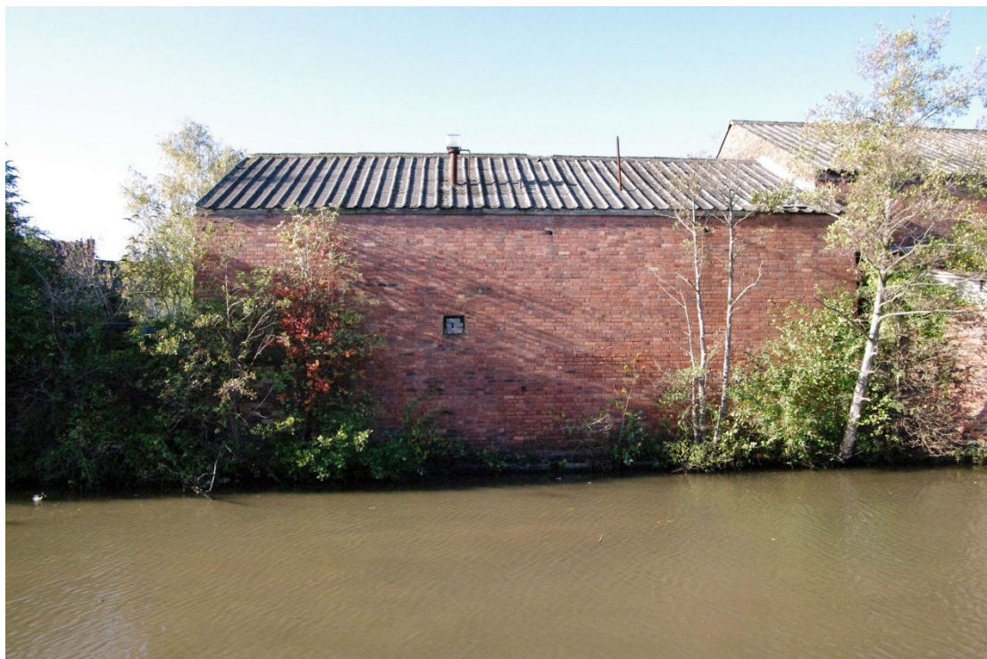
Figure 14 Building A/B north-east facing elevation Looking south-west. Building C/D on right
