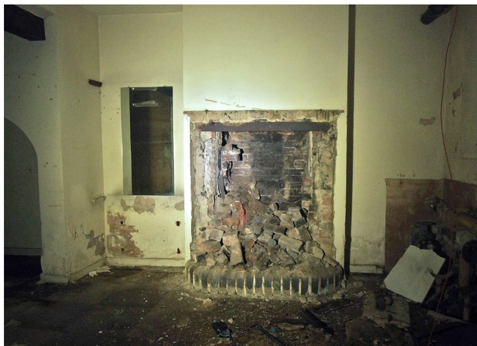
Figure 72 Rear wing R2 ground floor office Looking south-west through window
