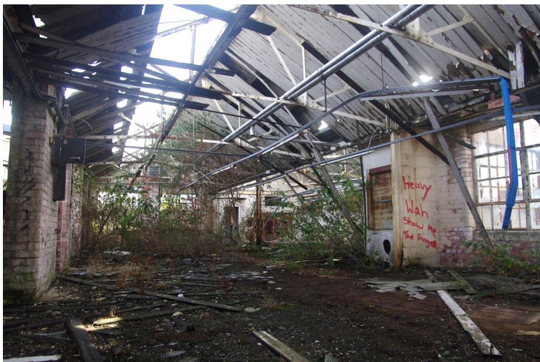
Figure 90 Building V second floor Looking north-west from southern staircase
