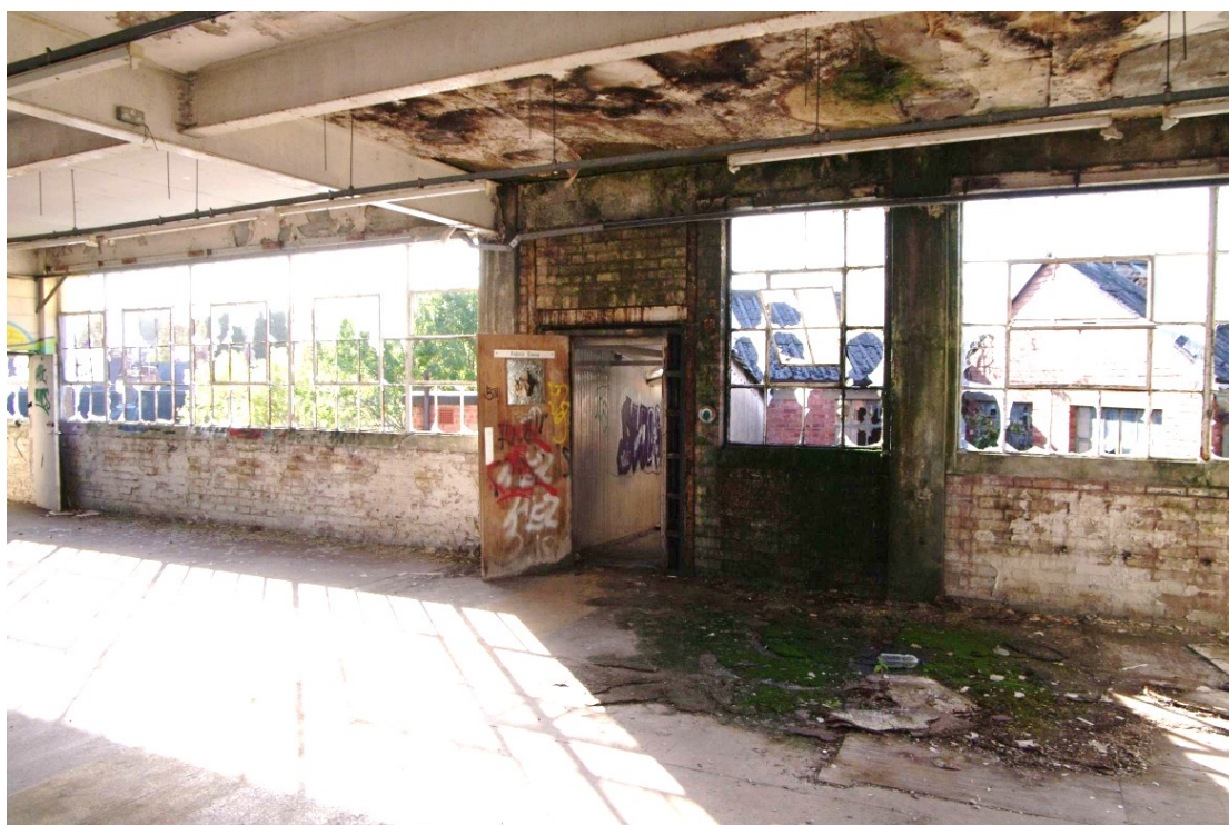
Figure 47 Bridge from second floor of Building F-L to Building V Looking south-west
