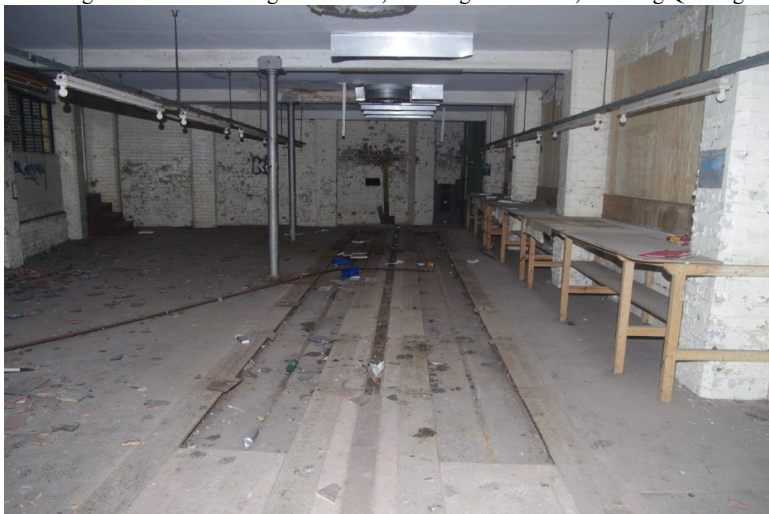
Figure 56 Building O/P ground floor Looking north-west towards Coleshill Road wall
