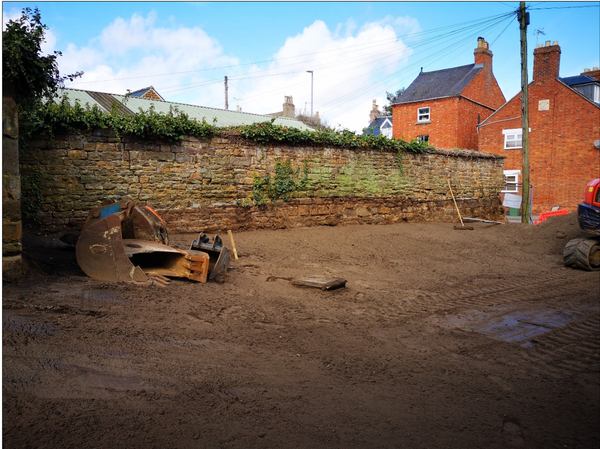
Figure 25: Internal garden area after completion of groundworks, topsoil reinstated, looking north-west.
