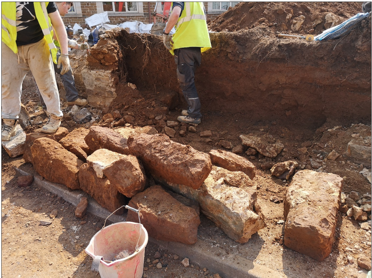
Figure 22: Footings being removed, looking south.
