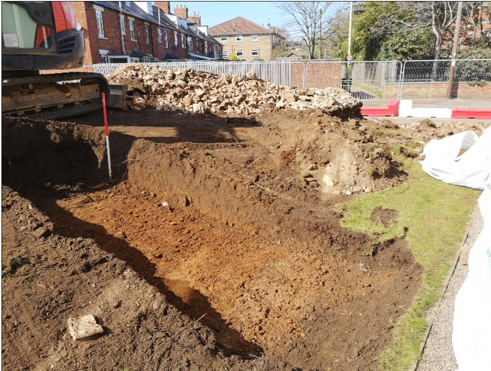
Figure 8: Trench 2 looking north
