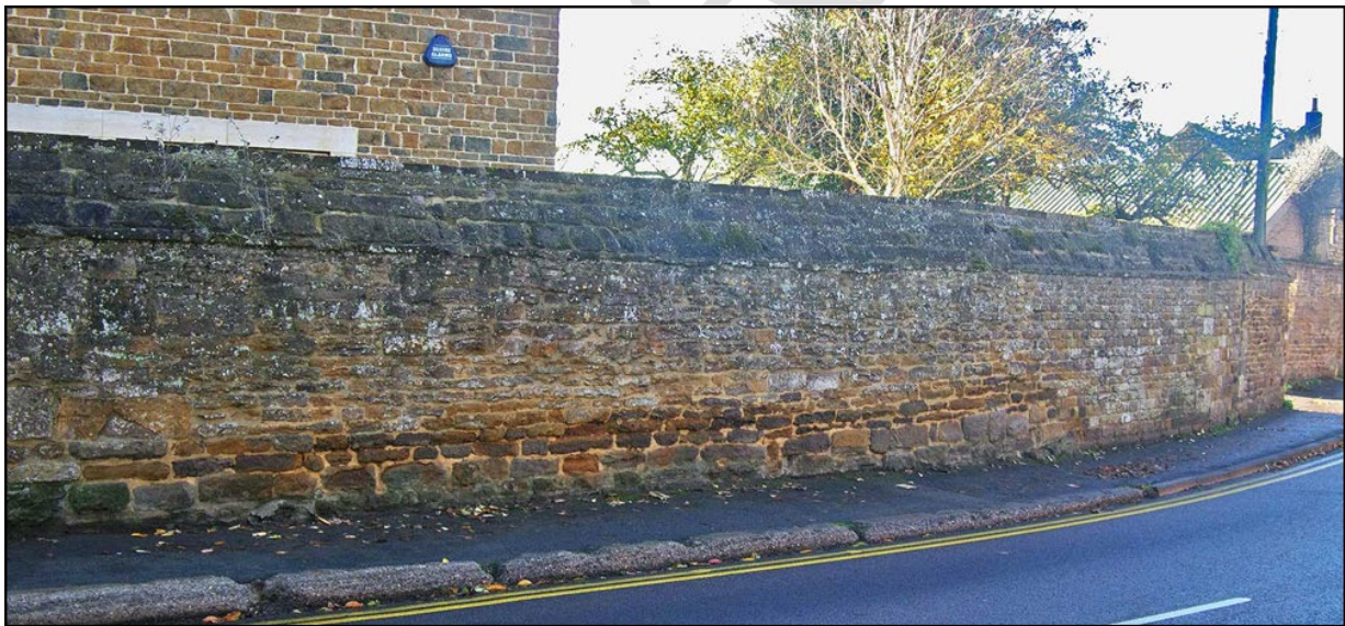
Figure 4: Wall subject to rebuilding prior to current works (Coward 2019).
