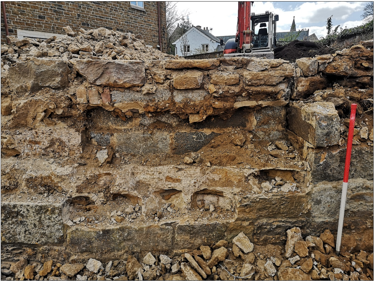
Figure 20: Wall (1) looking south, showing modern infilling.
