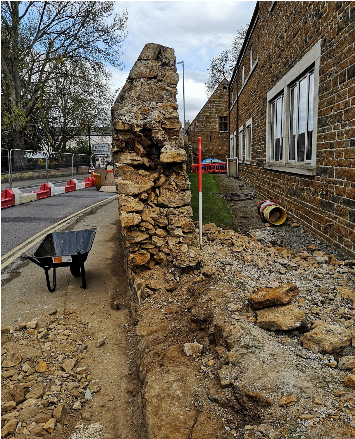
Figure 19: Wall (1) looking east, showing rubble core, mortared upper level, footings.
