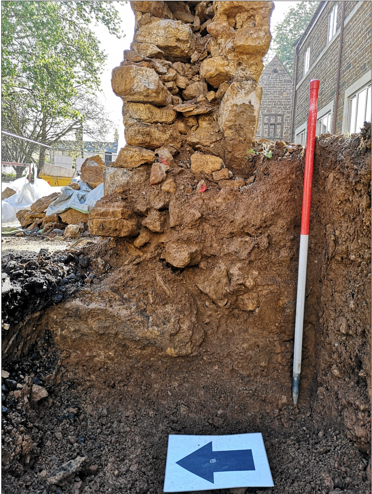
Figure 23: Wall (1) showing wider external footing (left), and lack of internal footing (right).
