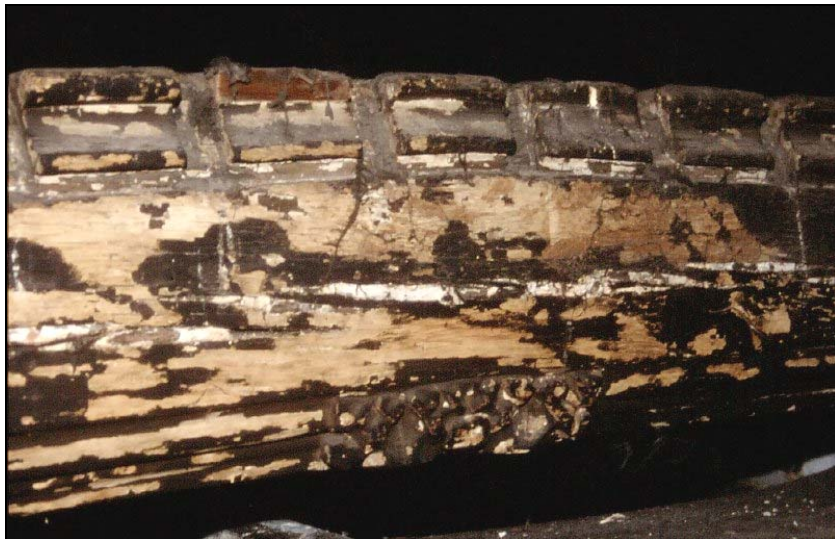
Figure 10. Detail of reused roof timber with crenellated moulding and boss fragment.
