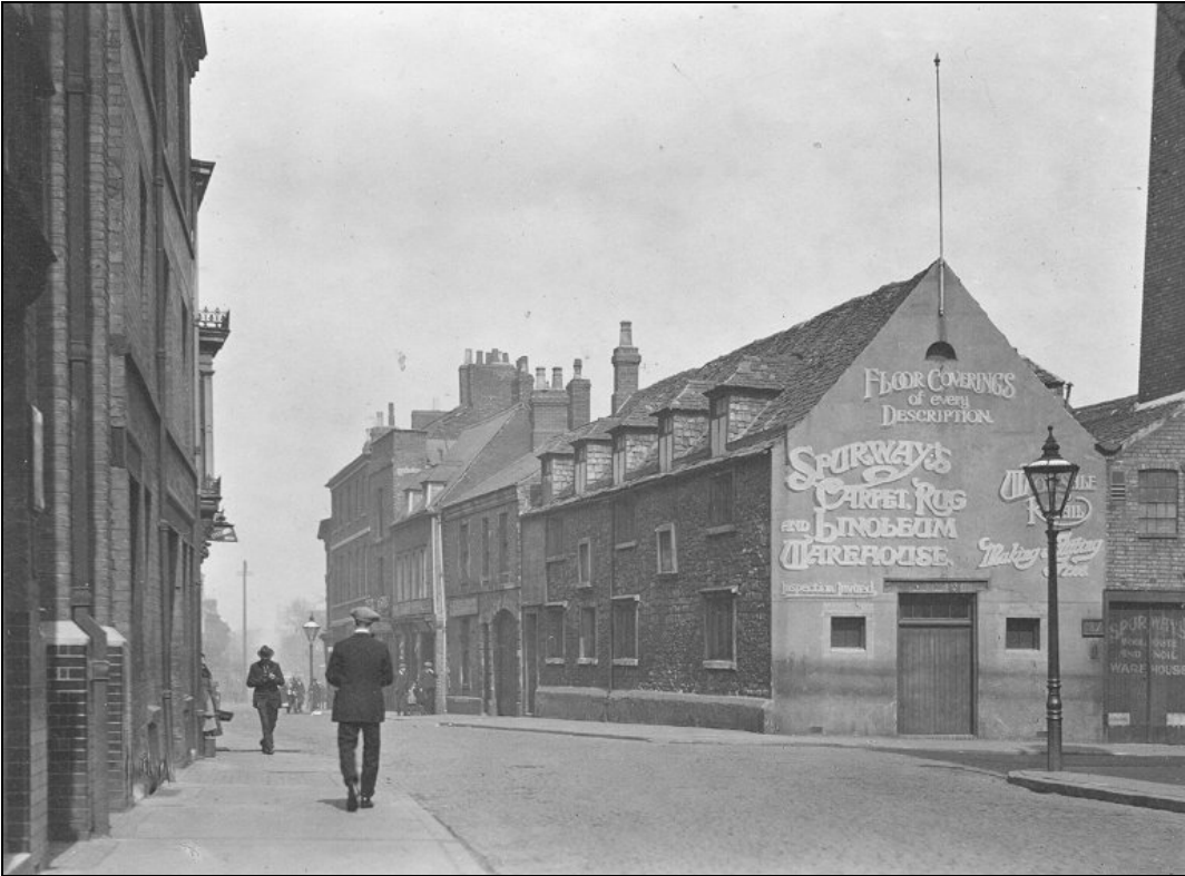
Figure 31. Photograph c.early 20th century Highcross Street elev. (DE3736 Box 17 Folder 6).
