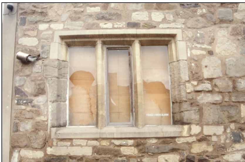
Figure 11. Window on rear (east) elevation with fragments of early stone jambs.
