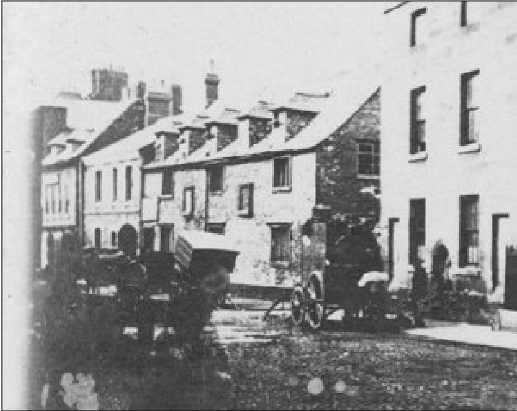
Figure 30. Photograph c.1880s Borough Gaol, Highcross Street (DE3736 Box 17 Folder 5).
