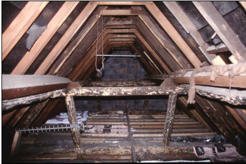
Figure 9. Free Grammar School roof structure.
