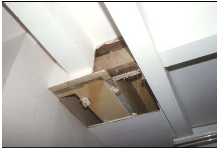
Plate 5. Area F opening to investigate first floor structure
