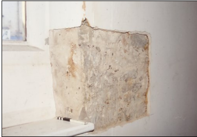
Plate 17. Area 8 opening to investigate internal wall coverings
