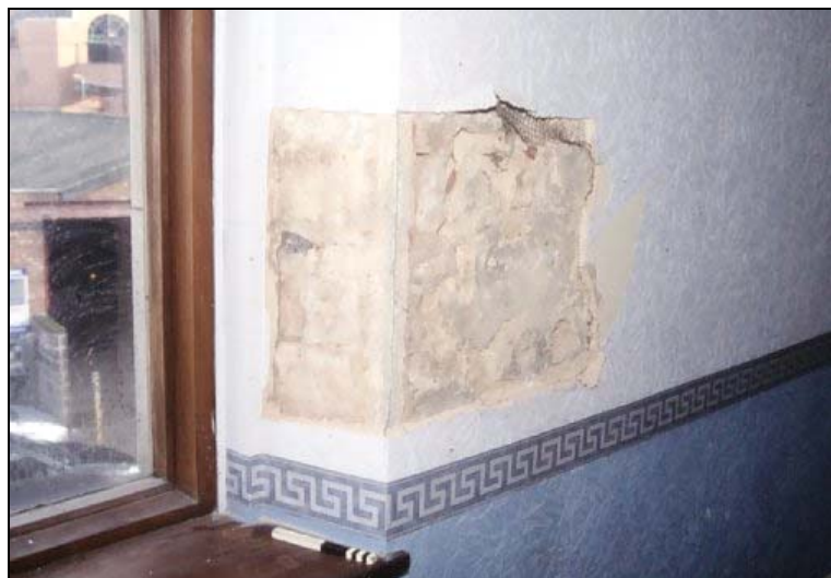
Plate 20. Area 11 opening to investigate internal wall coverings/window W14
