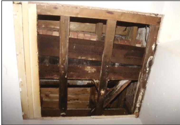
Plate 3. Area C opening to investigate first floor structure
