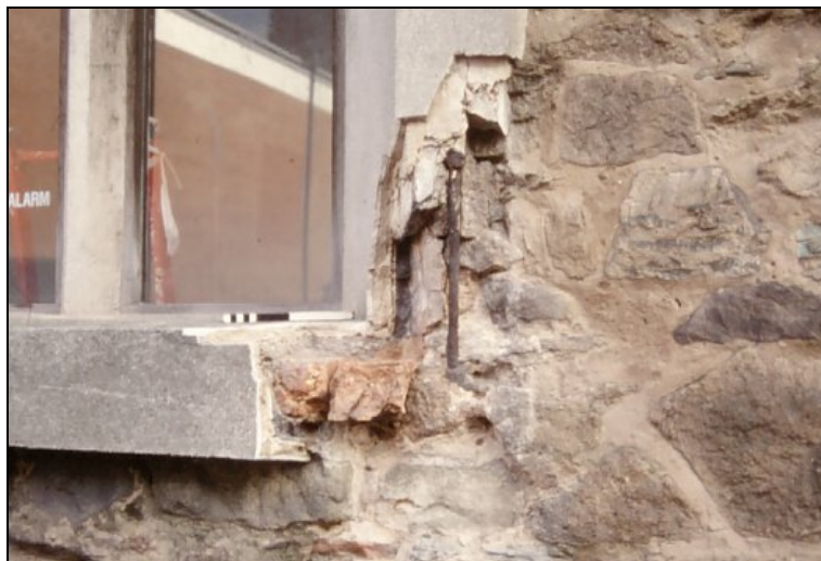
Plate 10. Area 3 opening to investigate surround of window W5
