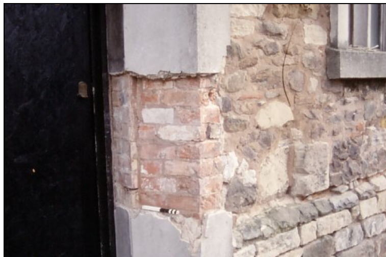
Plate 8. Area 1 opening to investigate surround of door D1
