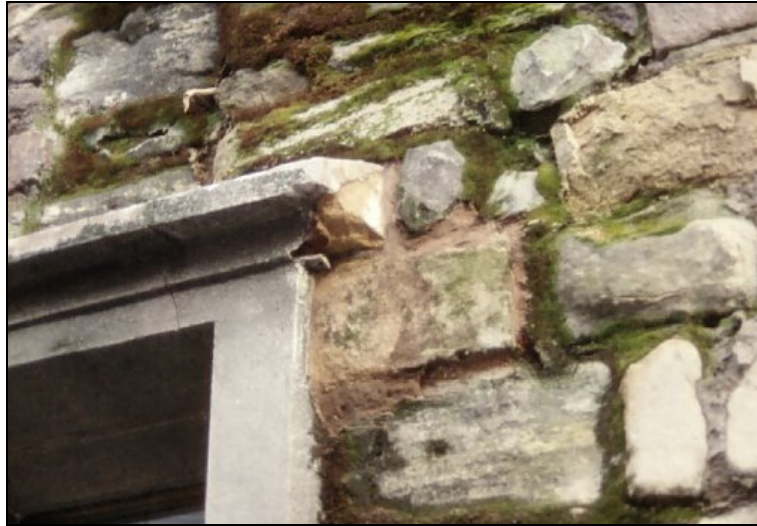
Plate 15. Area 6 opening to investigate hoodmould of window W1
