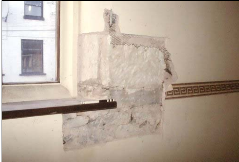
Plate 19. Area 10 opening to investigate internal wall coverings
