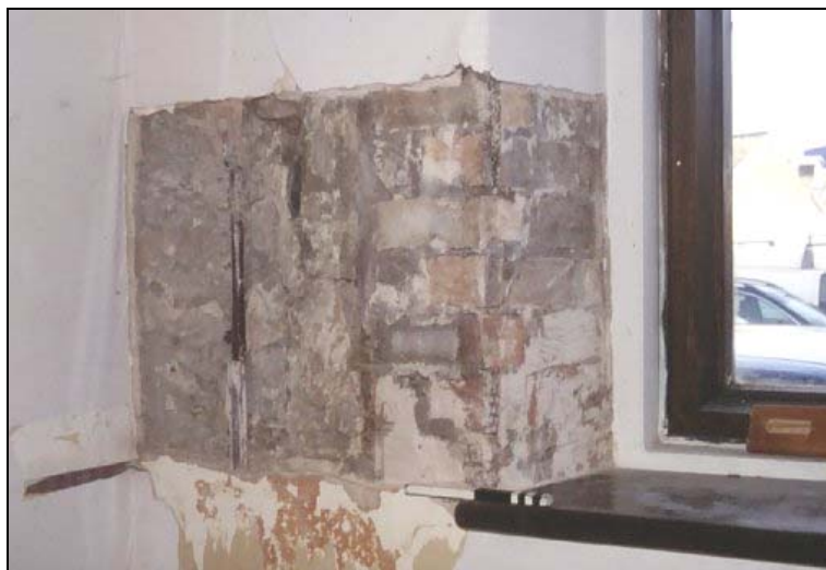
Plate 18. Area 9 opening to investigate internal wall coverings/window W6
