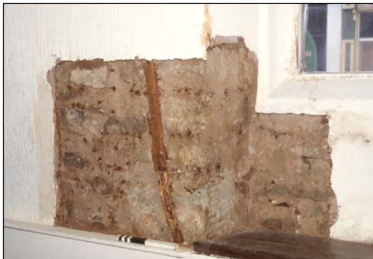
Plate 16. Area 7 opening to investigate internal wall coverings
