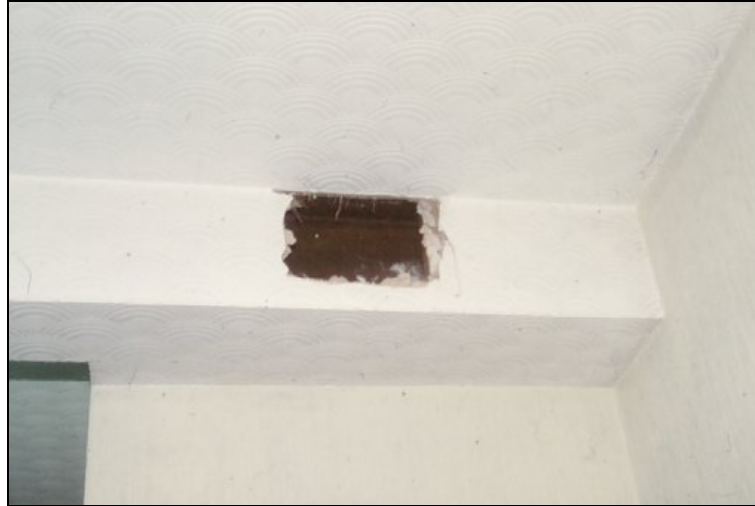
Plate 1. Area A opening to investigate first floor structure
