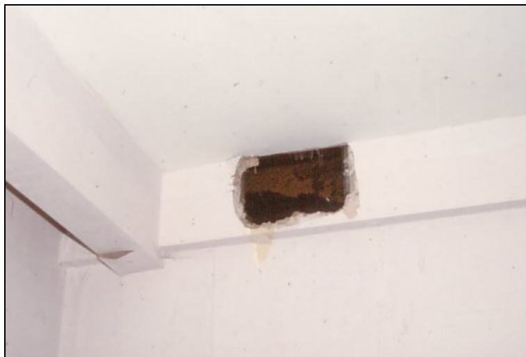
Plate 6. Area G opening to investigate first floor structure
