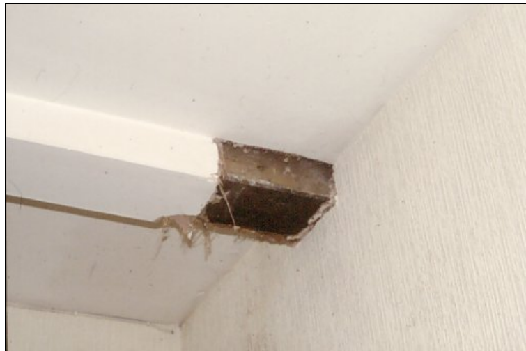
Plate 2. Area B opening to investigate first floor structure
