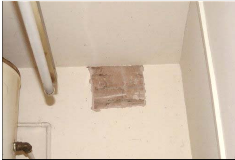
Plate 7. Area H opening to investigate first floor structure
