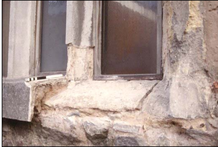
Plate 9. Area 2 opening to investigate surround of window W7
