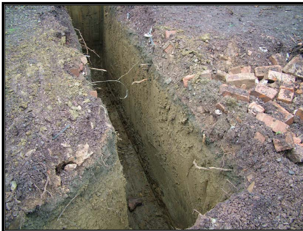
Figure 6 Foundation trench, illustrating depth and narrowness.
