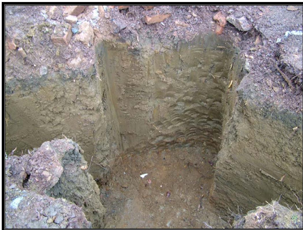
Figure 5 Foundation trench illustrating the thickness of alluvium and natural substrata.
