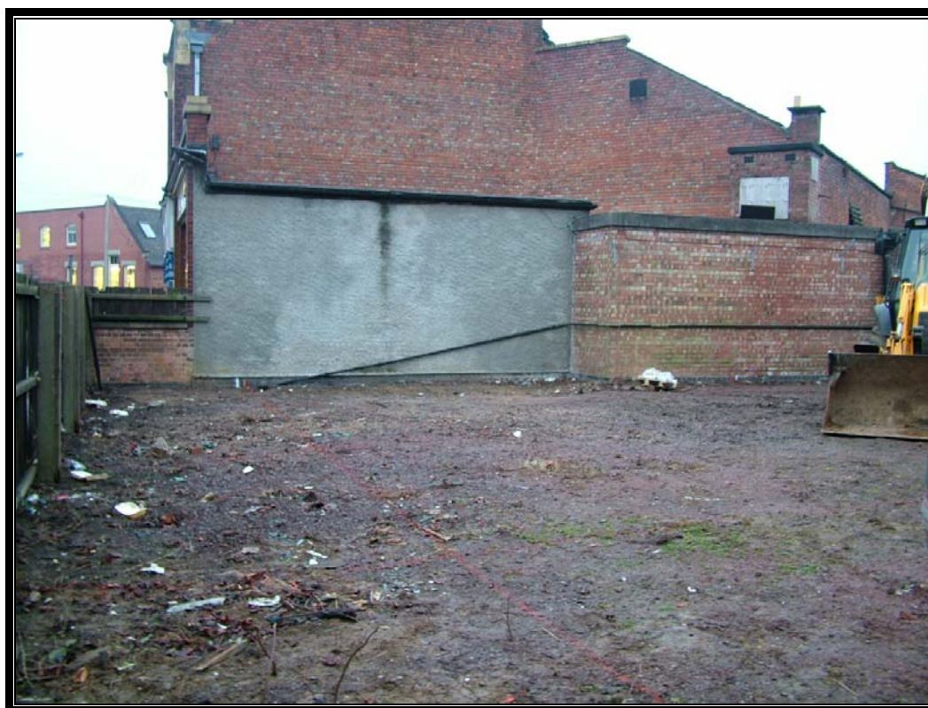
Figure 4 Site, pre-machining, looking south.
