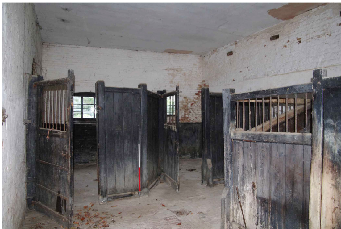
Figure 40 The Coach House ground floor west wing Looking north-west. 1m scale
