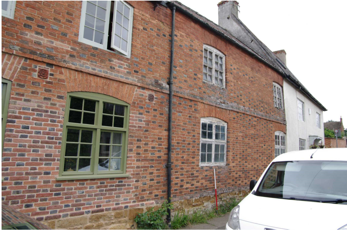
Figure 8 Saddle House south facing elevation Looking north-east. 1m scale. The wall of Saddle House appears to be continuous with Number 8 on left
