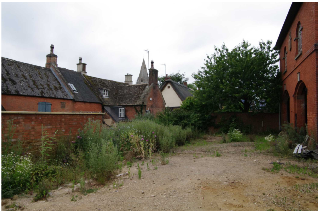
Figure 5 Saddle House and the Coach House Looking west. Saddle house on the left with the blue hayloft doors. Coach House on the right
