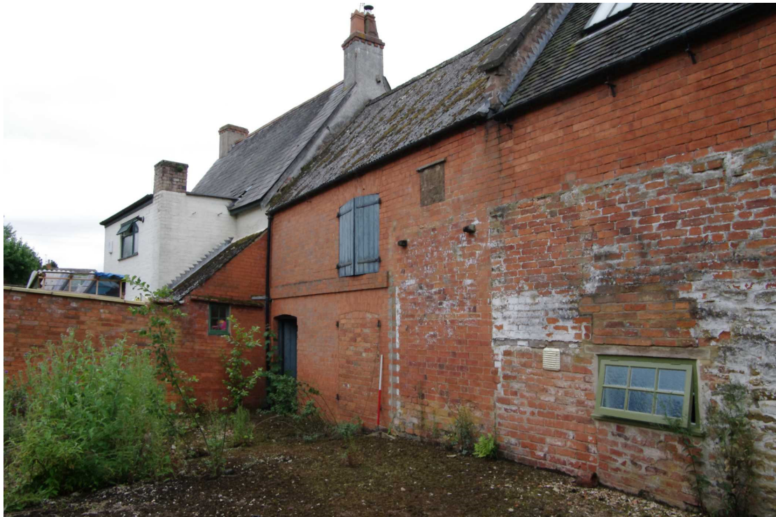
Figure 12 Saddle House north facing elevation Looking south-east. 1m scale
