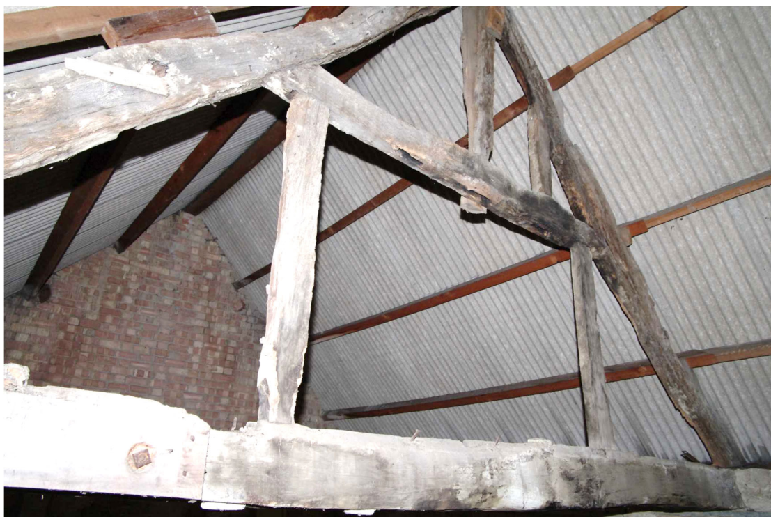
Figure 27 Detail of saddle House roof structure Looking north-west
