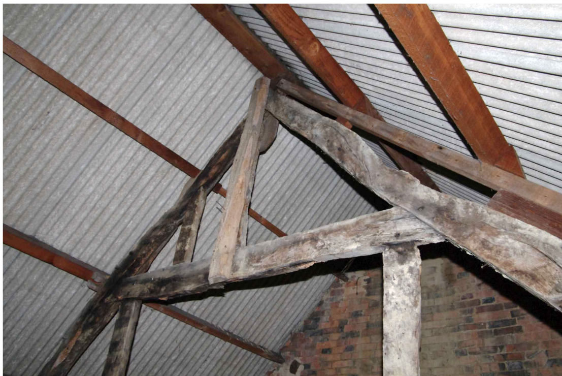
Figure 26 Detail of saddle House roof structure Looking north-east
