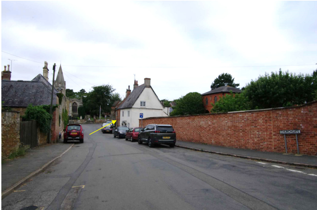
Figure 4 Saddle House and Coach House location Looking west along Churchgate. Saddle House shown by yellow arrow. The Coach House is behind bushes on the right
