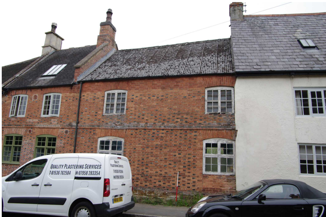
Figure 7 Saddle House south facing elevation onto Churchgate Looking north. 1m scale. Note stone base of wall and raised eaves. The blocked doorway which is now a window is on the right behind the black car's bonnet
