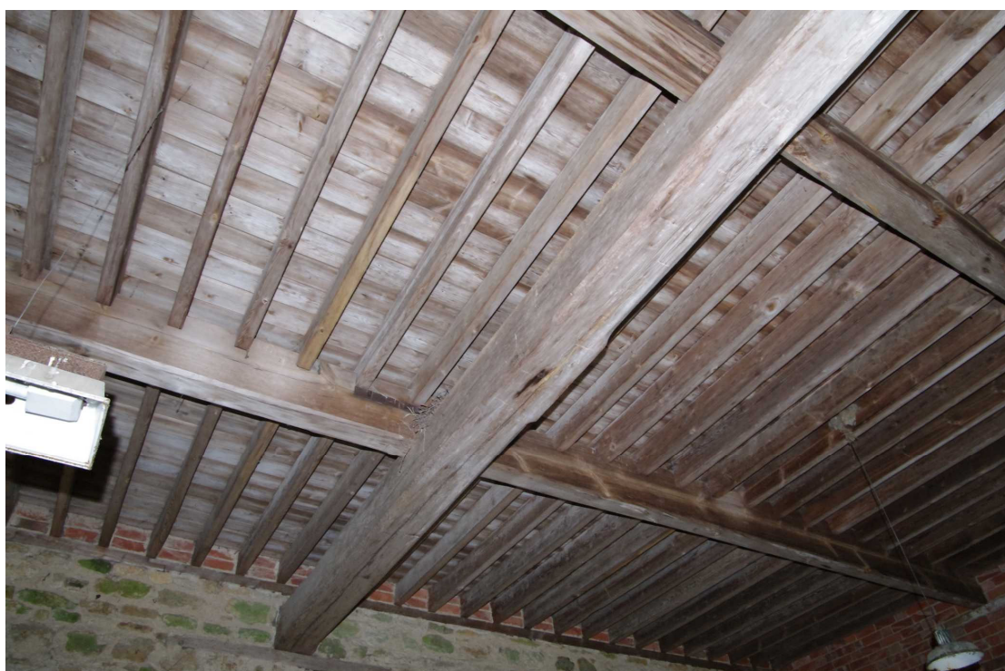
Figure 48 The Coach House ground floor middle range North to south stop-chamfered beam
