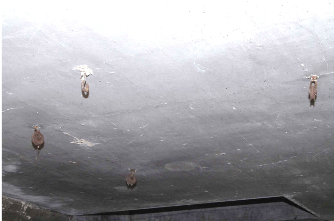
Figure 20 Saddle House ground floor eastern room ceiling Looking north-west. Hooks and pulleys of unknown function
