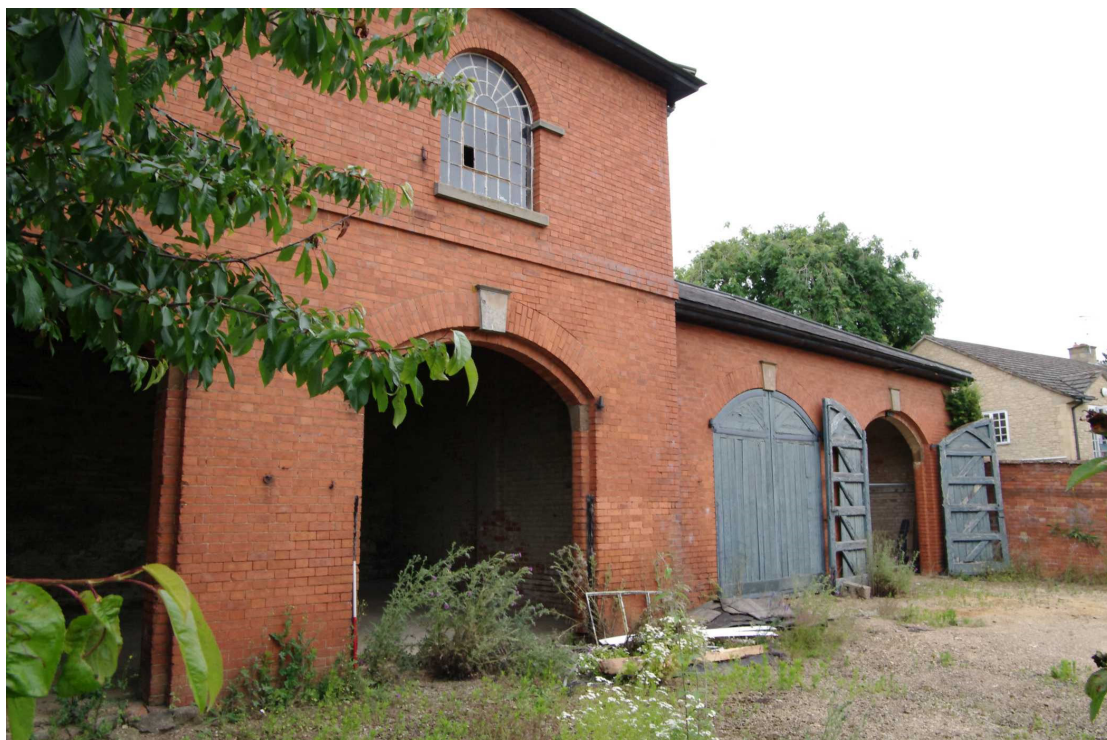
Figure 31 The Coach House south facing elevation Looking north-east. 1m scale
