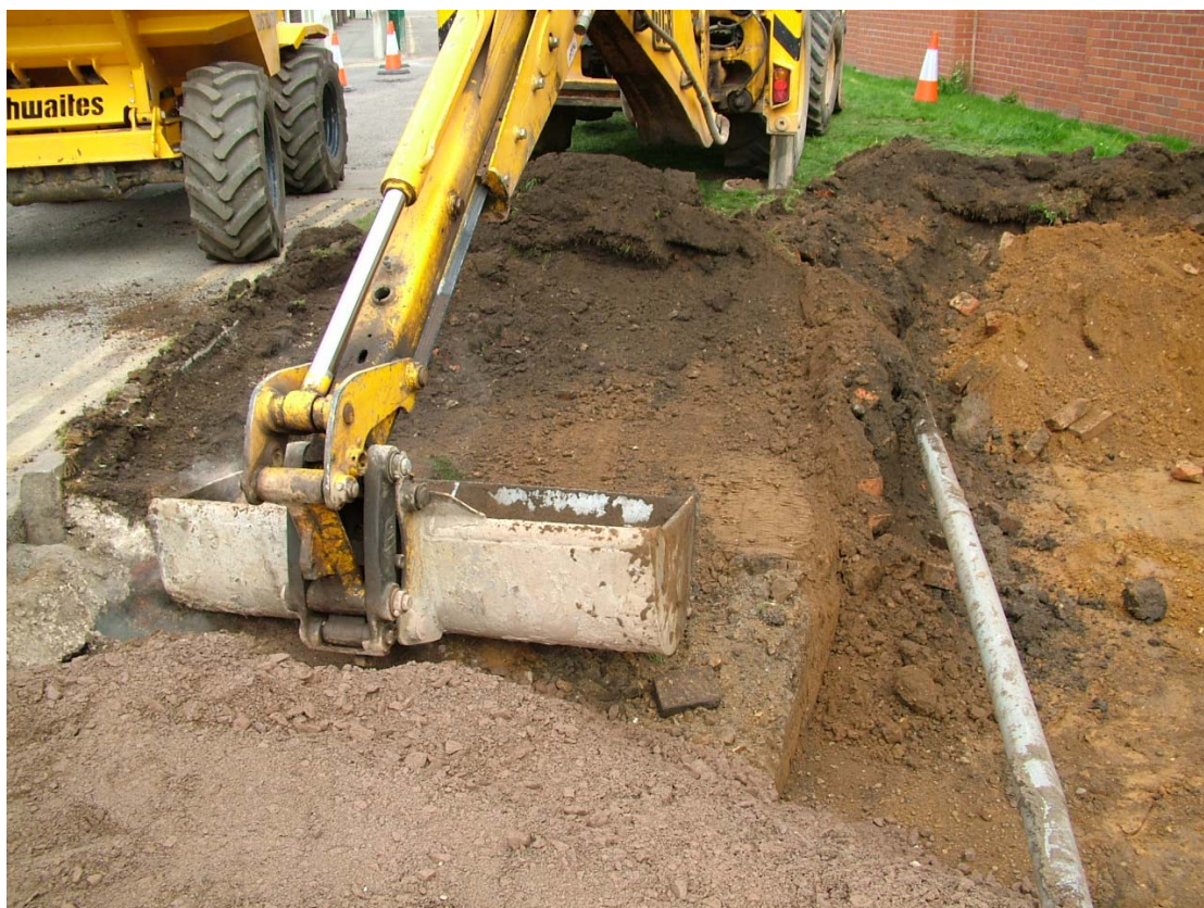
Fig 5 Ground reduction in progress in the area of the car park
