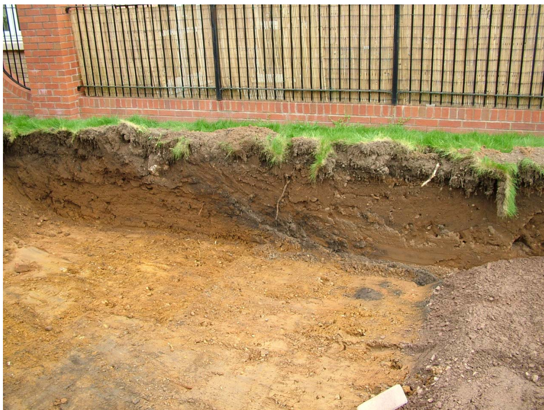
Fig. 6 Car park ground reduction. Natural substratum below subsoil and topsoil visible in section
