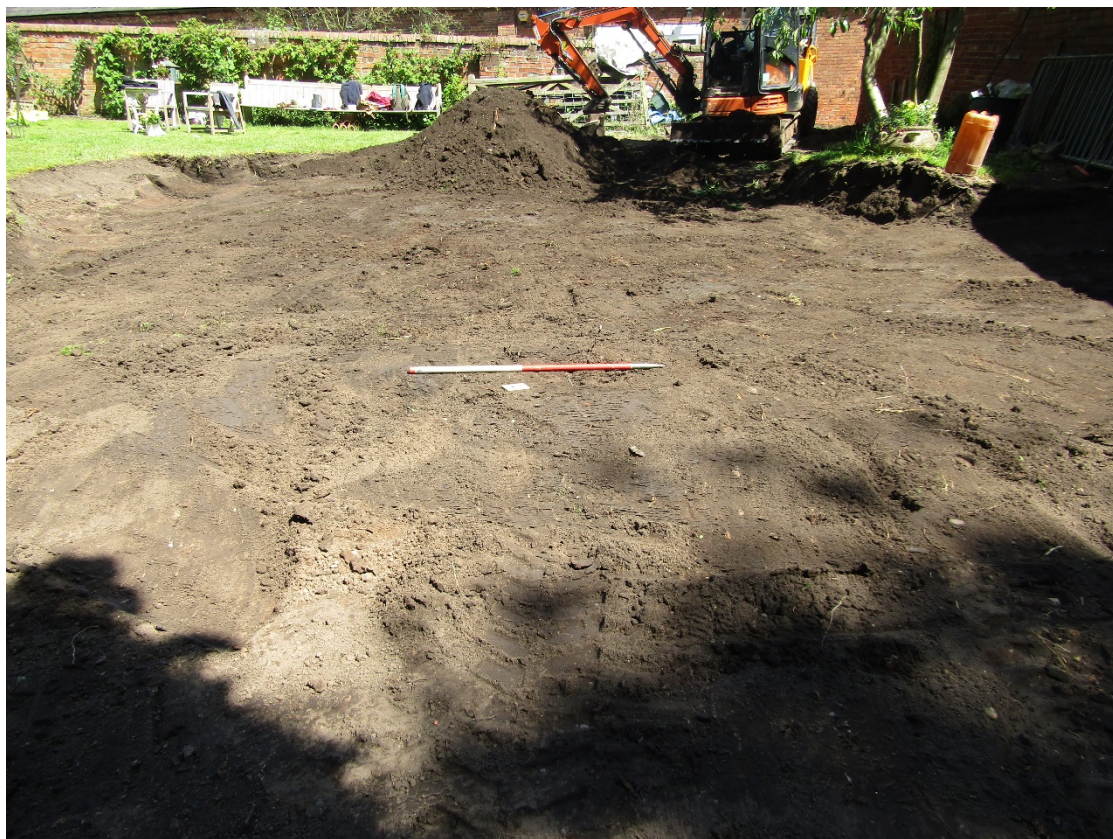
Figure 9: Development site looking east
