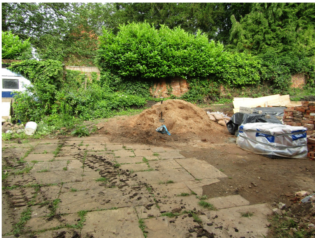
Figure 6: Area of hardstanding to the west of the workshop looking west.
