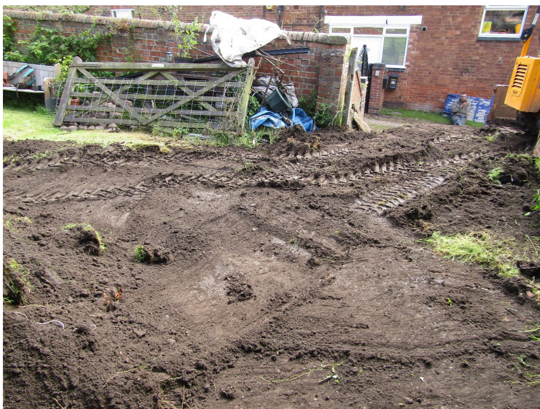
Figure 11: Development site looking east, towards the proposed (and current) access.
