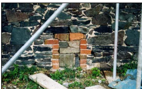
Plate 59. Blocked feature on south wall of building eight.
