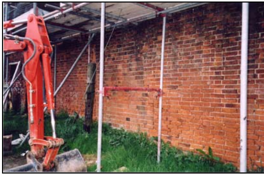
Plate 2. Patch of rebuilt brickwork on the centre of the west elevation.
