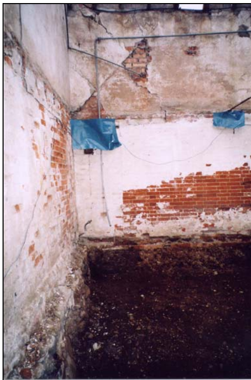
Plate 26. Northeast corner showing top of moat wall with joist sockets above.
