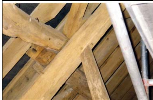
Plate 53. Southern aspect of principle truss on the east wall. Plate 54. Close up view of 53 above illustrating example of carpenter's marks.
