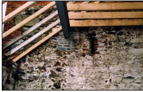
Plate 49. Southeast corner of barn showing rubble walling. Plate 50. South wall of barn showing rubble construction.
