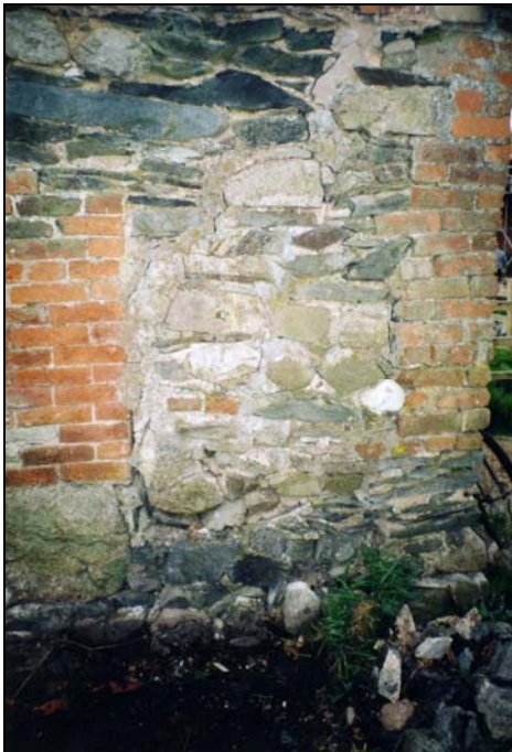
Plate 32. Detail of north elevation showing blocked door. Plate 33. West elevation of building four.
