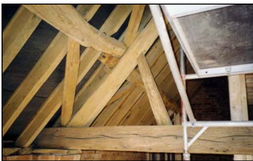
Plate 53. Southern aspect of principle truss on the east wall. Plate 54. Close up view of 53 above illustrating example of carpenter's marks.
