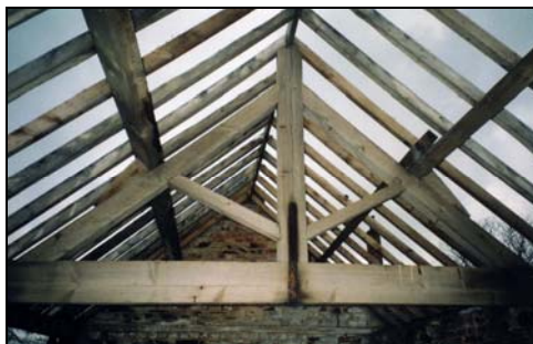
Plate 35. General arrangement of the roof structure, building four.
