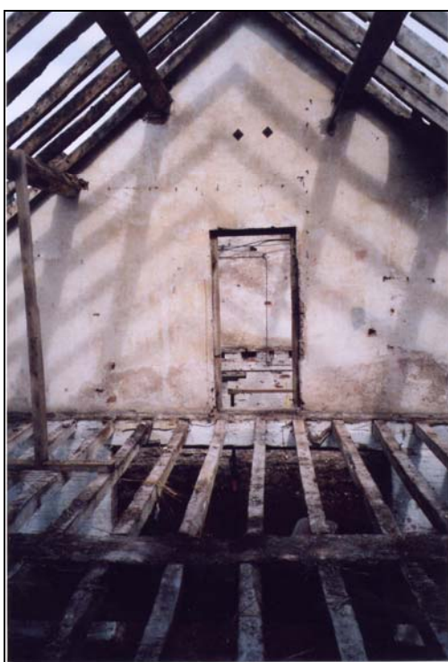
Plate 27. First floor level showing arrangement of floor joists.
