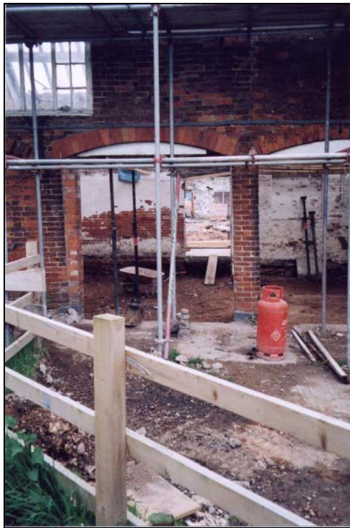
Plate 22. The centre left bay arched opening showing rebuilt soldier.
