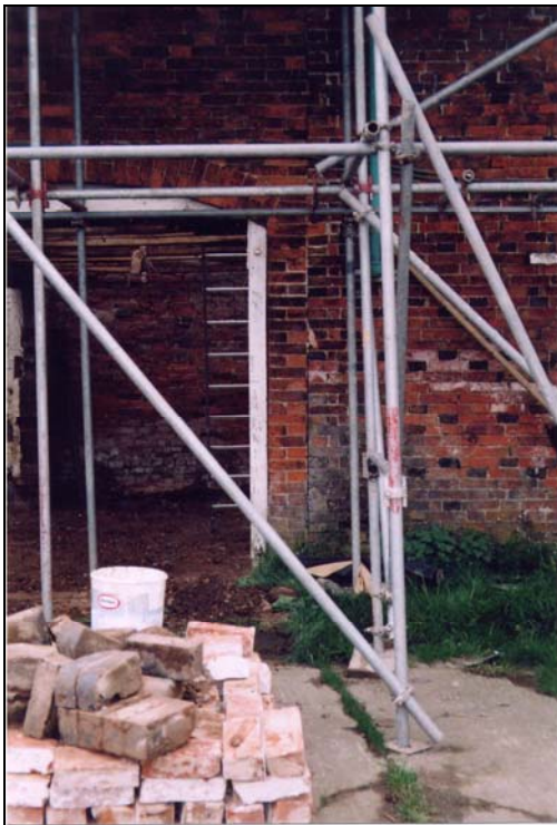
Plate 23. Southwest corner butt joint to north wall of Pigeon house.
