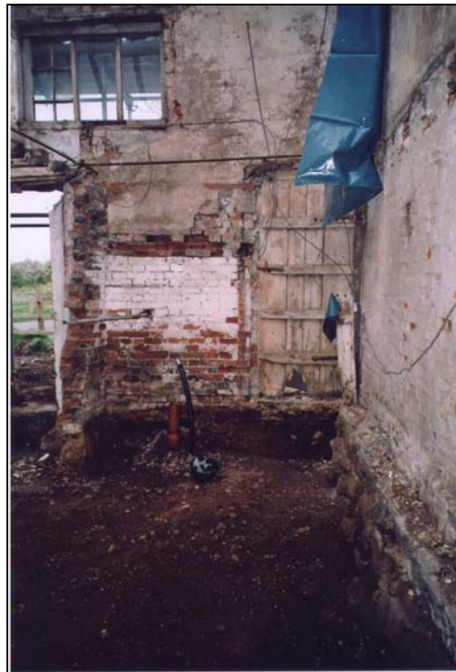
Plate 23. Southwest corner butt joint to north wall of Pigeon house.
