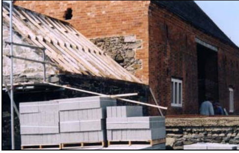
Plate 49. Southeast corner of barn showing rubble walling. Plate 50. South wall of barn showing rubble construction.
