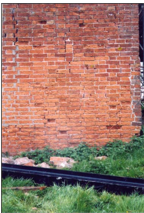
Plate 7. Blocked former vent opening on the south wall.
