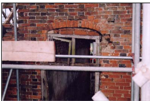
Plate 11. The segmented arch above the east elevation door. Plate 12. East elevation of building three showing former milking shed outline.
