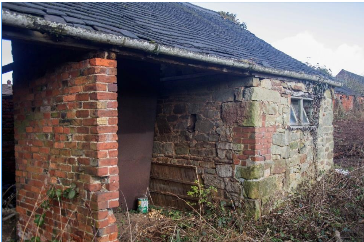
Figure 33 Block F, looking north-east
