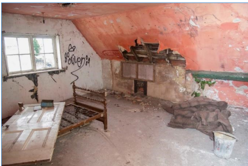
Figure 61 Second floor south east bedroom, looking south east
