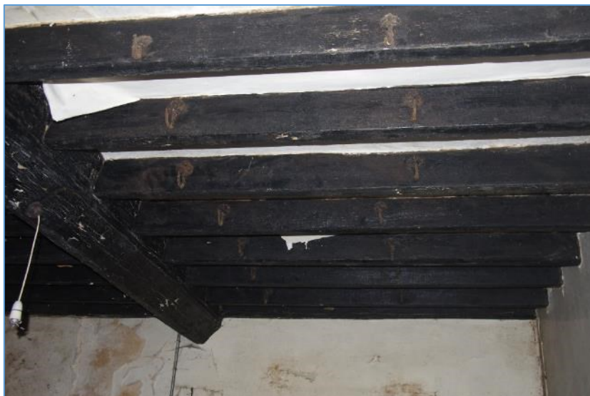
Figure 46 Joists with meat hooks
