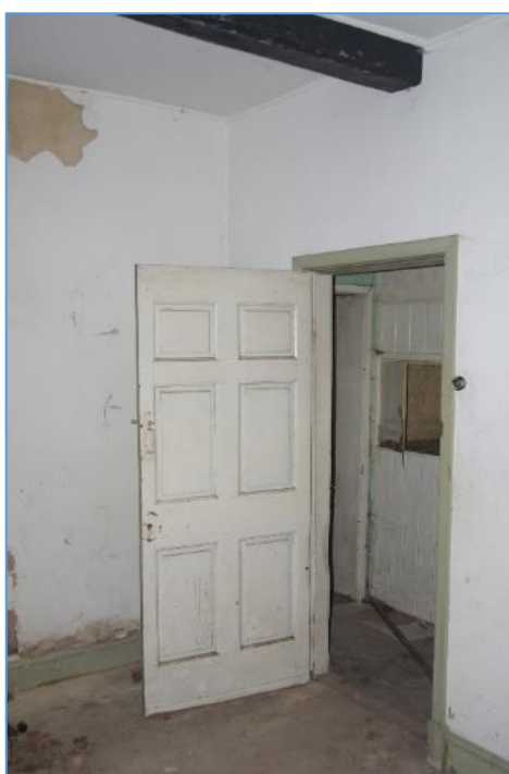
Figure 49 Dining room, looking across corridor to serving hatch
