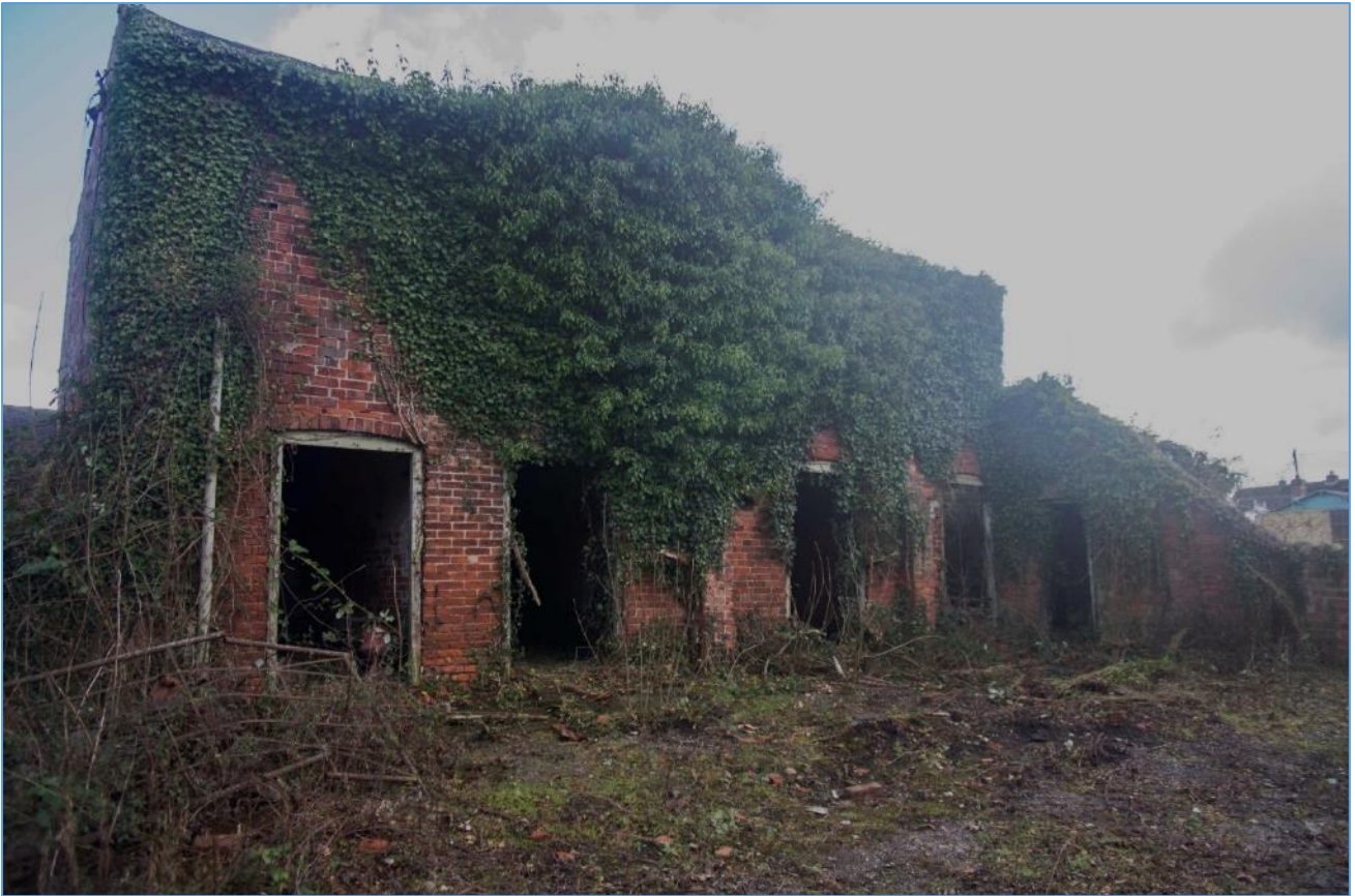
Figure 28 Block E looking east
