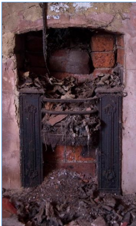
Figure 62 Detail of Pantheon hob grate
