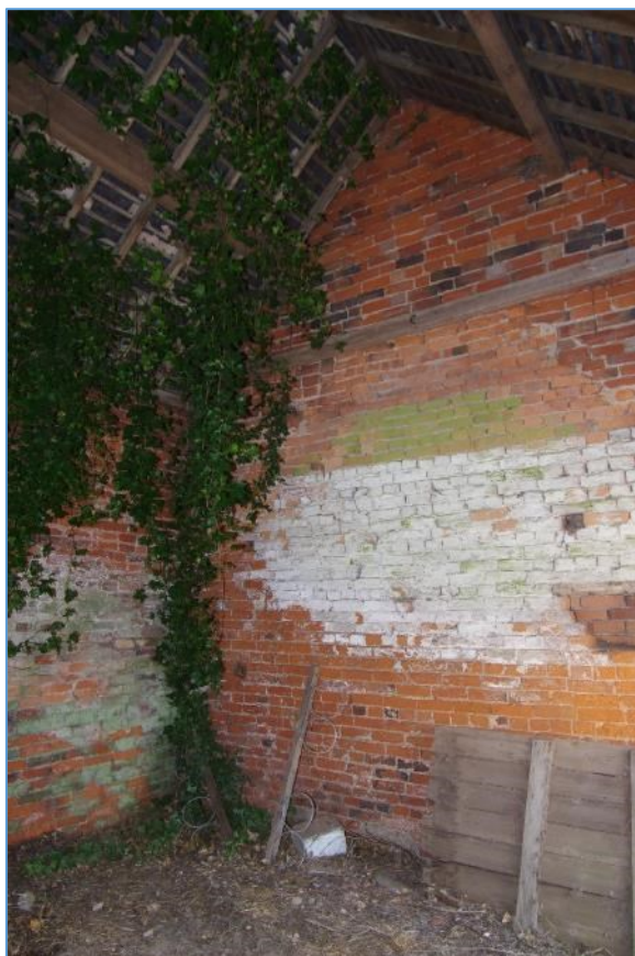
Figure 21 Block C, north unit, looking south east.
