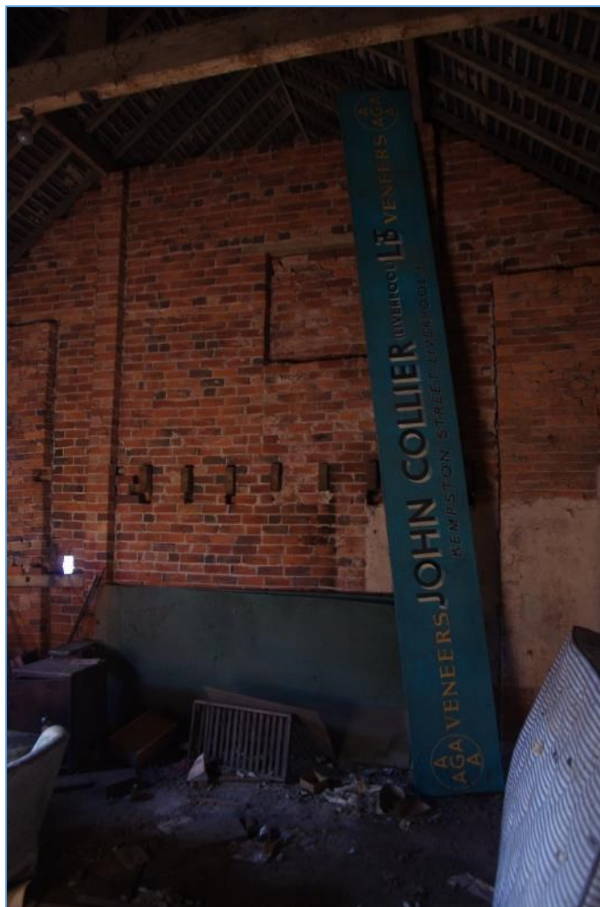
Figure 14 Block A east side. Looking west
