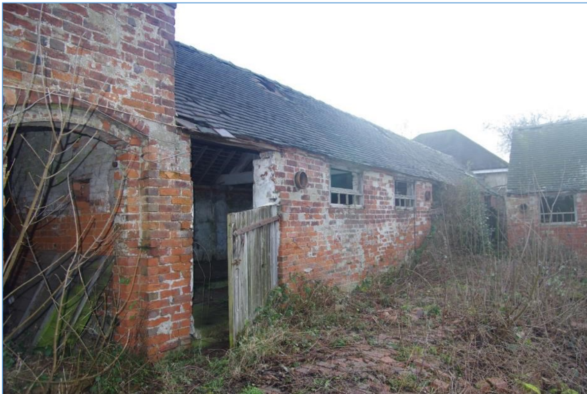
Figure 20 Block C west elevation looking south-east
