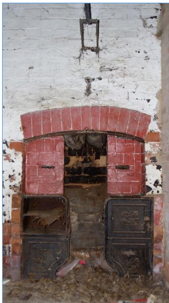
Figure 52 Open range on north wall
