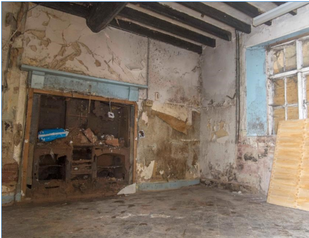
Figure 45 Kitchen, looking north east
