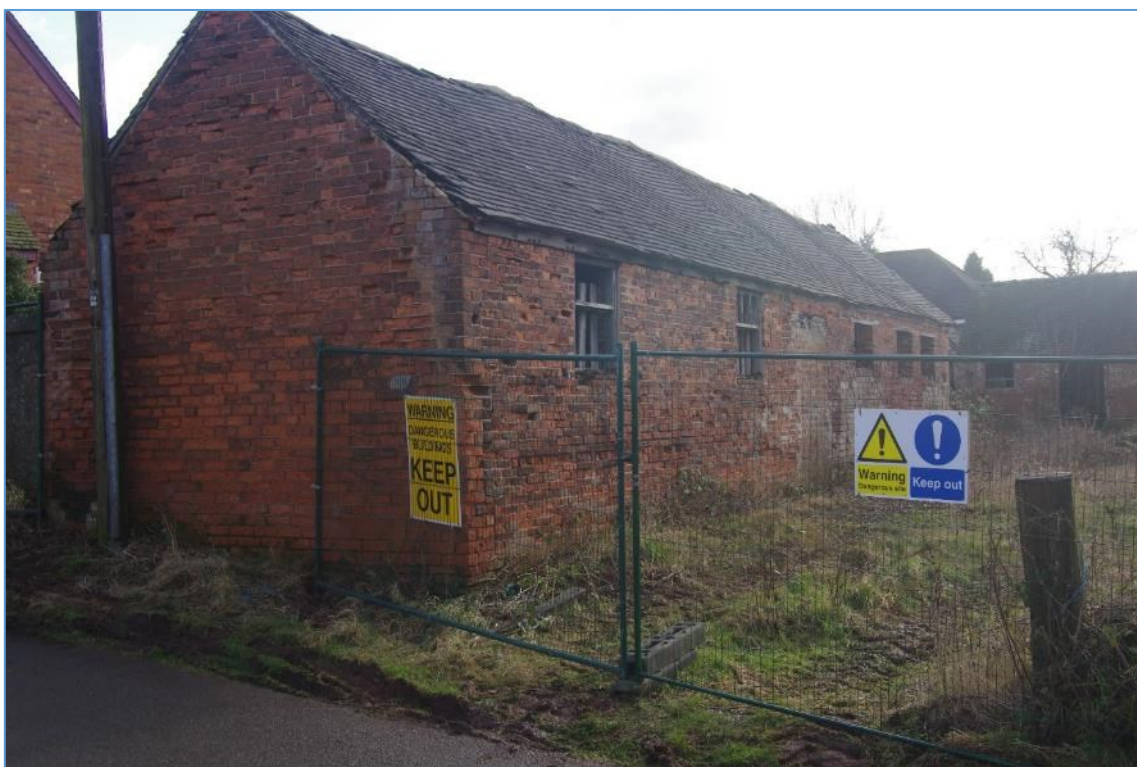
Figure 16 Block B looking south-east. Note rebuilt gable end
