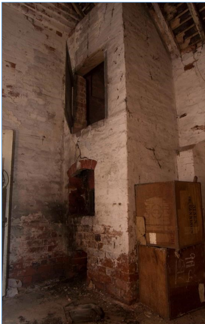
Figure 50 Oven in bakehouse/scullery. Looking south west
