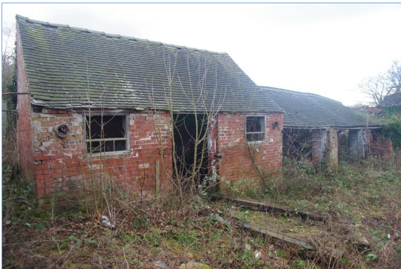
Figure 24 Block D looking south west
