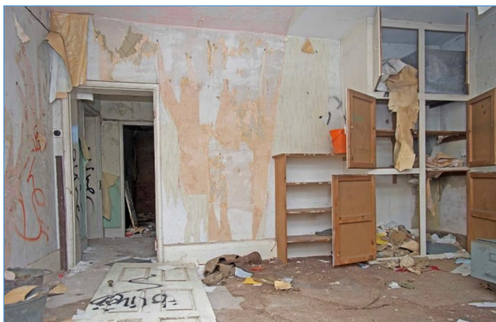
Figure 59 North east bedroom, looking west
