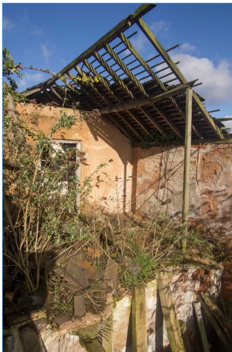
Figure 31 Block E upper storey looking north
