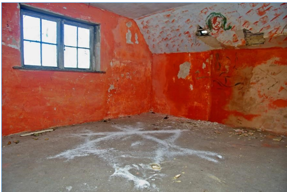
Figure 64 Second floor north west chamber, looking north west
