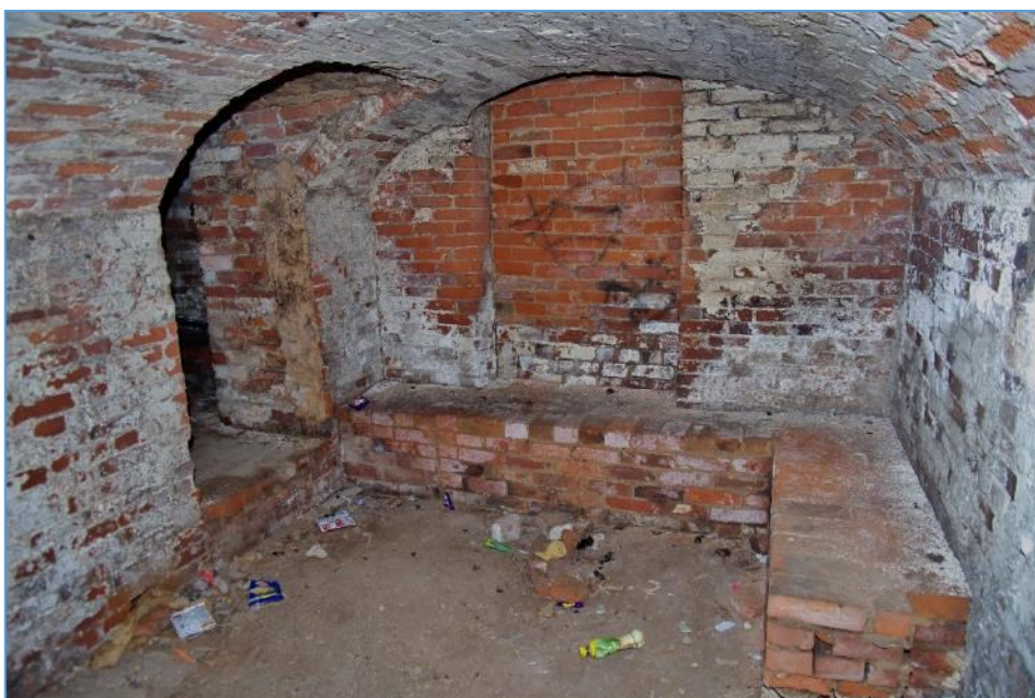
Figure 66 Cellar, beneath reception room, looking east. Note blocking to rear wall
