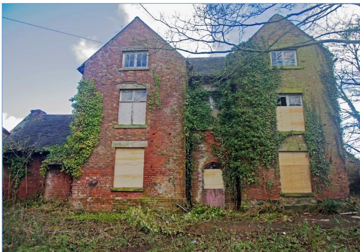
Figure 40 Main (west) façade, looking east
