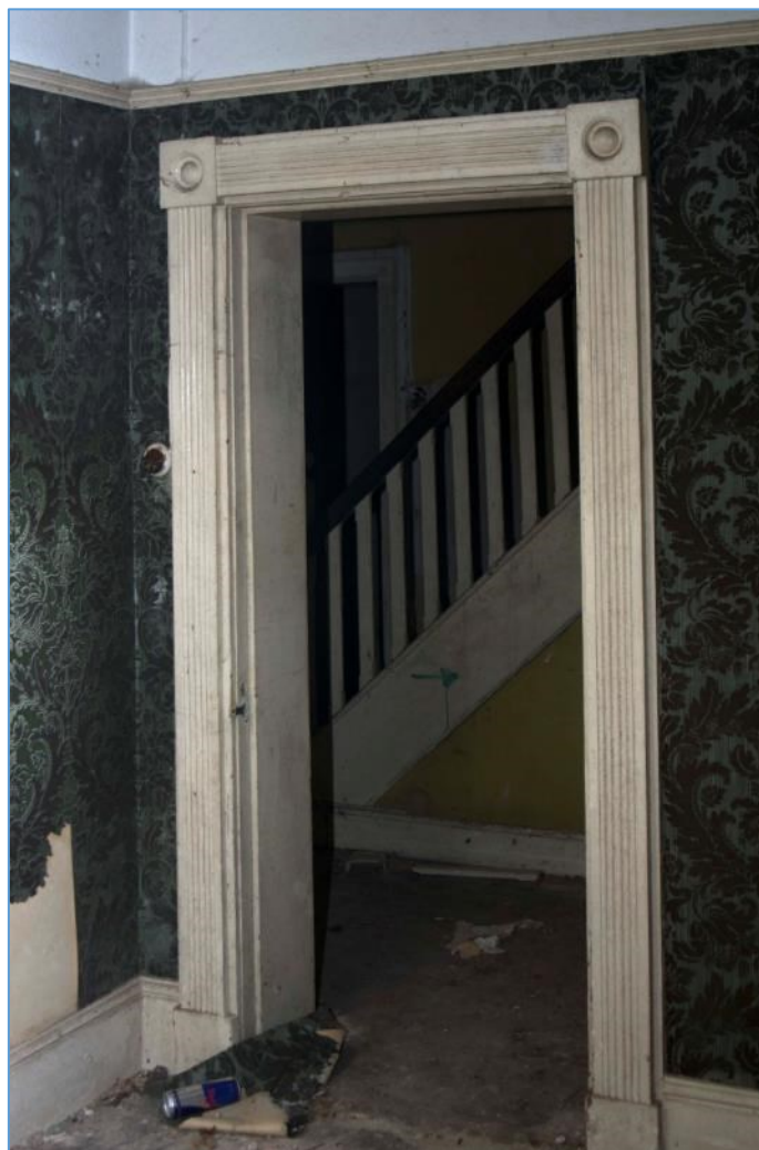
Figure 53 South east reception room door case
