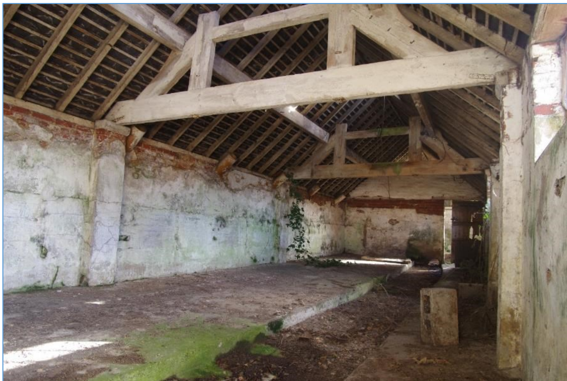
Figure 22 Block C central, looking south-east
