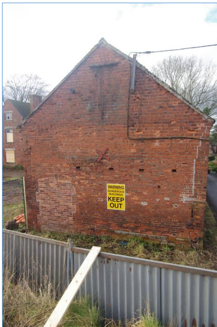
Figure 5 Block A east elevation
