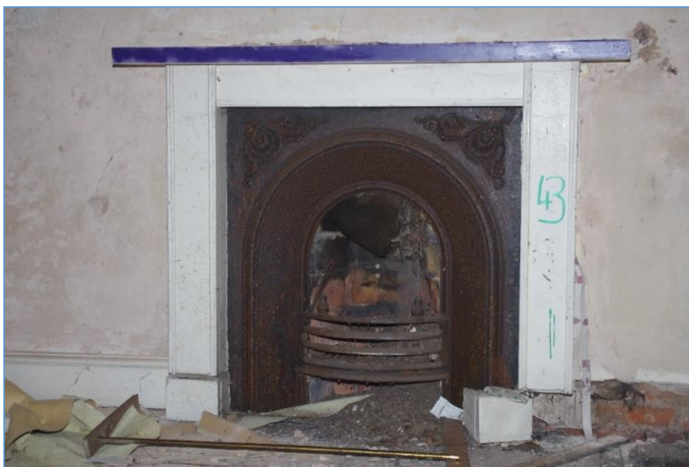
Figure 58 Fireplace in south-east bedroom first floor
