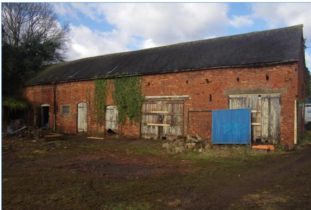
Figure 4 Block A south elevation
