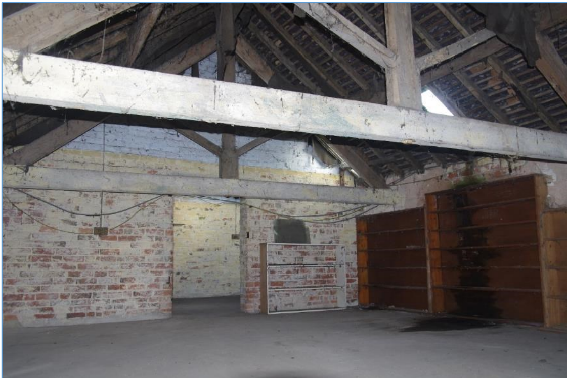
Figure 11 Block A upper floor, west end looking east
