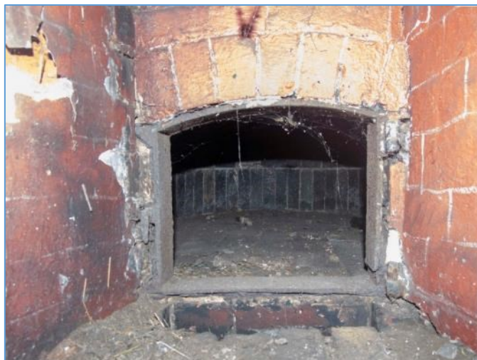
Figure 51 Mouth of oven, showing firebrick back
