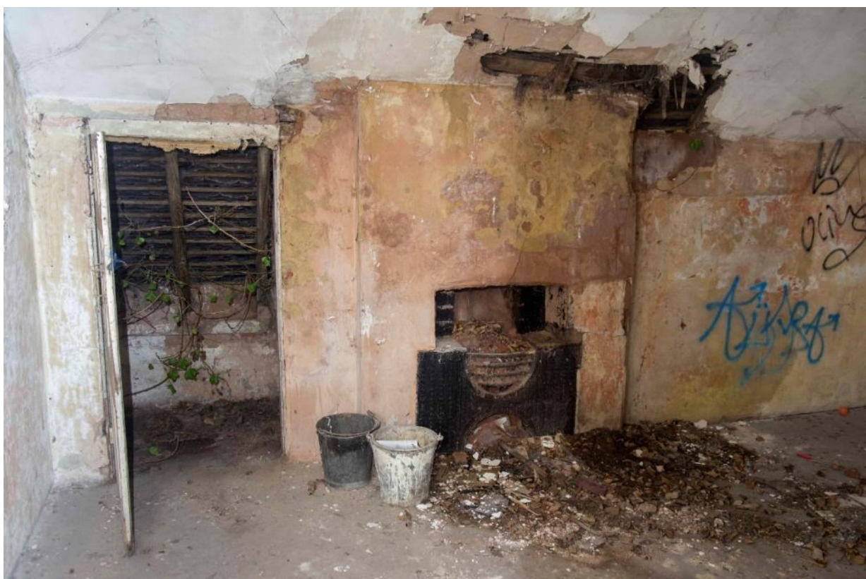
Figure 63 Second floor south west bedroom, looking south. Forest hob grate
