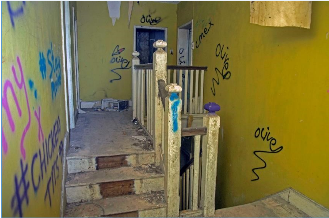
Figure 44 First floor landing, looking west
