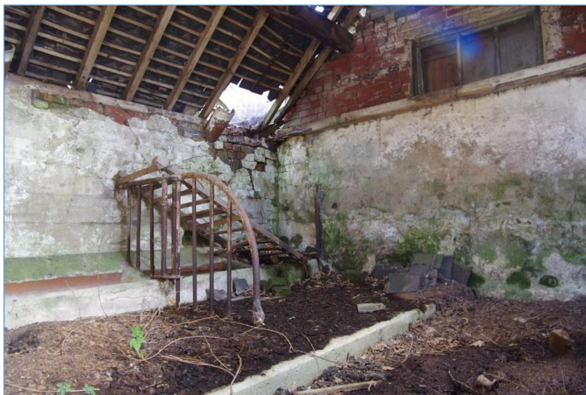
Figure 23 Block C south end, looking south-east
