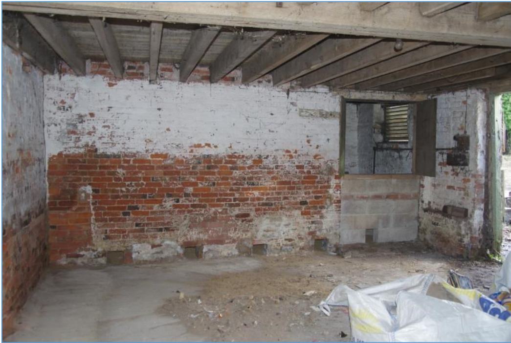
Figure 10 Block A ground floor, west end looking east
