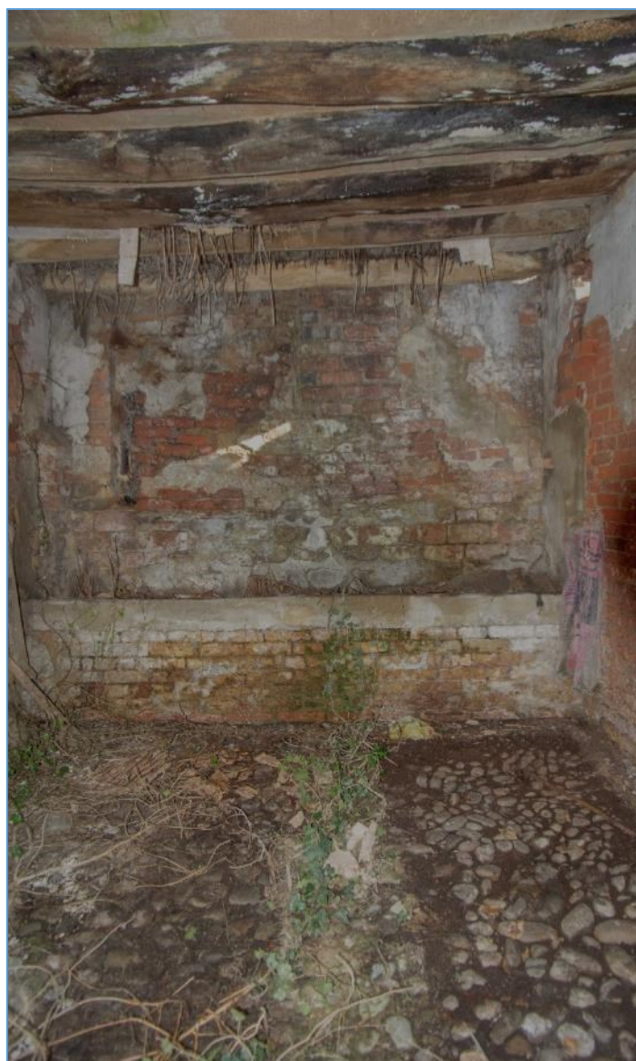
Figure 30 Block E, third stall from the north
