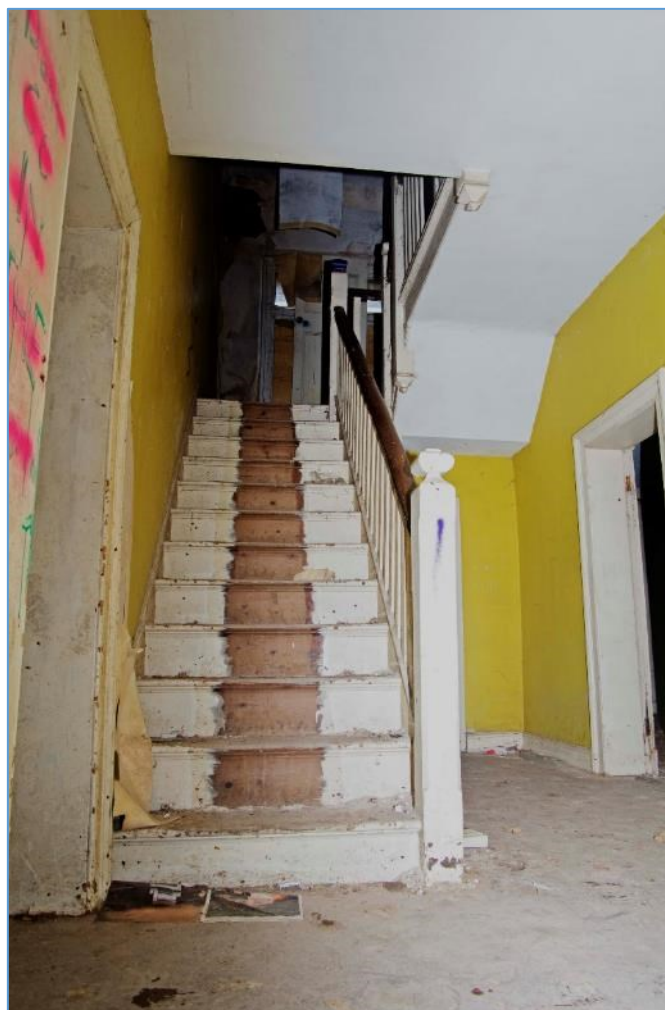
Figure 43 Hall and stairs. Looking east
