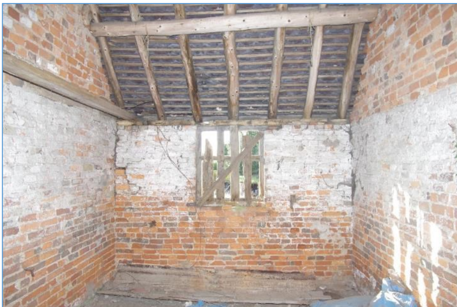
Figure 19 Block B, north unit, looking west.
