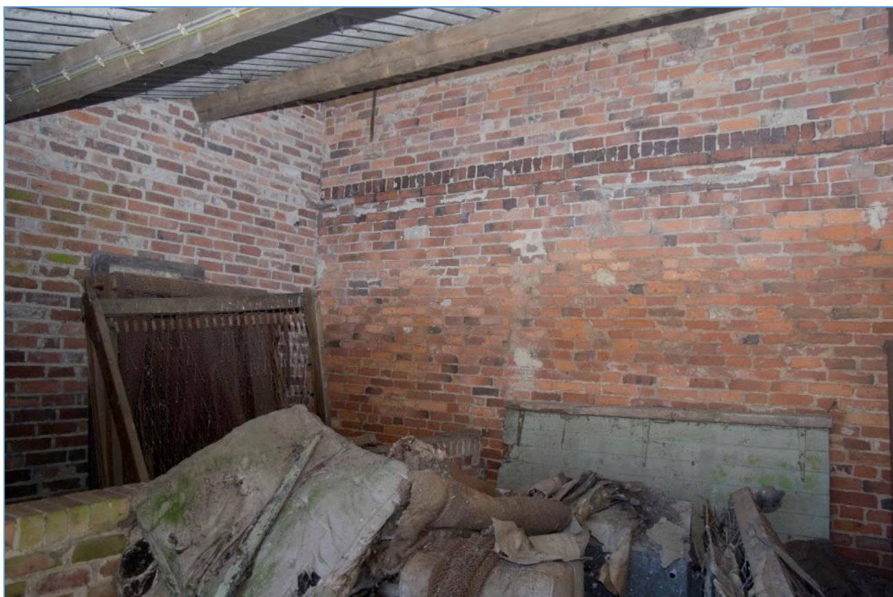
Figure 38 Block G northern unit, looking south west
