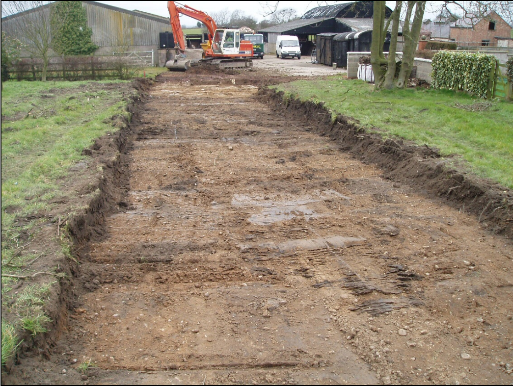
Plate 1. Development site viewed from Ashby Road.
