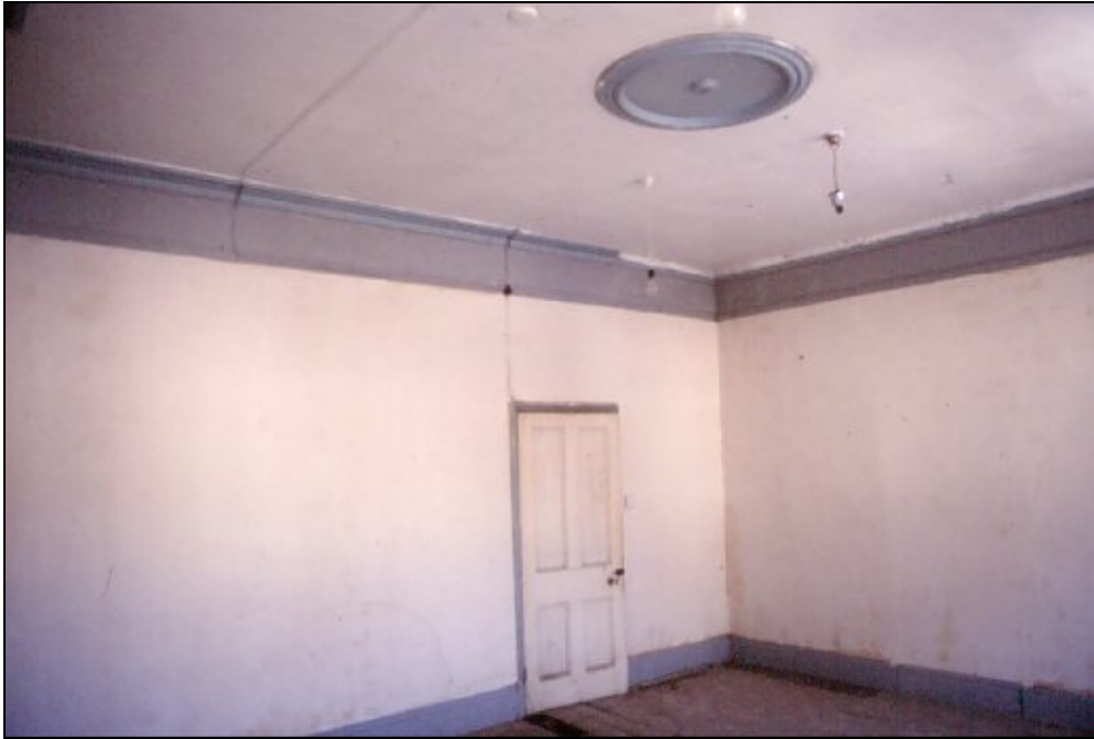
Plate 7. First floor front room of No. 22 with plaster decoration and panelled door.
