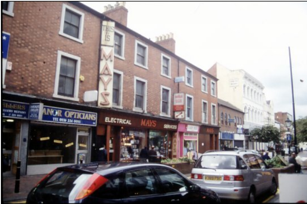
Plate 2. 14 to 22 Churchgate (No. 12 out of shot).
