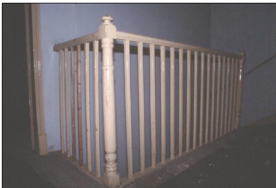
Plate 11. Second floor stairs. Banister and landing in No. 22.
