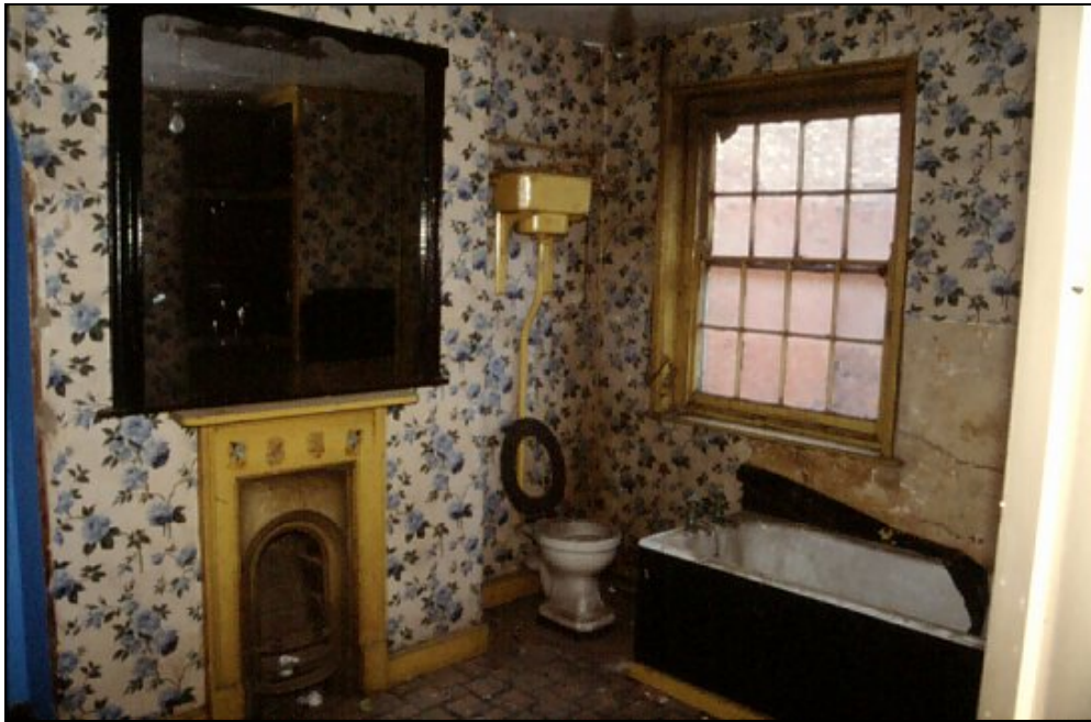
Plate 9. Second floor rear room of No. 22.
