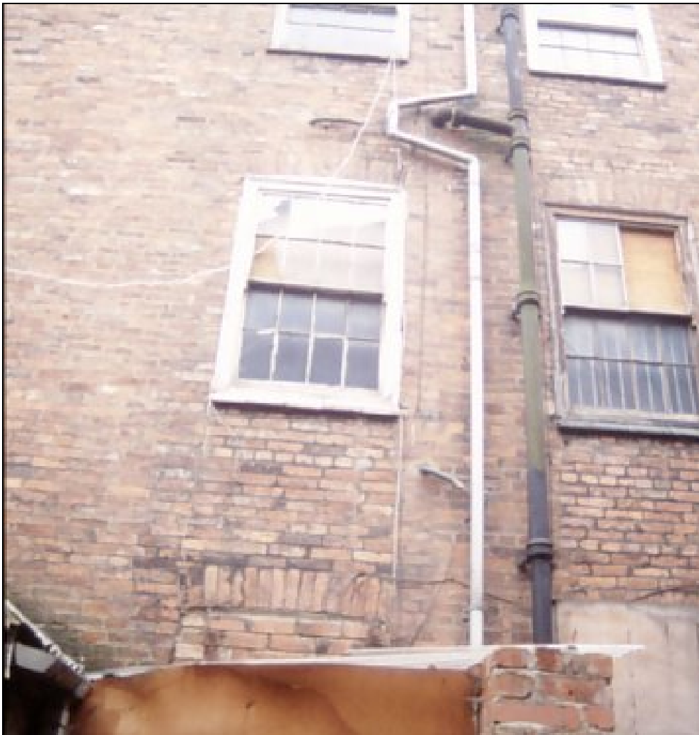
Plate 4. Rear elevation showing sash windows and blocked ground floor windows.
