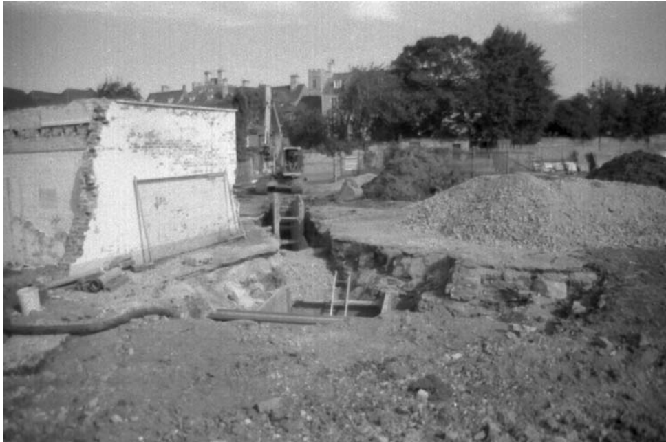
Pl. 1 Watching brief, machining of west service trench, looking north
