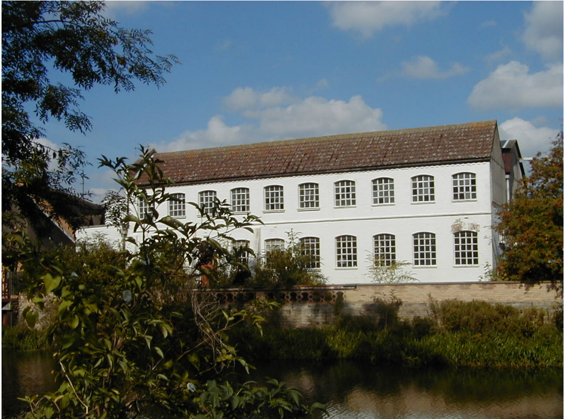
Pl. 2 Exterior of 1902 Stamford Electric Light Company building, looking N, also shows Blashfield terracotta balustrade
