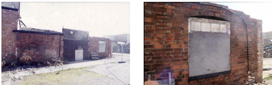
Figure 6 Two Views of Building 4.
