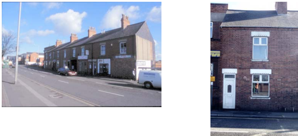
Figure 9 General View & Detailed View of Derby Road Frontage.
