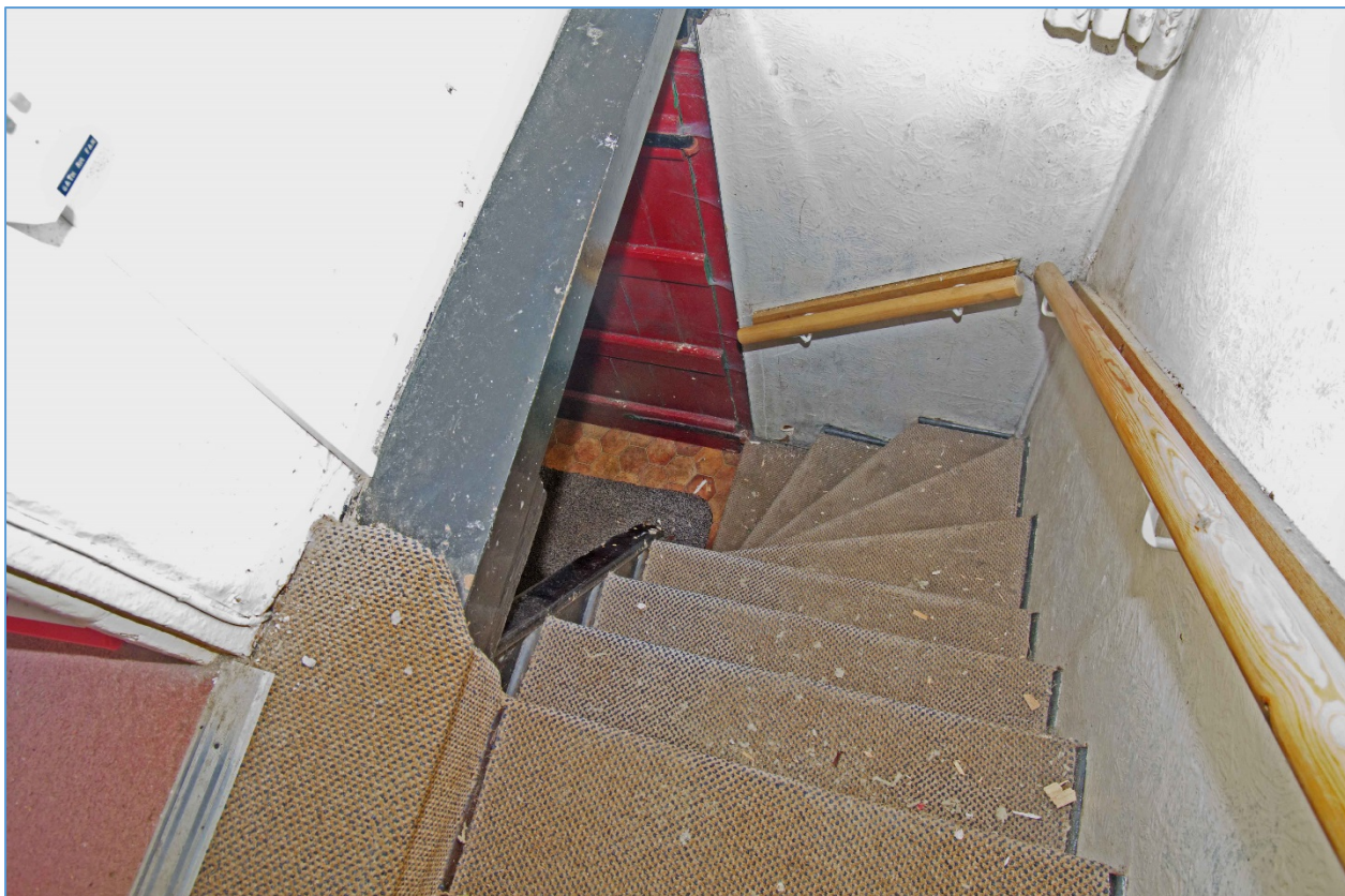
Figure 25 Looking down stairs towards back door
