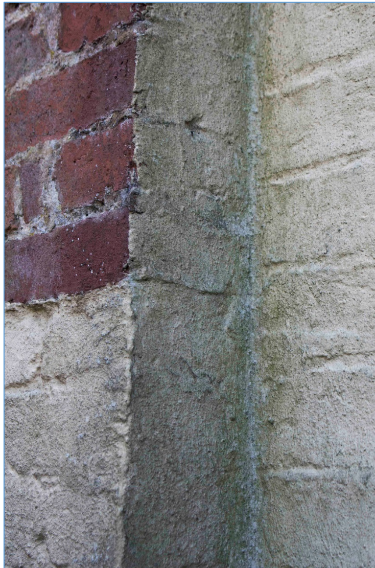
Figure 14 Junction of wing (left) and rear wall (right); detail
