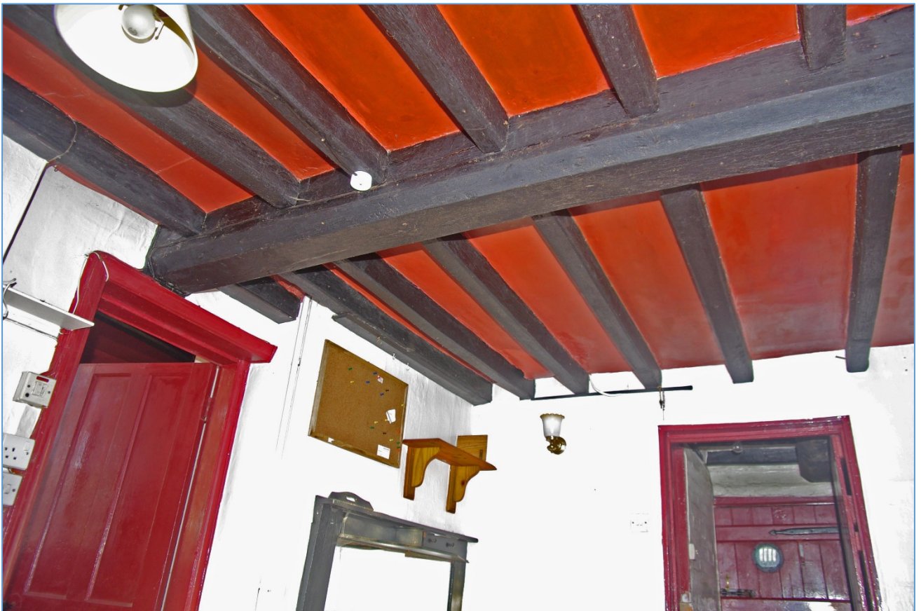
Figure 23 Ceiling structure, looking north. Rear exterior door visible at the back
