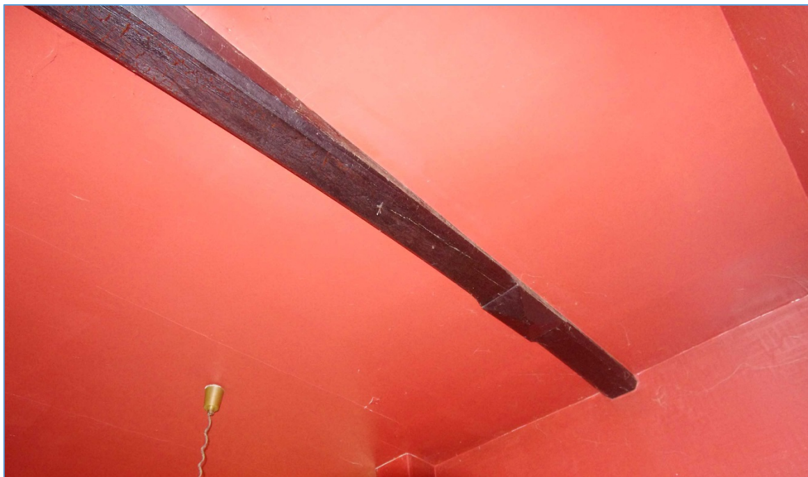
Figure 19 Underside of tie beam showing off-centre boss, disappearing into corridor wall
