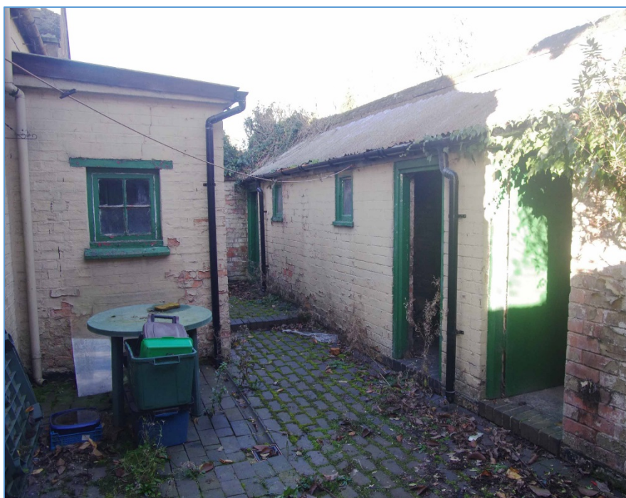
Figure 12 Rear yard, looking north-west. Added bathroom block to the left
