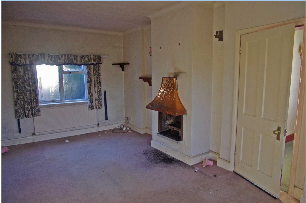
Figure 15 North-west wing ground floor, looking towards rear
