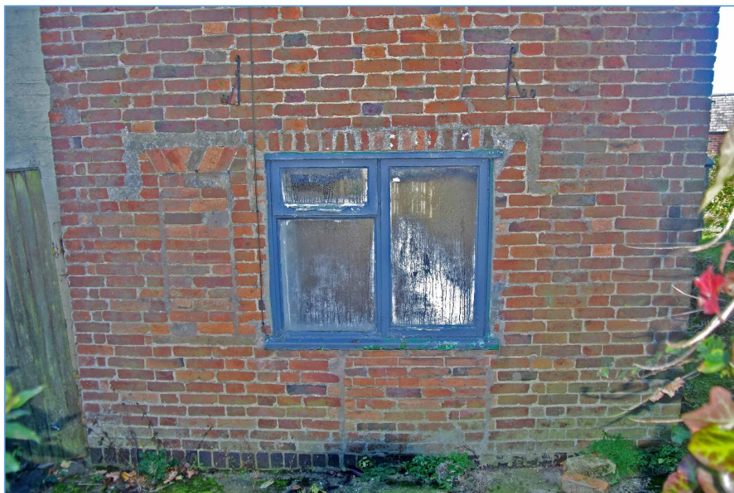
Figure 11 Blocked door and window, north-west wing
