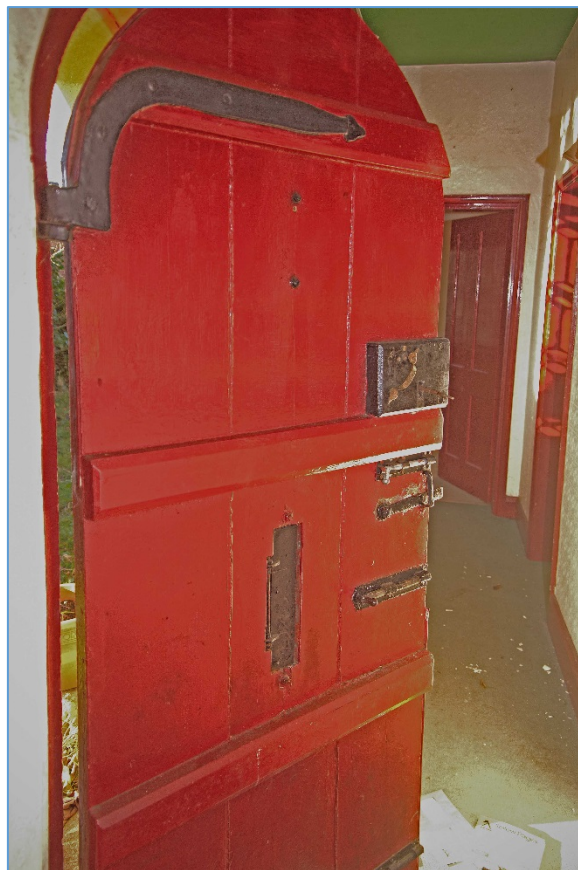
Figure 21 Front door and corridor looking north-west
