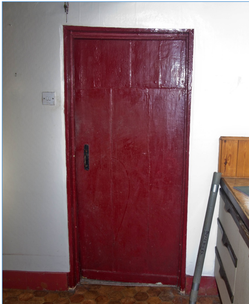
Figure 24 Door into scullery/stairs
