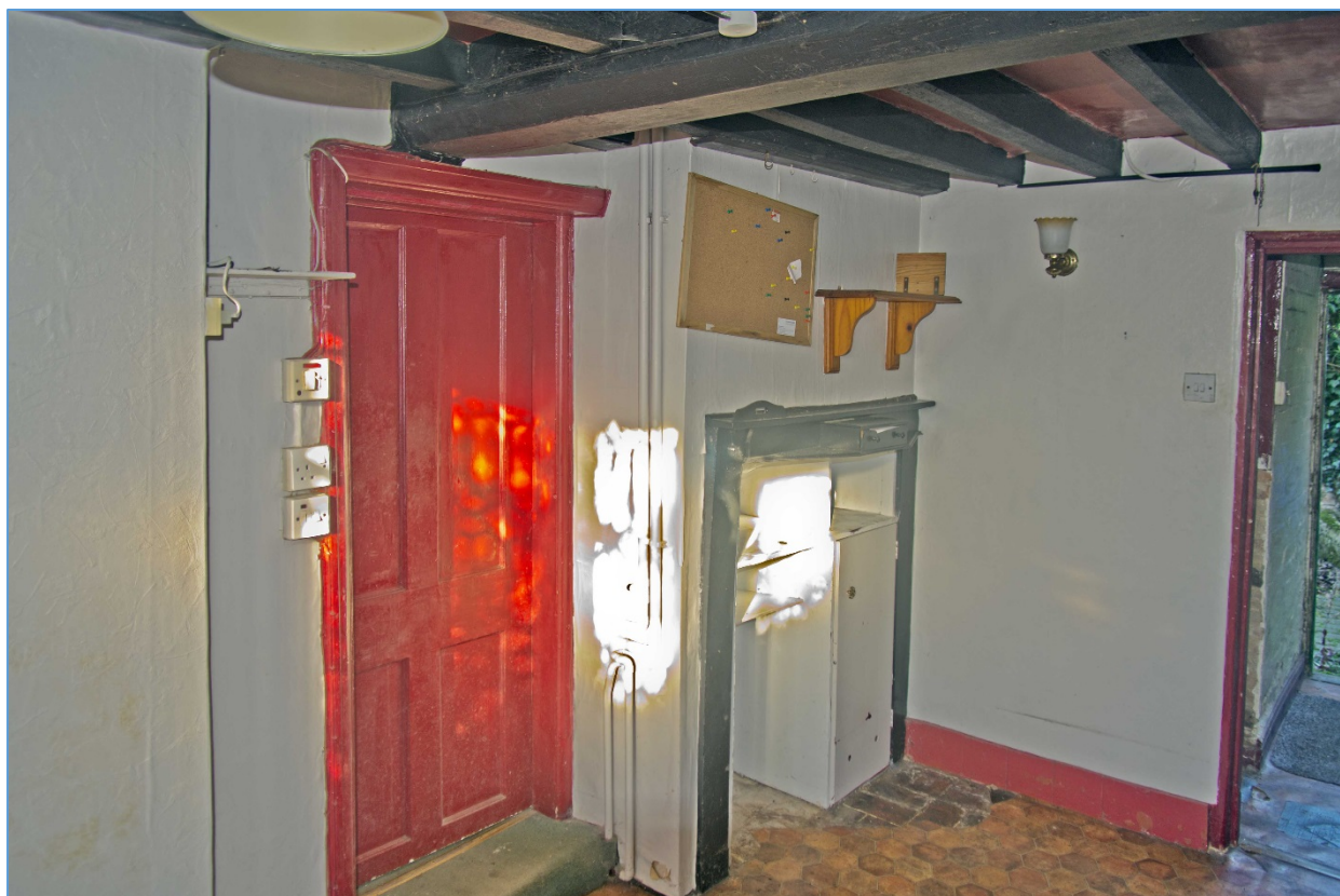
Figure 22 Accomodation wing ground floor, looking north
