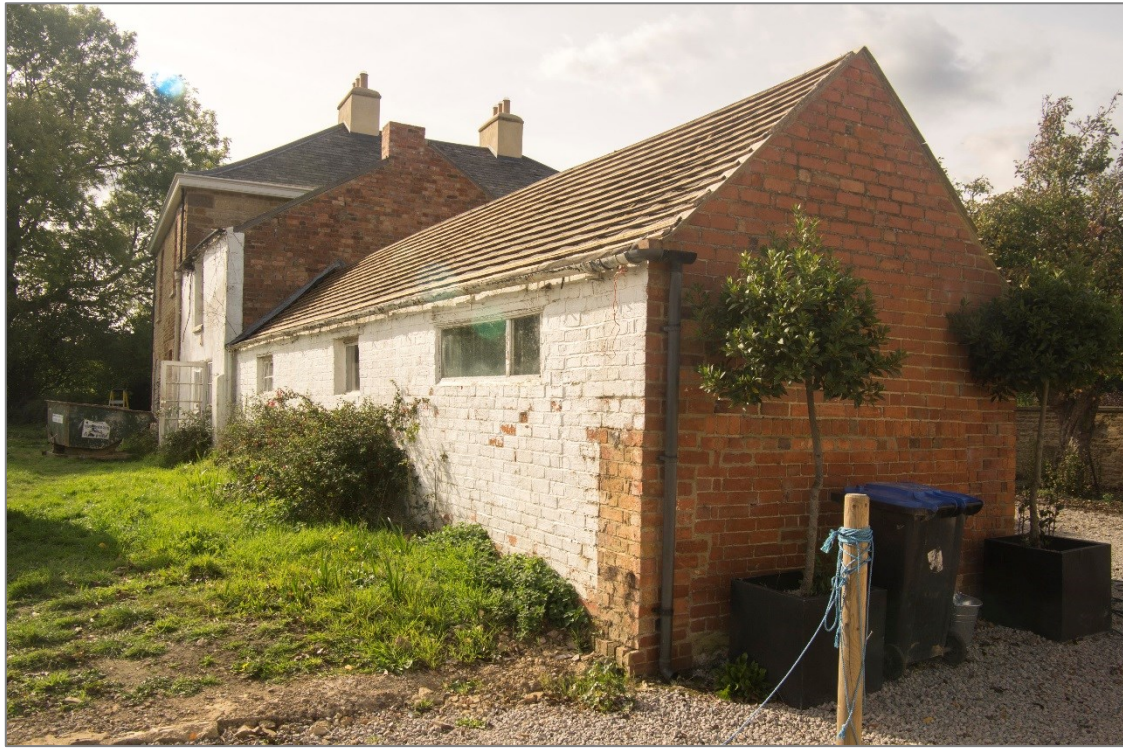
Figure 14 South, and East faces, block E
