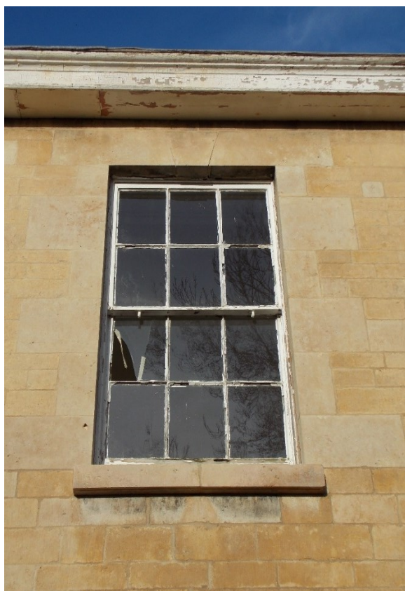
Figure 28 Original hornless sash on west façade. Photo provided by client
