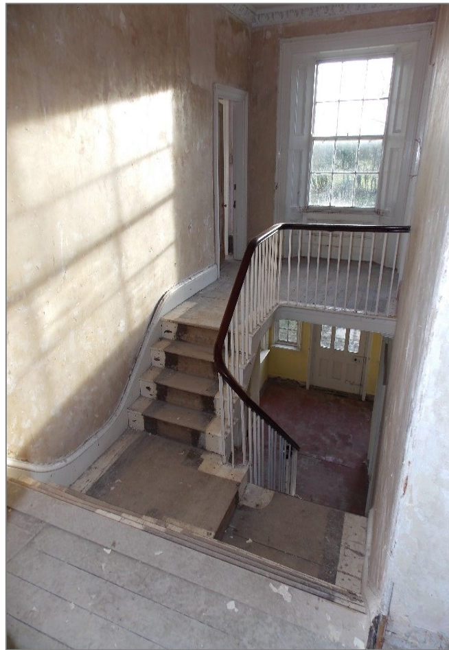
Figure 29 Stairway, before renovation. Photo provided by client
