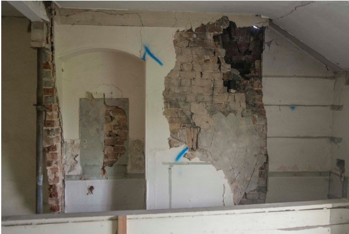
Figure 23 Block D upper floor, blocked fireplace and flue above removed range
