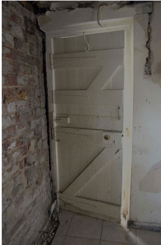
Figure 16 Stable door between blocks D and E
