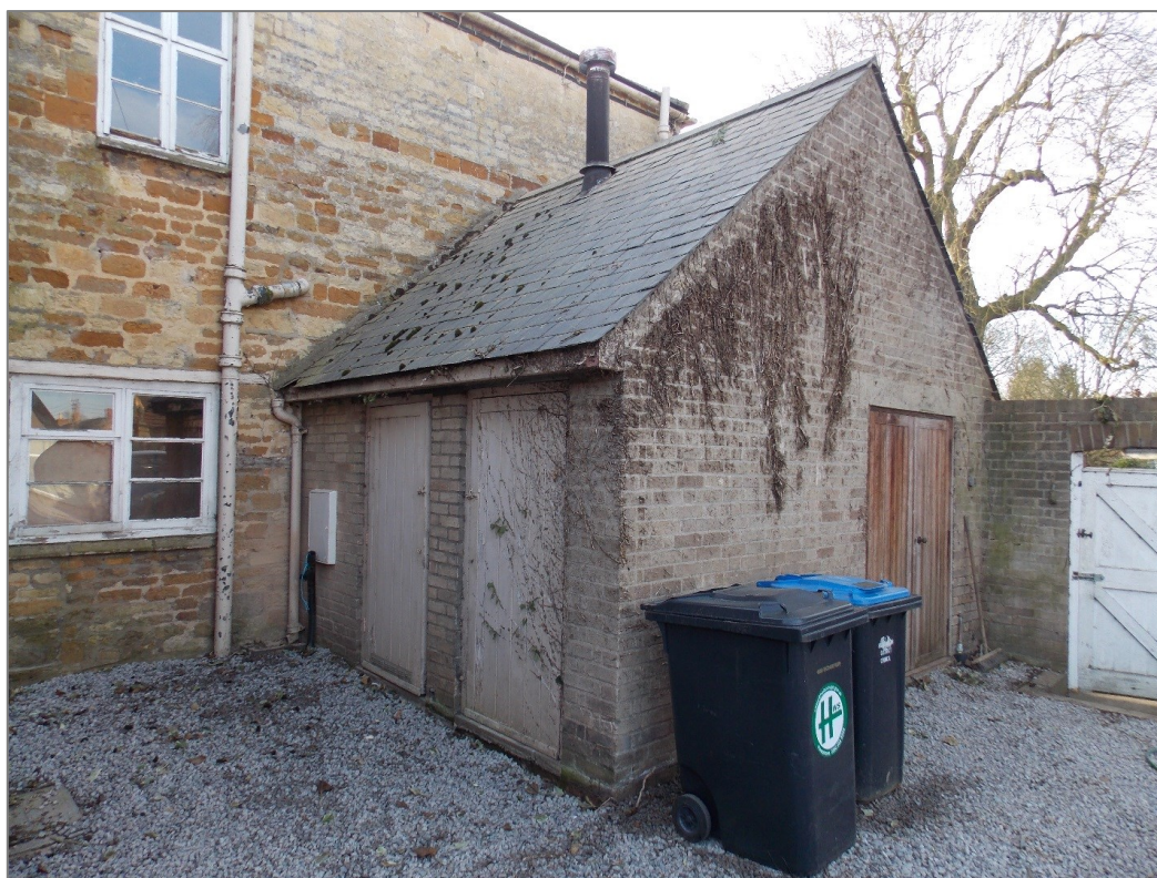
Figure 9 Block C, looking north-west
