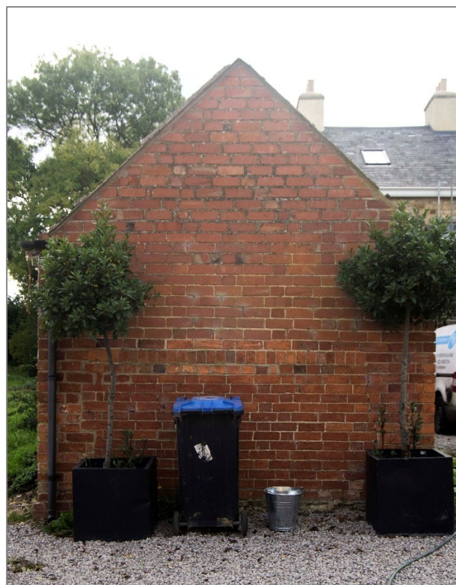
Figure 13 East end of block E
