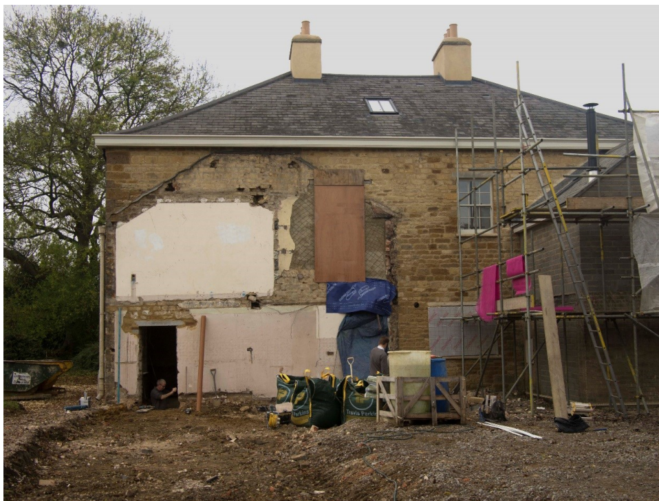
Figure 25 Main house, east side after removal of outbuildings.
