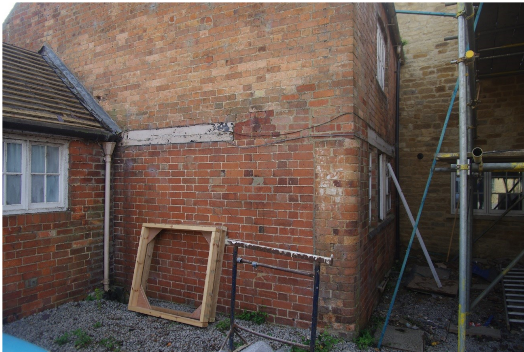
Figure 19 Block D looking west. Note bull-nose pier and blocked openings
