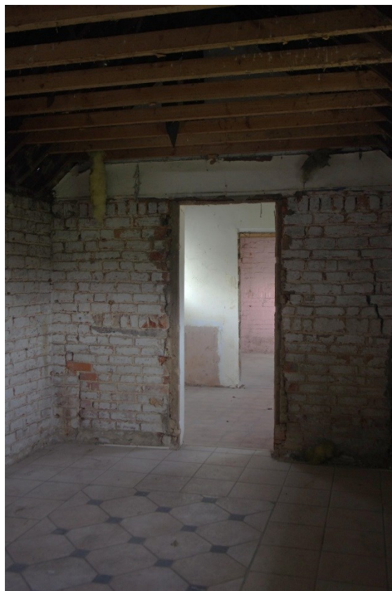
Figure 17 Block E, looking east to gable end wall (pink)
