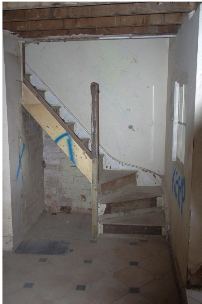
Figure 22 Block D stairs
