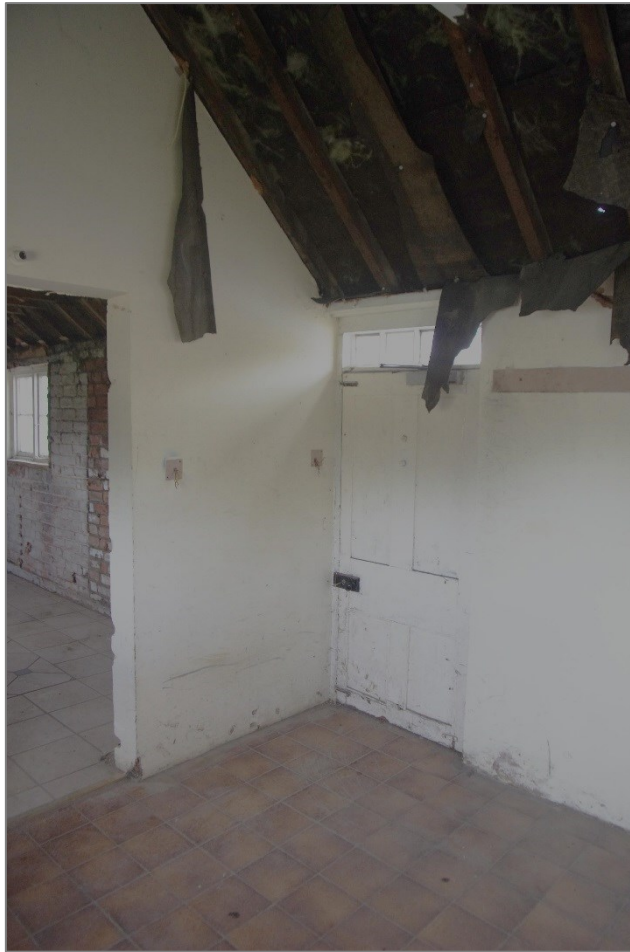
Figure 18 Block E, looking north-east to present entrance door
