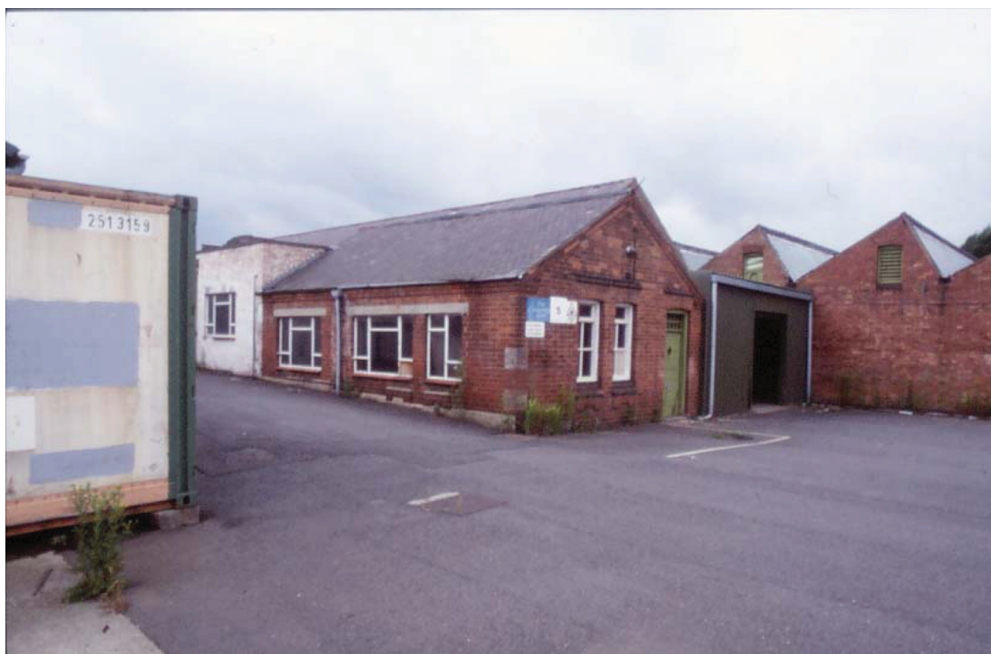
Colour Plate 2 Room on North Westernmost Gable of Building 2/Bay 4.
