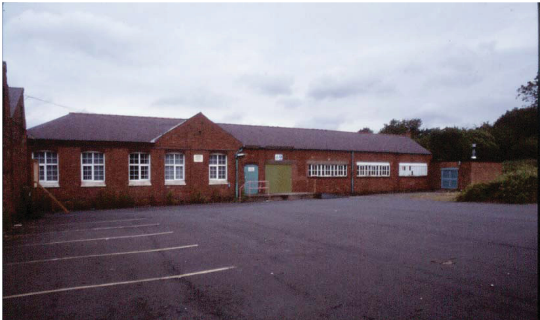
Colour Plate 1 Building 1, Southwest Facing Elevation.
