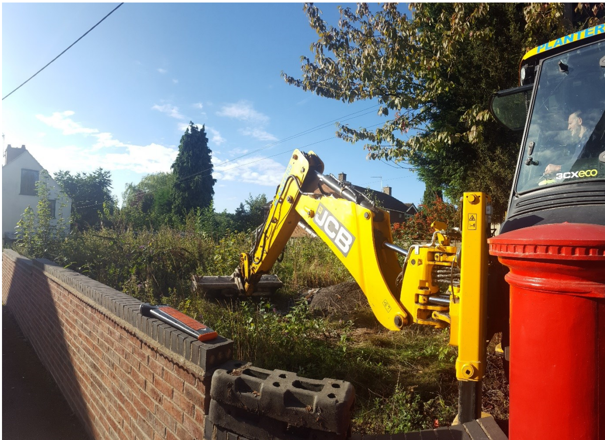
Figure 2: Site during initial clearance work. Looking south-east.
