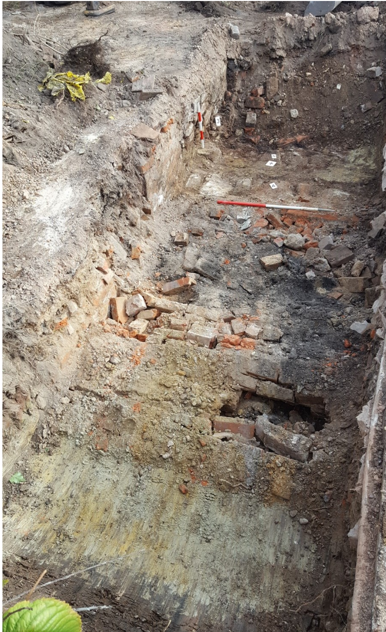
Figure 10: West end of Trench 2, natural ground level and showing brick culvert in foreground and backfilled cellar.
