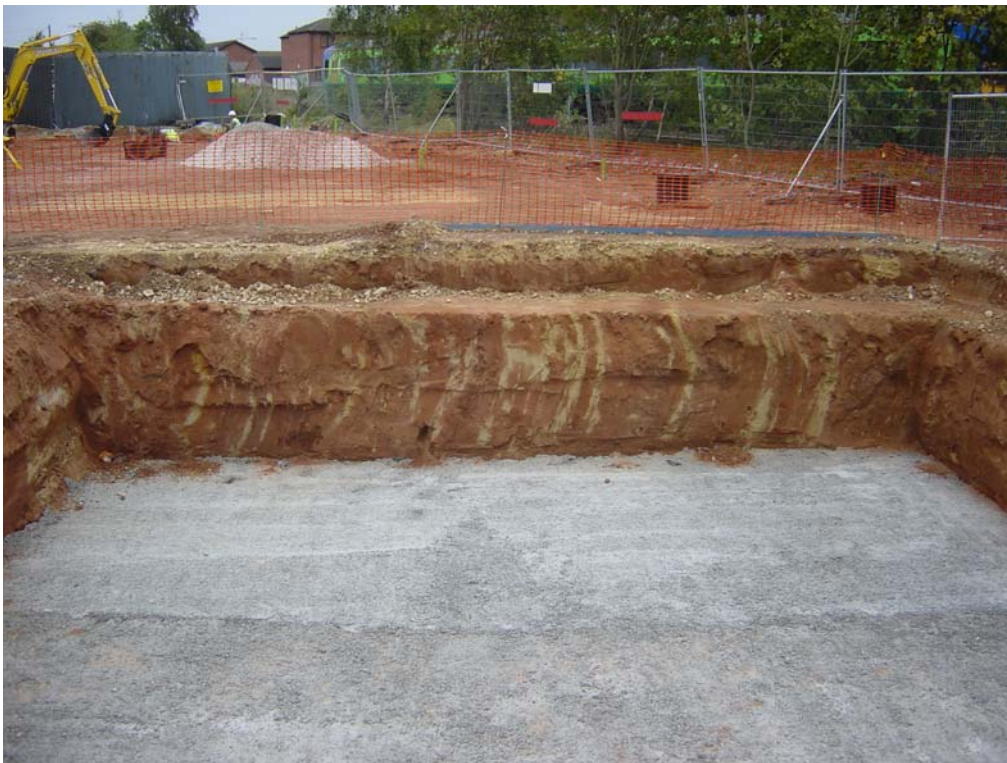
Colour Plate 1 South Facing Section of Northernmost Crane Base.
