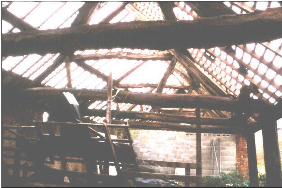
Colour Plate 3 Barn 3 Detail of Roof Construction
