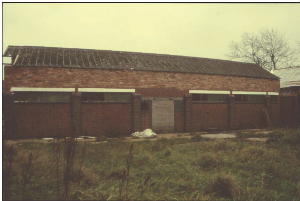
Colour Plate 1 Barn 1 Northwest Facing Elevation.
