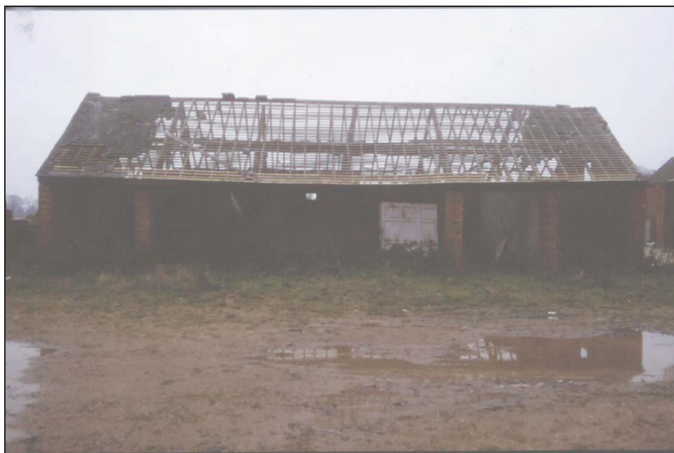
Colour Plate 2 Barn 3 Northwest Facing Elevation.
