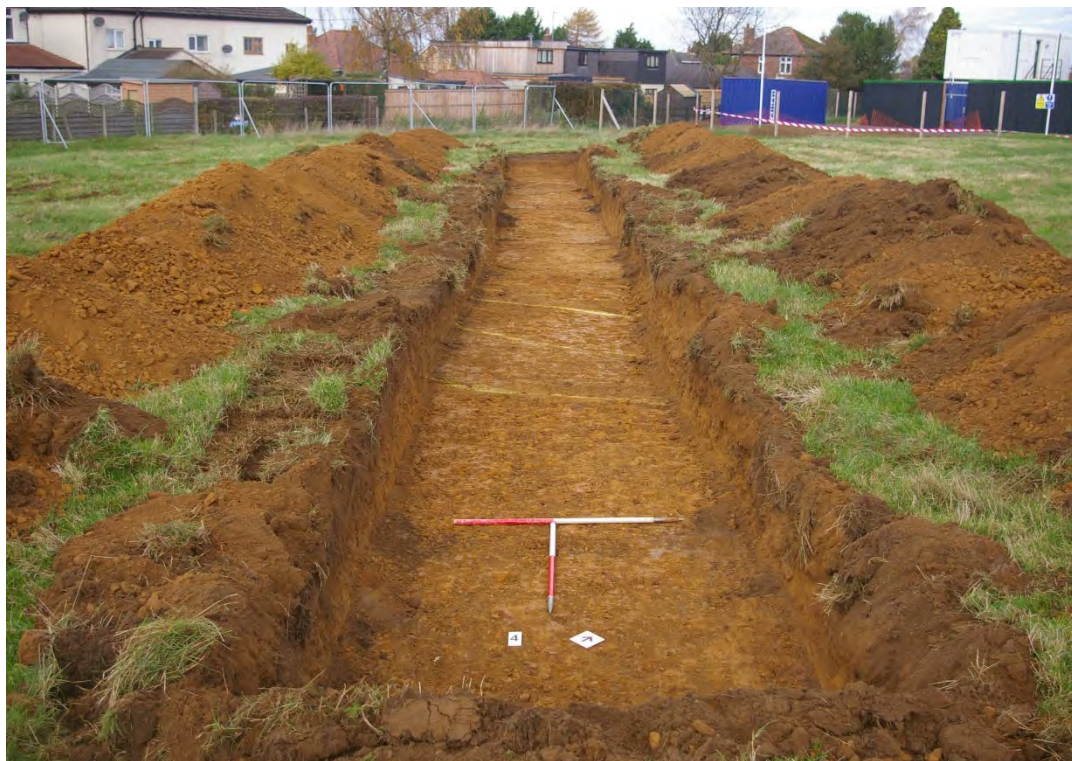
Figure 17: Trench 4 looking North-West
