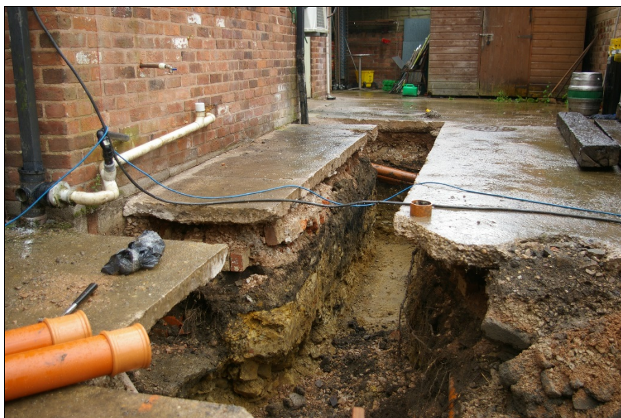
Figure 5: Natural substratum observed in small area of trench, drains visible
