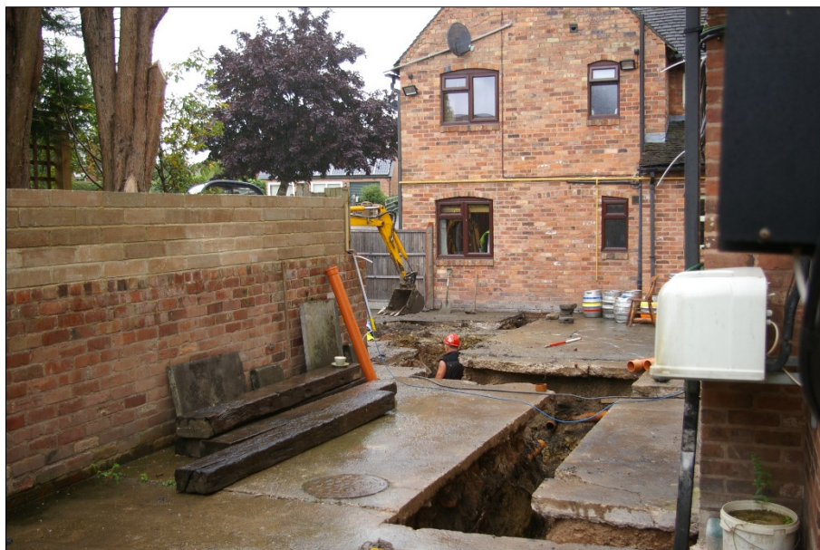
Figure 8: Trench following completion of excavation, looking north
