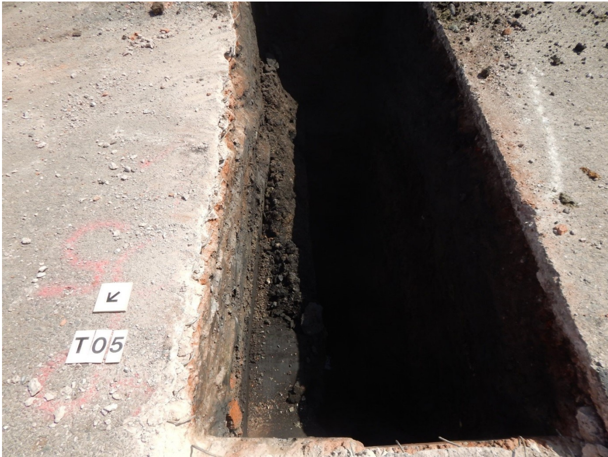
Figure 7: TP05 post-excitation, looking south-east
