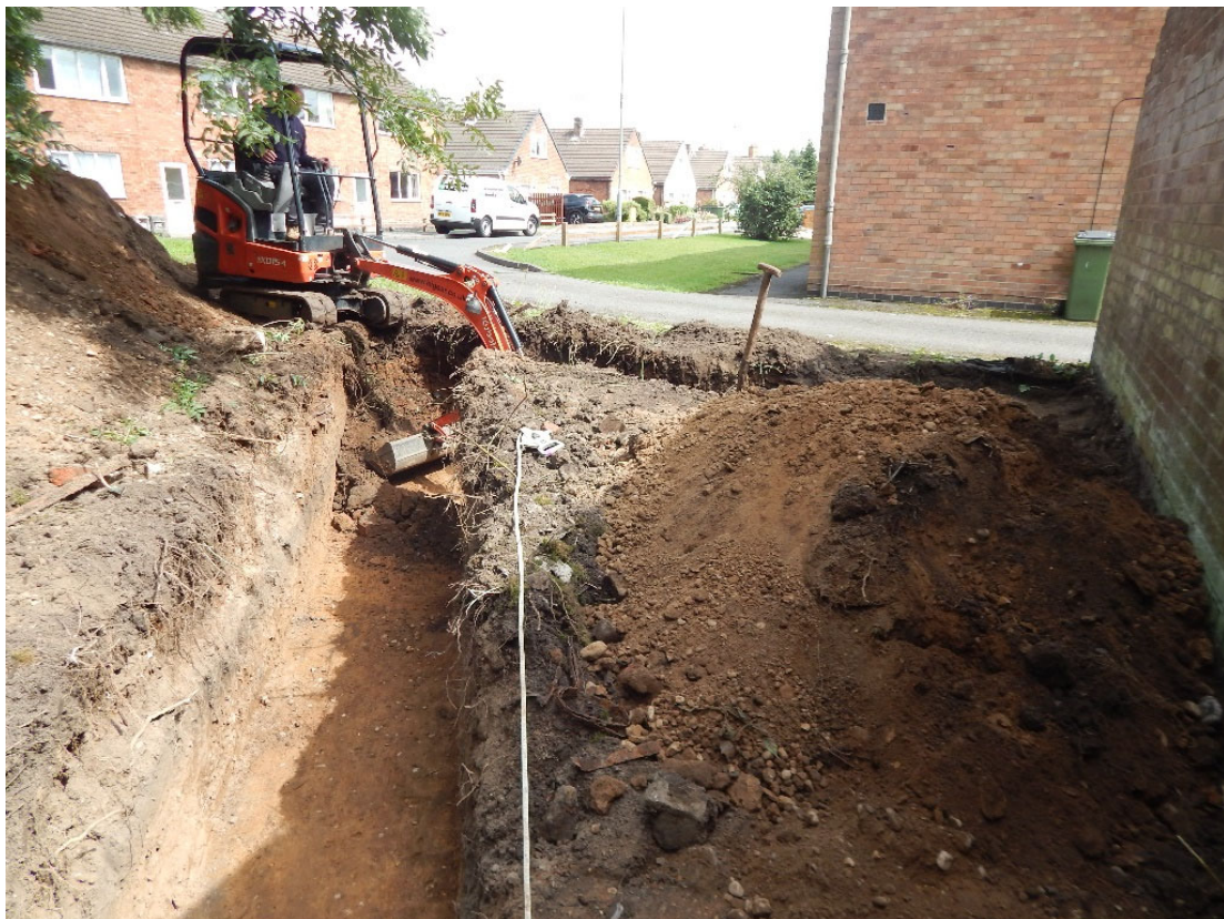
Figure 6: Excavation of Trench 2 in progress, within Building Plot C
