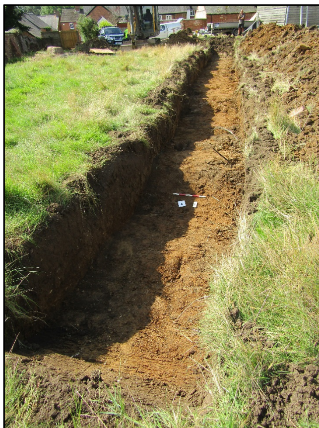
Figure 8: Trench 1 looking south west
