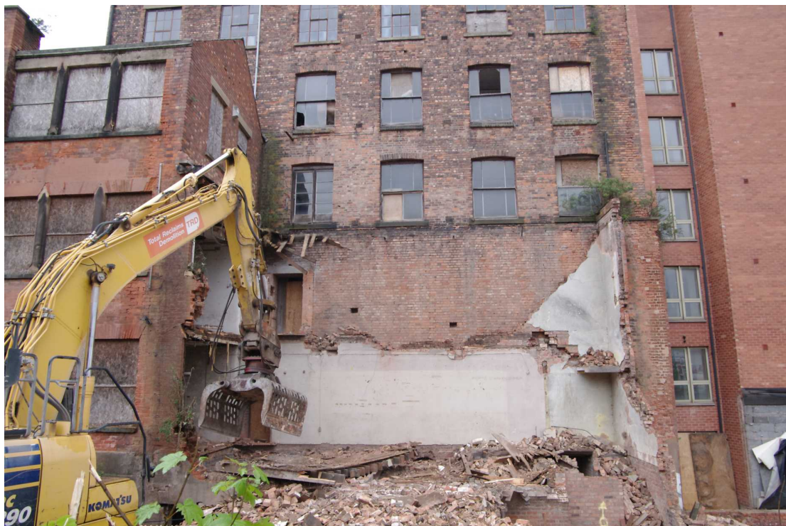
Figure 33 Rear (southern) section of 10 Short Hill during demolition Looking east
