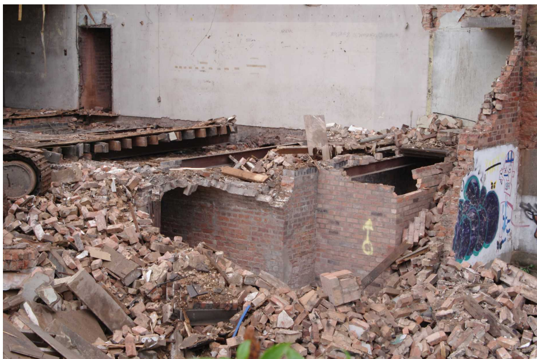
Figure 34 Rear (southern) section of 10 Short Hill, basement Looking north-east
