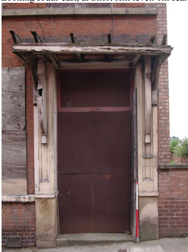
Figure 18 Number 10 Short Hill, north facing elevation. Doorway Looking south. 1m scale
