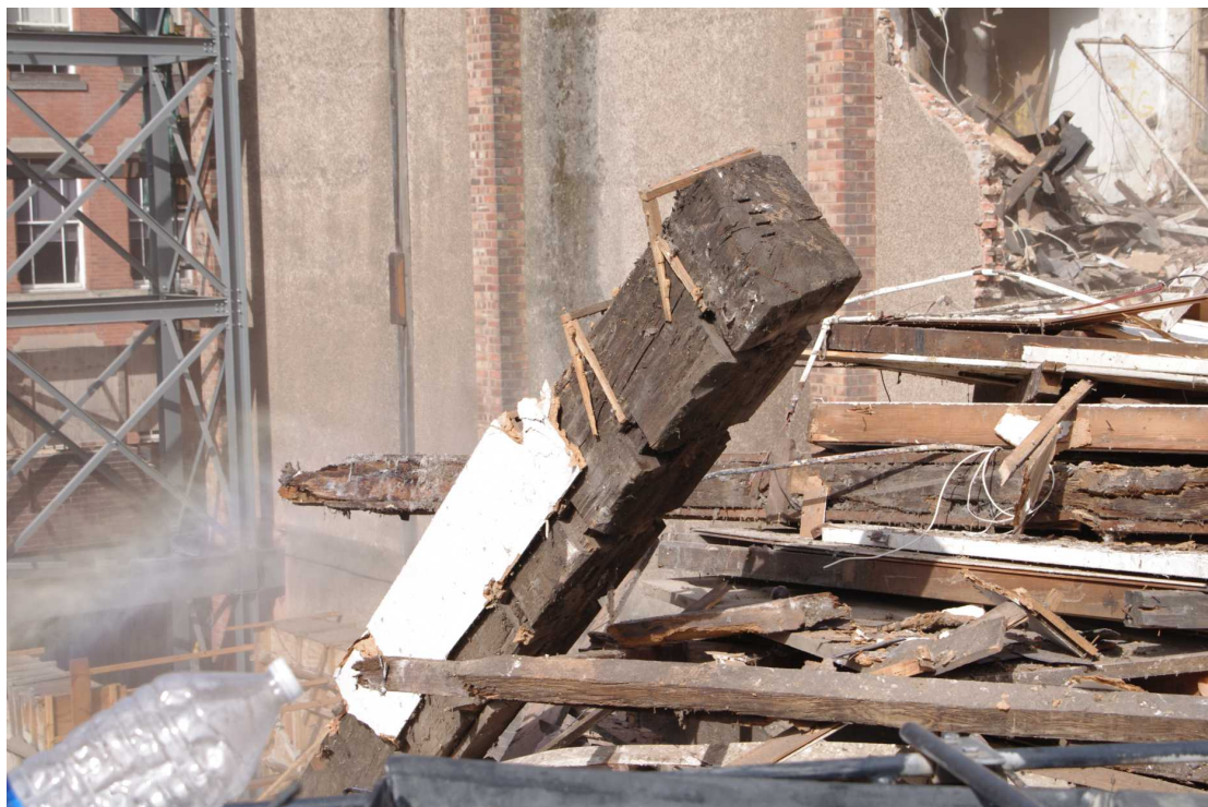
Figure 41 Northern section truss with carpenter's marks on end
