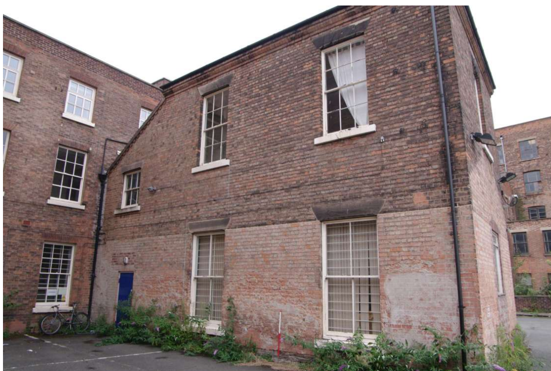
Figure 53 19th century extension, west facing elevation Looking north-east. 1m scale
