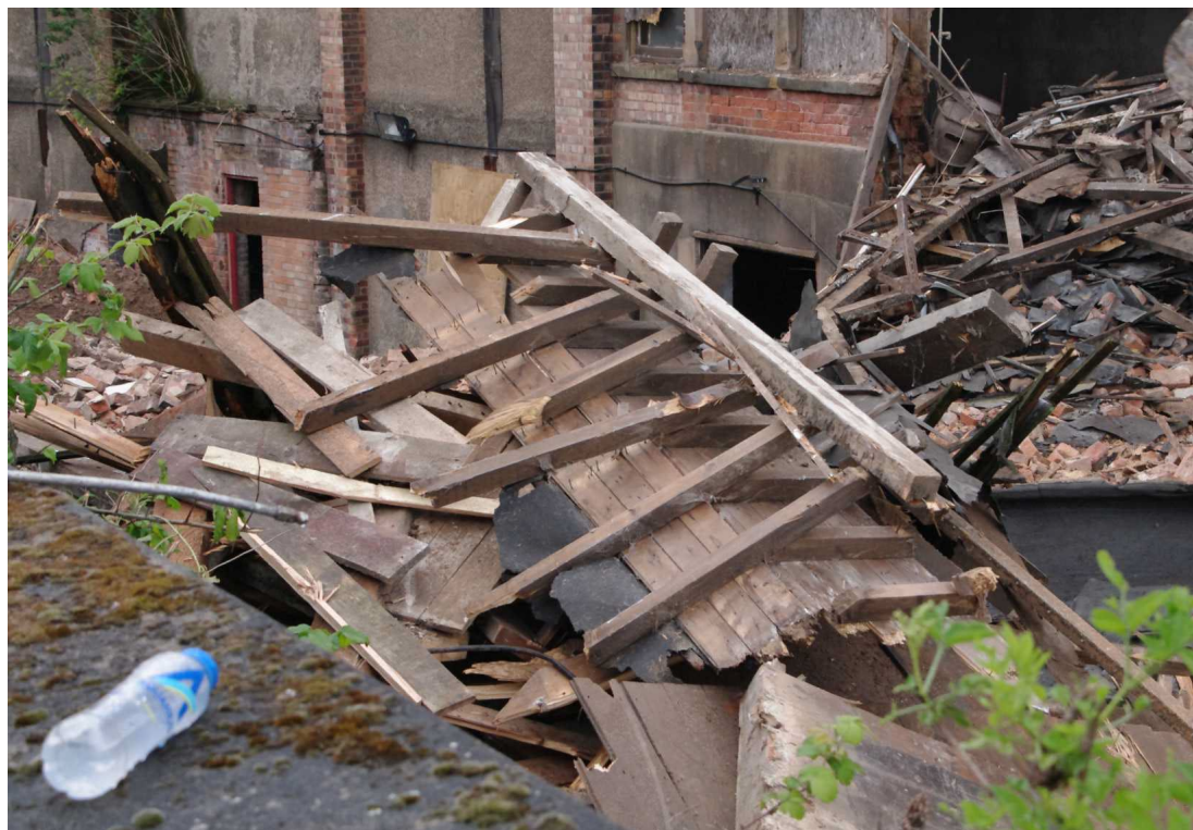
Figure 37 Centre section roof structure After removal of roof
