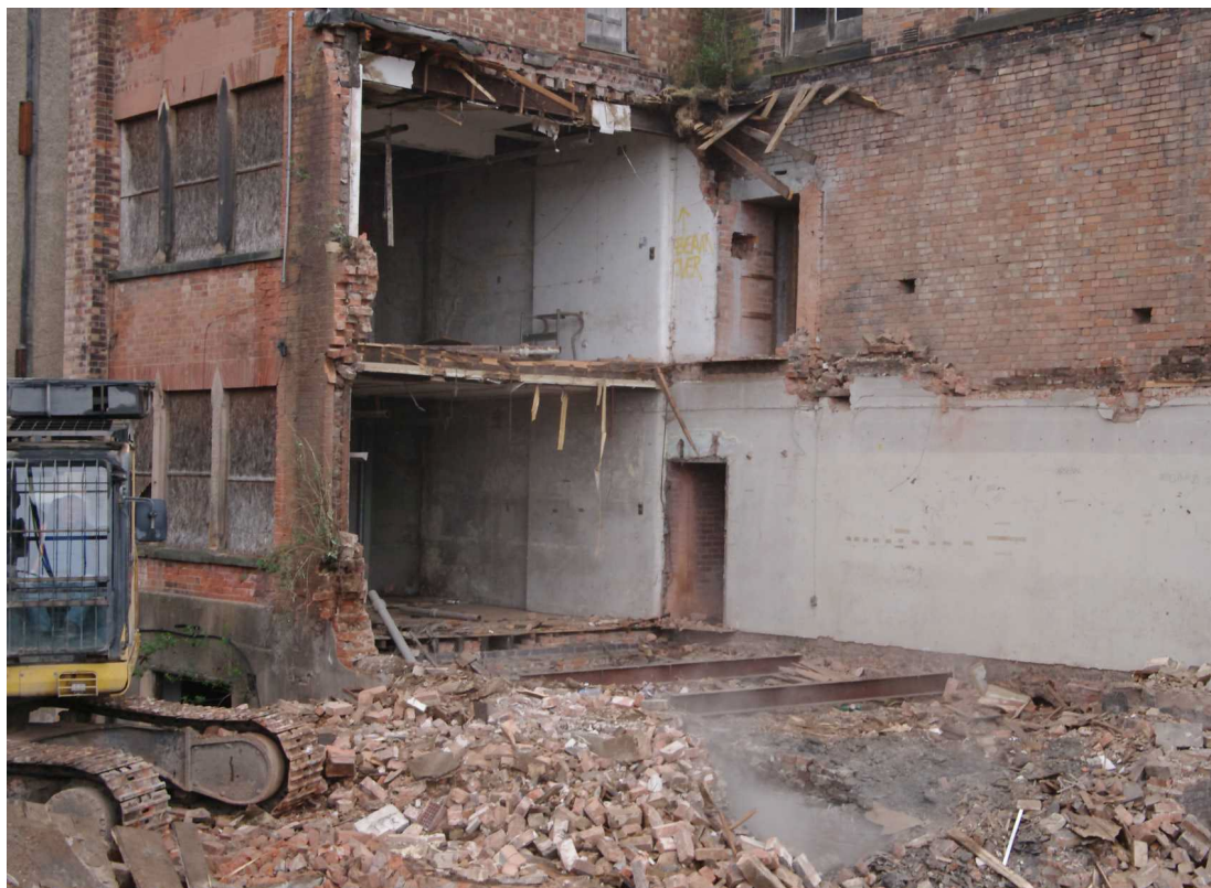
Figure 35 Centre section, close-up of ground and first floor rooms Looking north-east
