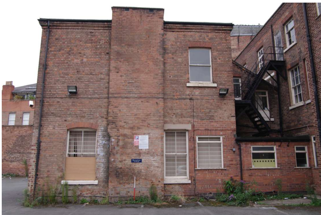
Figure 50 19th century extension, east facing elevation Looking west. 1m scale
