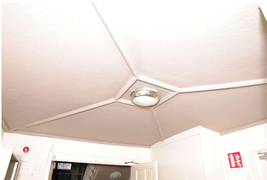
Figure 56 Ceiling detail of link between Number 56 and 19th century extension
