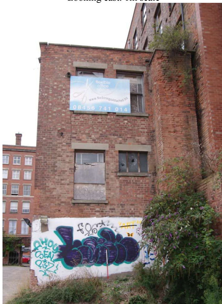
Figure 27 Number 10 Short Hill, south facing elevation. Looking north. 1m scale
