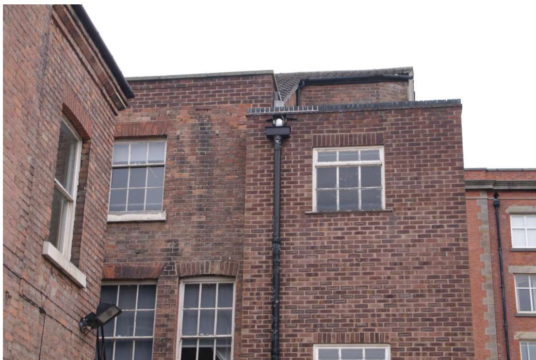
Figure 64 1960s extension, south facing elevation and roof level joint Looking north
