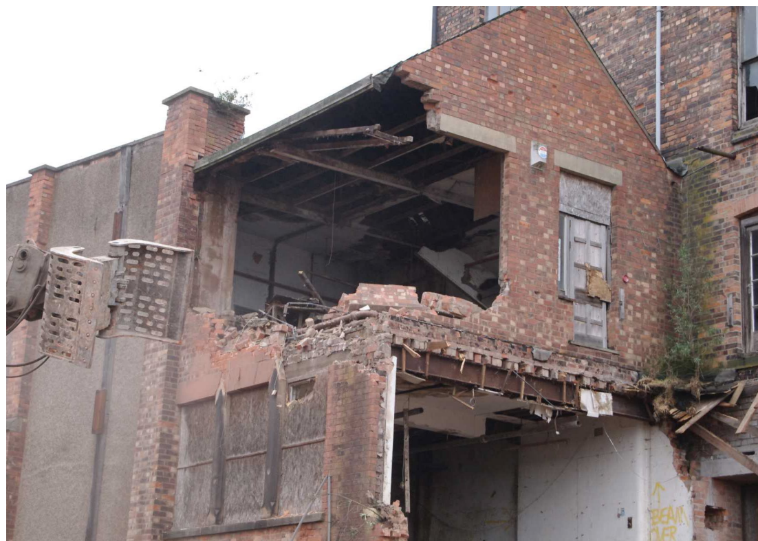
Figure 36 Centre section, demolition of second floor Looking north-east
