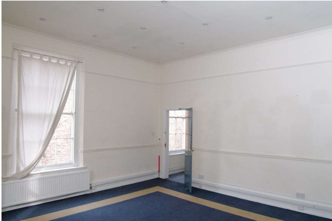
Figure 61 19th century extension first floor Looking north-west. 1m scale
