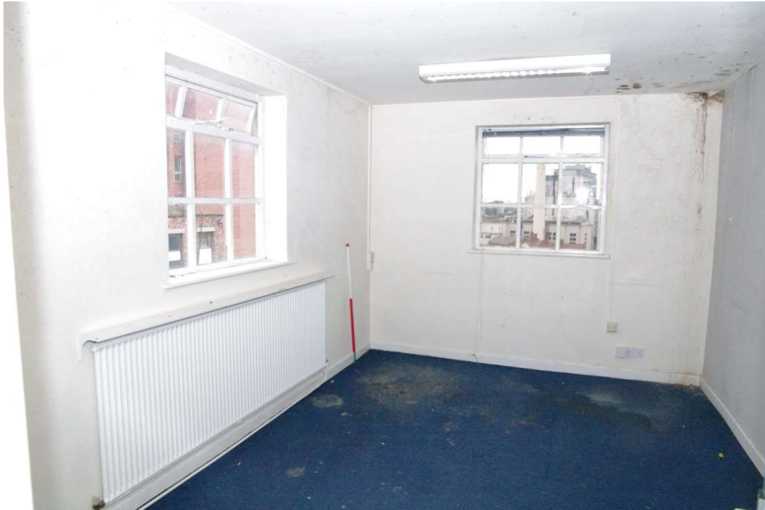
Figure 68 1960s extension, second floor room Looking south-east. 1m scale
