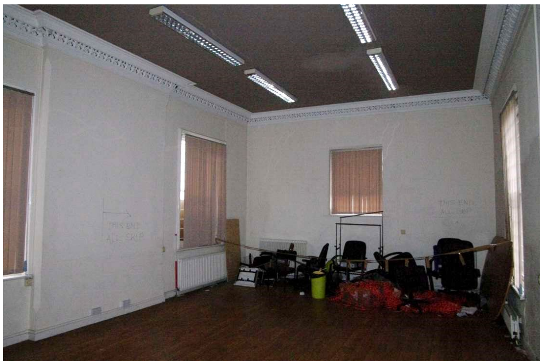
Figure 57 Ground floor room of 19th century extension Looking south-east. 1m scale
