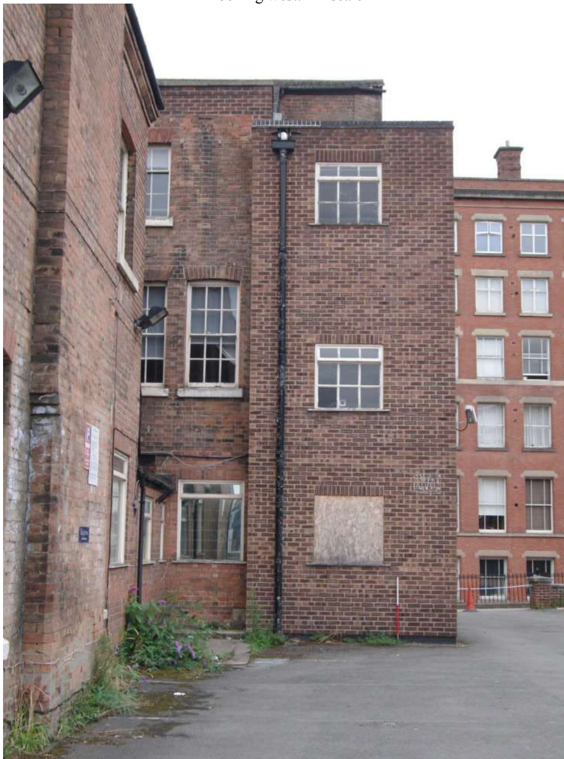
Figure 63 1960s extension, south facing elevation Looking north. 1m scale
