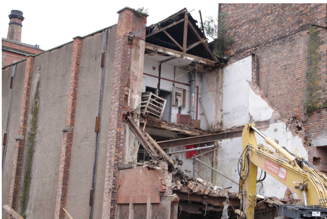
Figure 38 Roof structure linking truss between front and centre sections, Looking north-east
