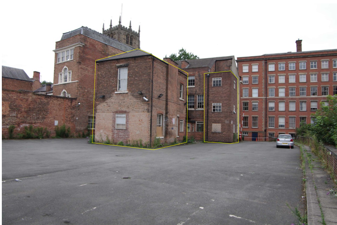
Figure 12 Rear of 56 High Pavement Looking north-west from car park. Surveyed components highlighted
