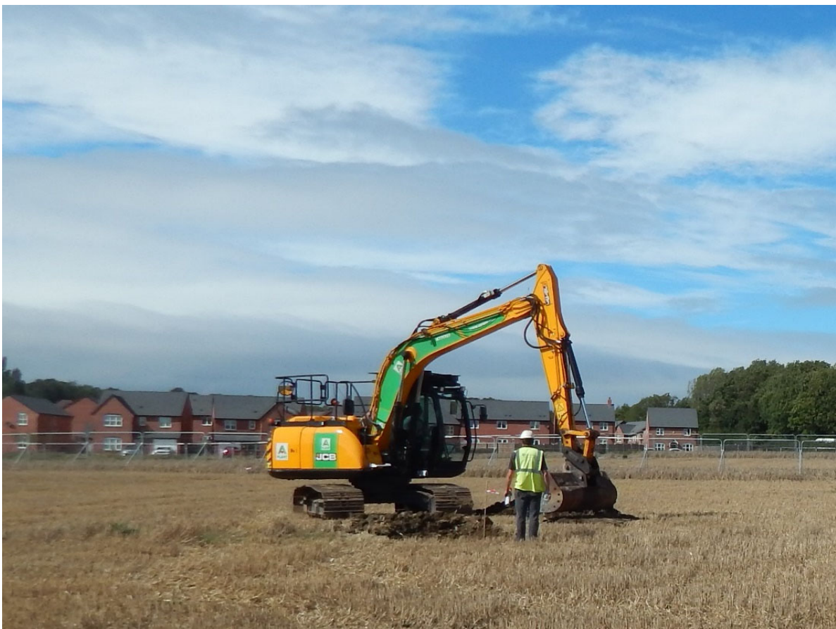
Figure 9: Excavation in progress of Trench 2, looking south-east.
