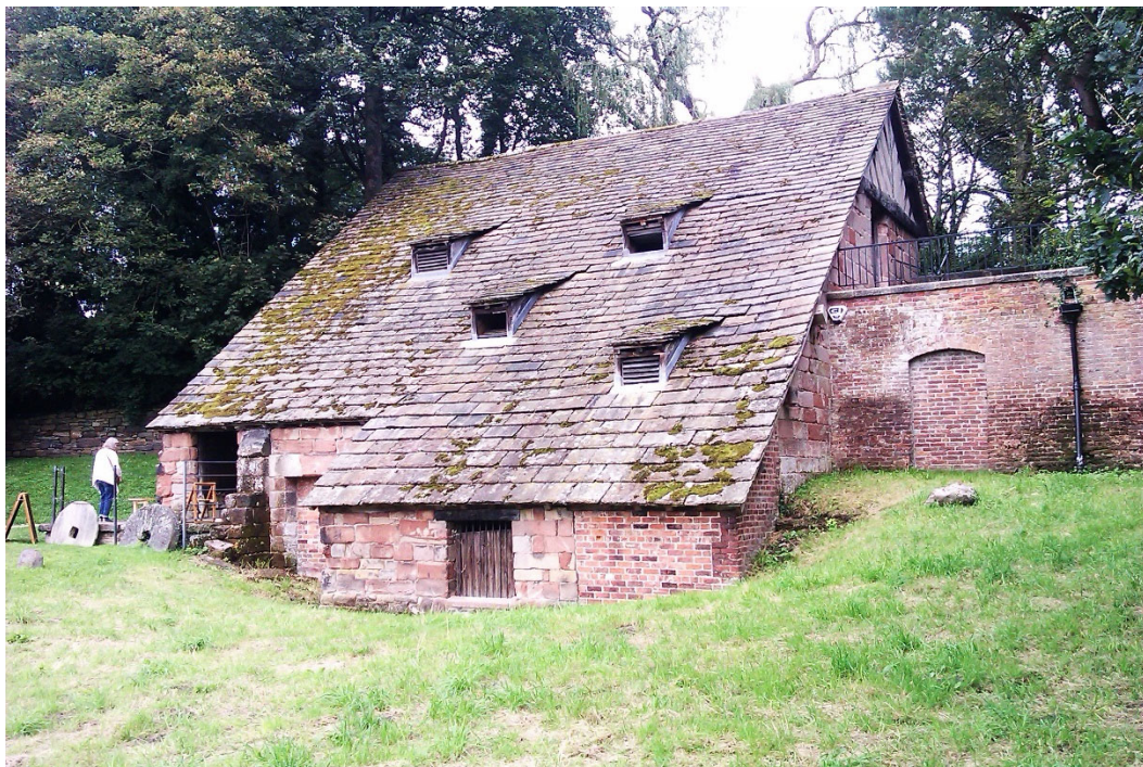
Figure 4: A restored overshoot mill of 16th century origin (NT) with mill pond on a higher level in the background, Nether Alderley, Cheshire
