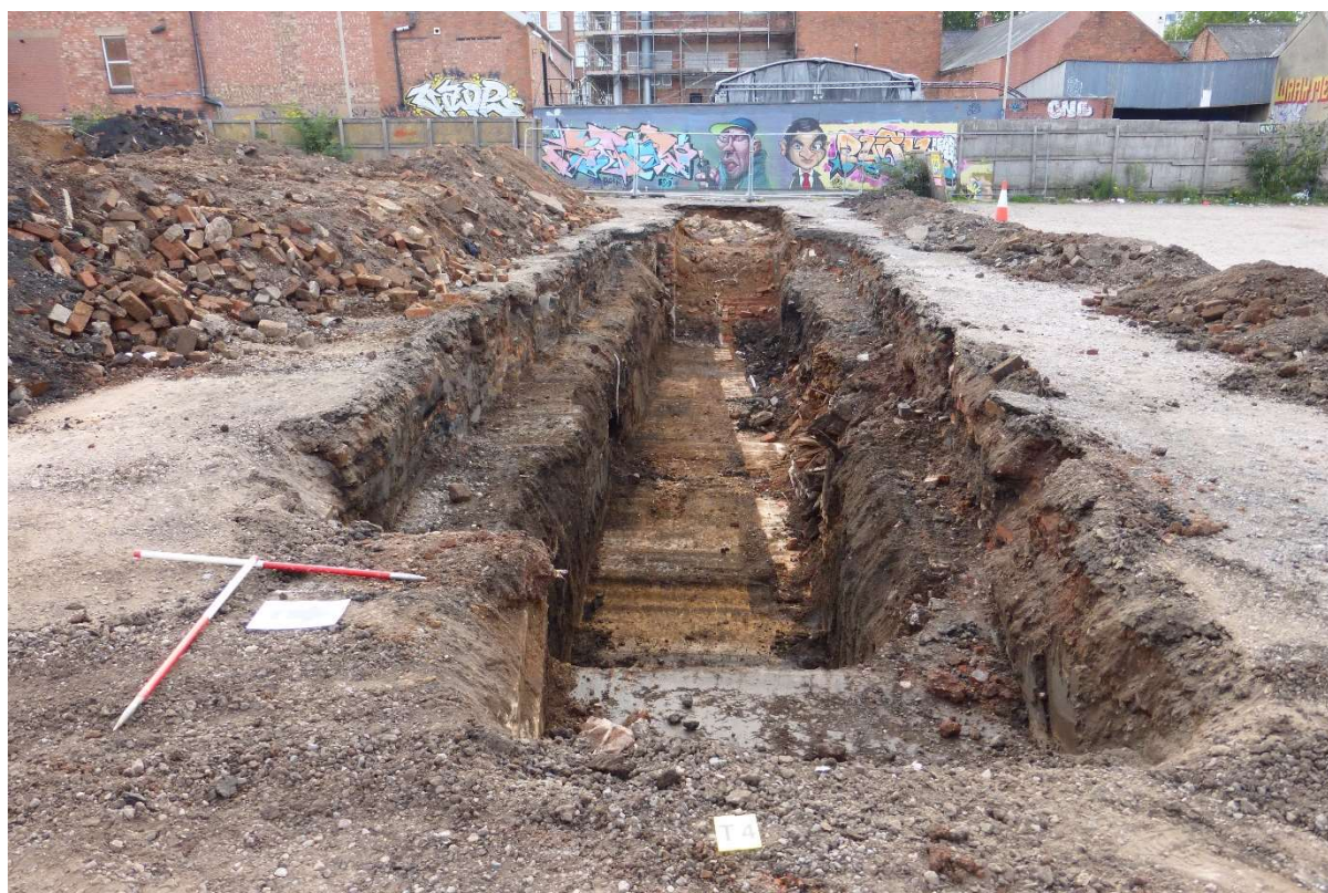
Figure 11: Trench 4 from the north-east. Backfilled cellars are visible to the right and in the background.
