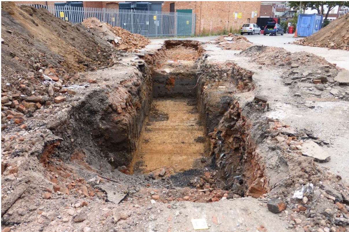
Figure 10: Trench 3 from the north-west. Backfilled cellars are visible in the foreground and background.
