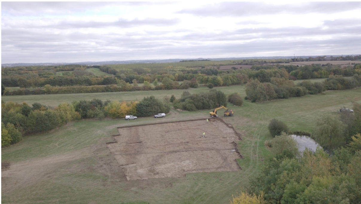
Figure 29: Aerial view of Area B, with work in progress, looking south-east
