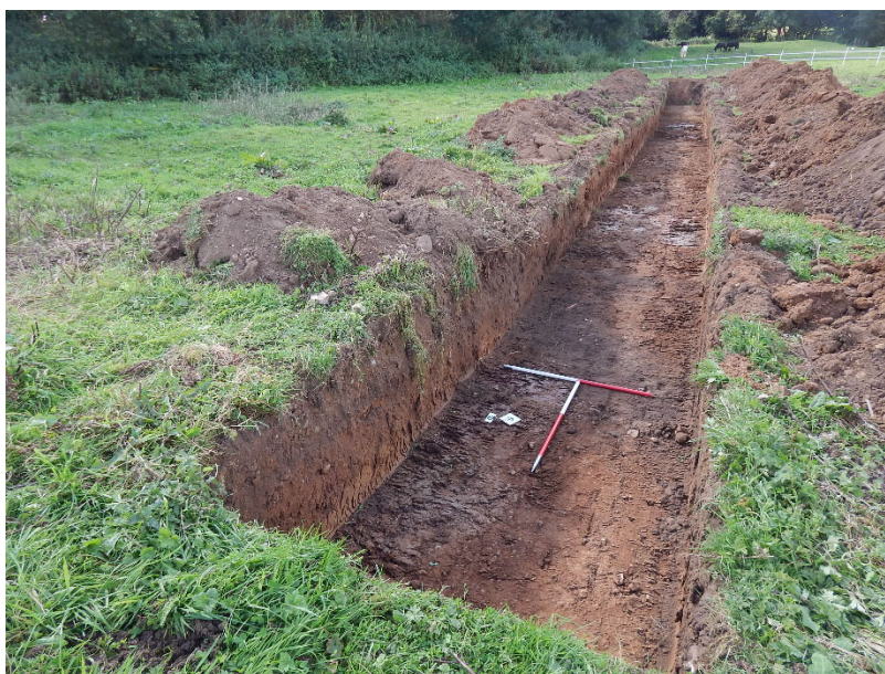
Figure 12: Trench 6, post-excitation, looking north-west
