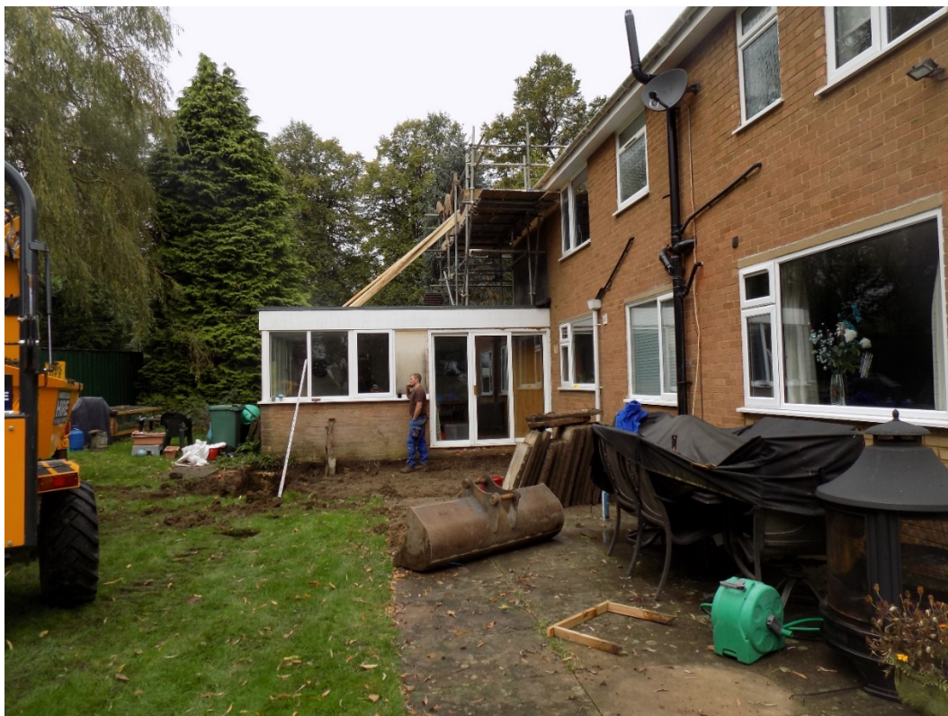
Figure 8: The development area (forward of machine bucket). Looking west.
