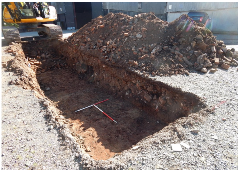
Figure 4: Trench 1, post excavation, looking east
