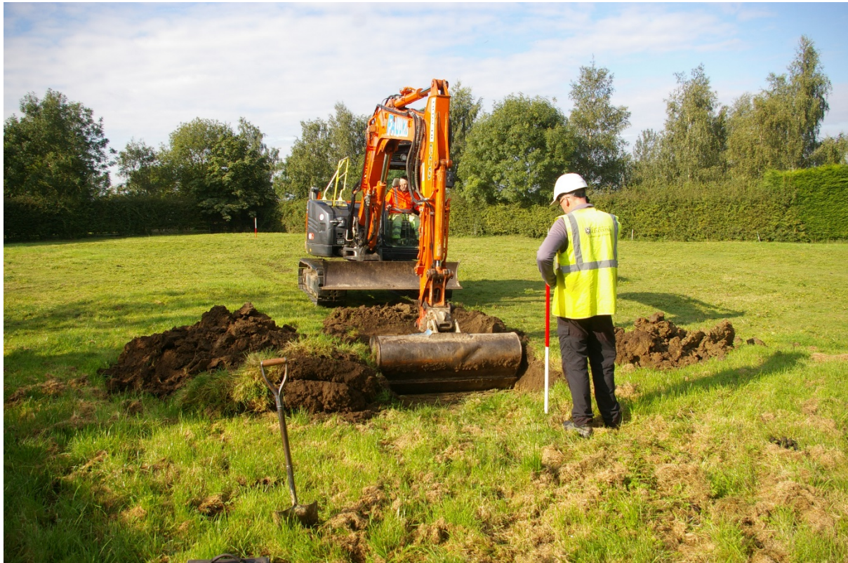
Figure 6: Work in progress.
