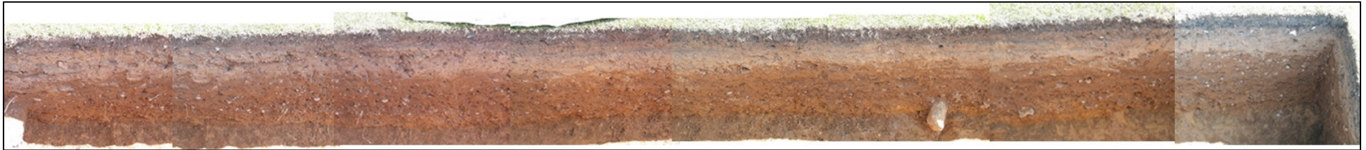
Figure 15: Composite photograph of west facing section.
