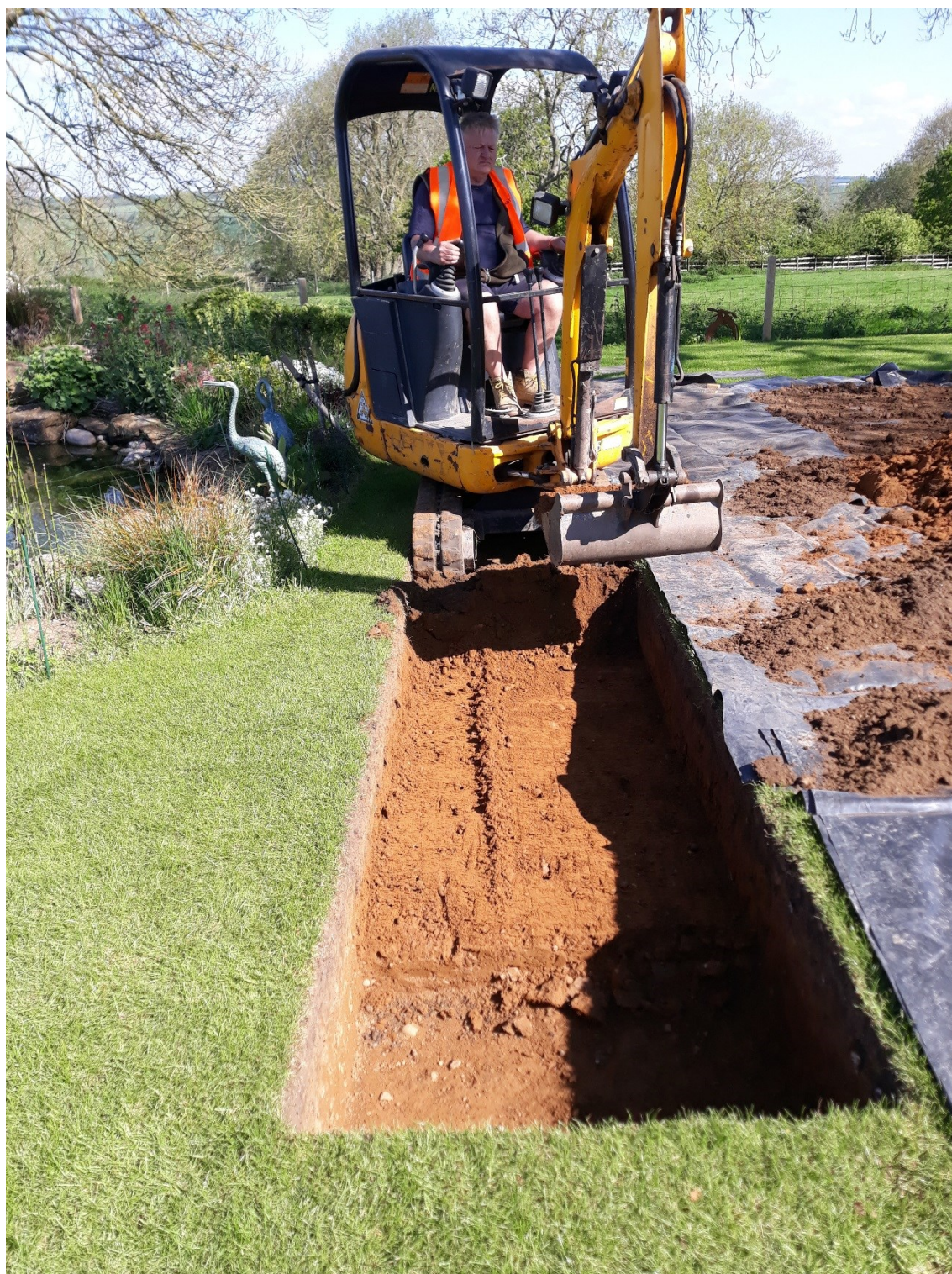
Figure 6: Mini-digger excavating top and sub soil to 0.5m. Looking north.
