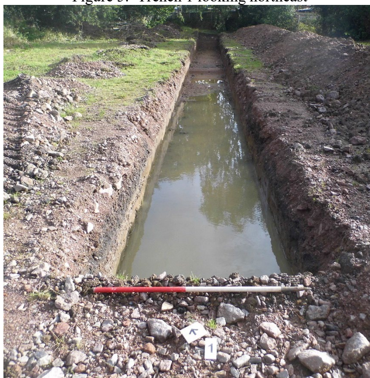
Figure 6: Trench 1 looking northeast and flooded
