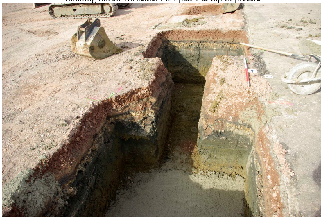
Figure 10 Post pad 23 Looking north. 1m scale
