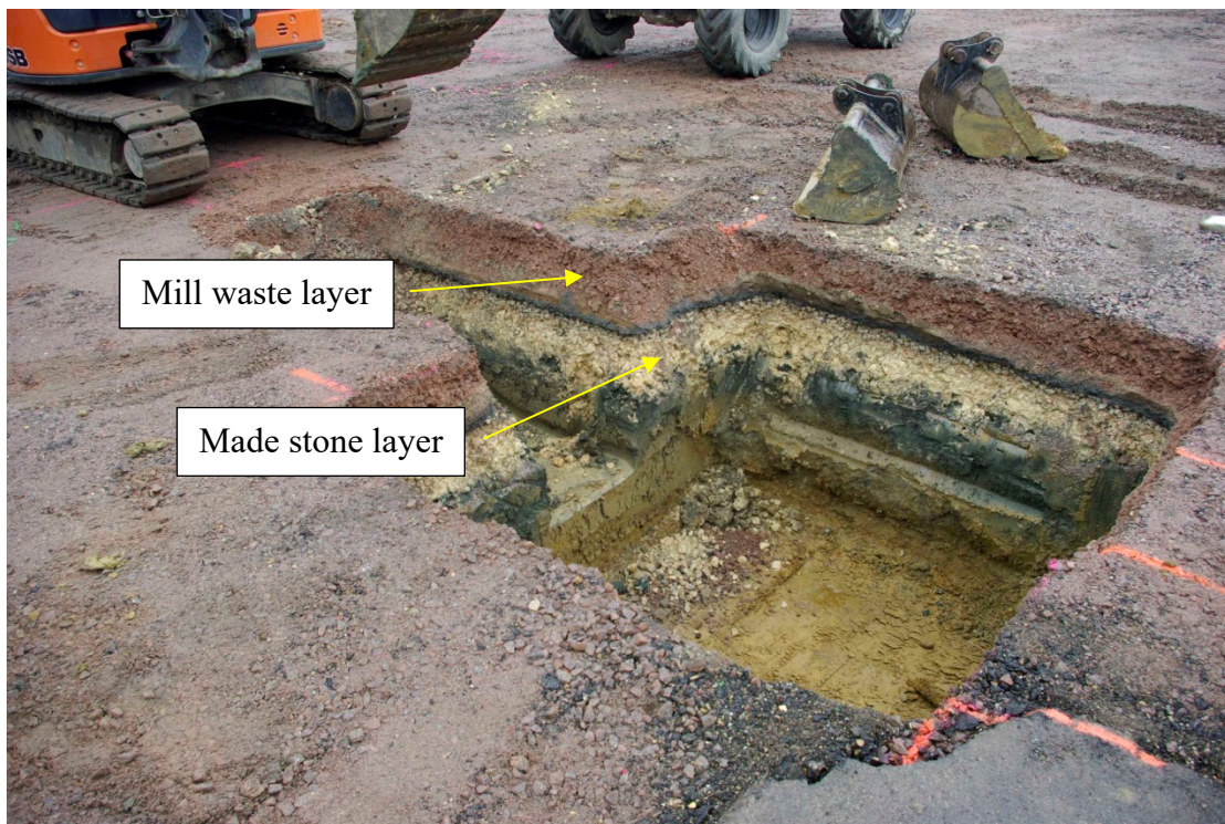
Figure 8 West end of post pad number 9 during excavation Looking south-east
