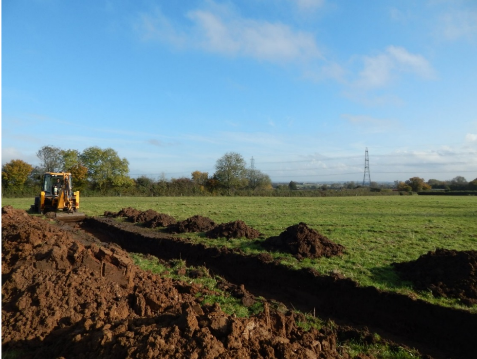
Figure 4: Work in progress on Trench 01, looking east
