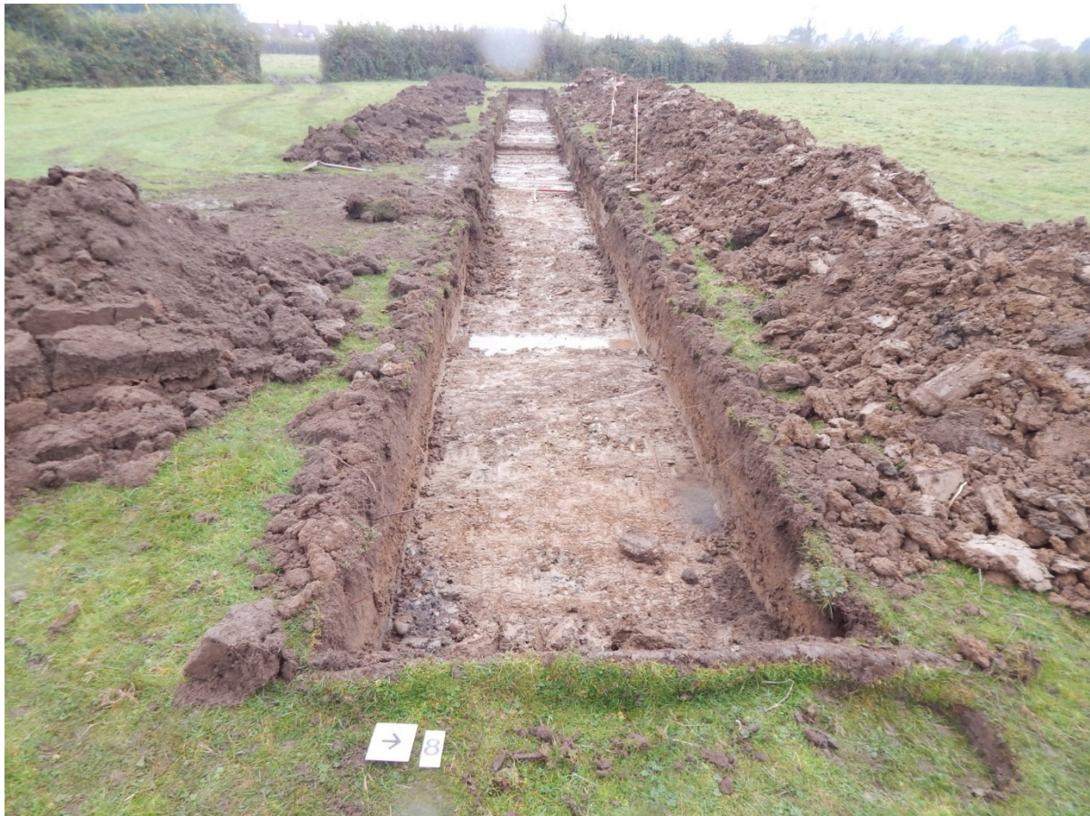
Figure 12: Trench 08, post-excavation, looking west
