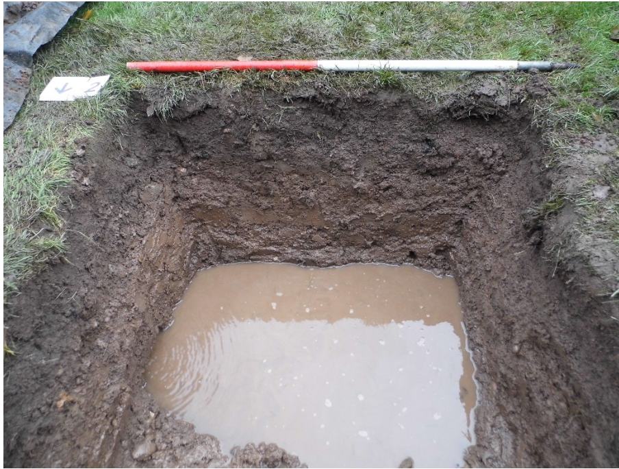
Figure 5: Test pit 2 looking south (beginning to flood)
