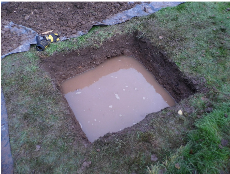
Figure 6: Test pit 2 flooded
