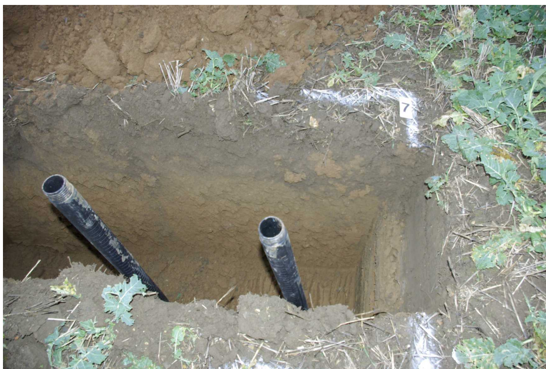
Figure 12 TP107 fully excavated Looking south
