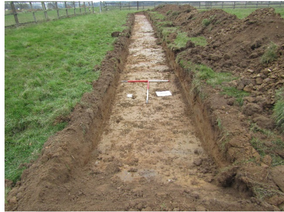
Trench 2 Facing west
