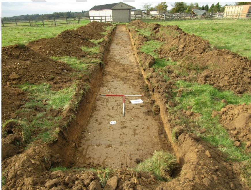
Figure 9: Trench 4 looking north-west
