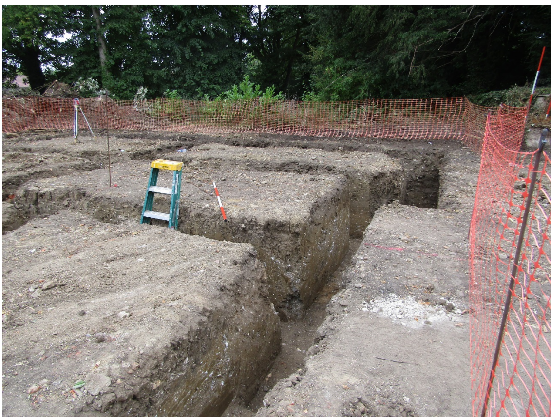
Figure 8: Excavated foundation trenches, looking west towards the church.
