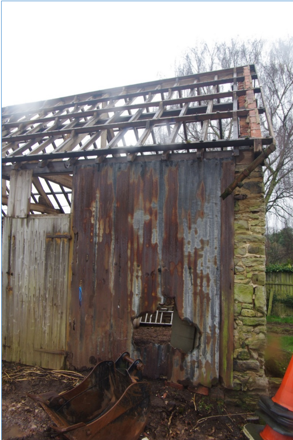
Figure 9 North elevation, west end. Note superstructure over rafters for corrugated sheets
