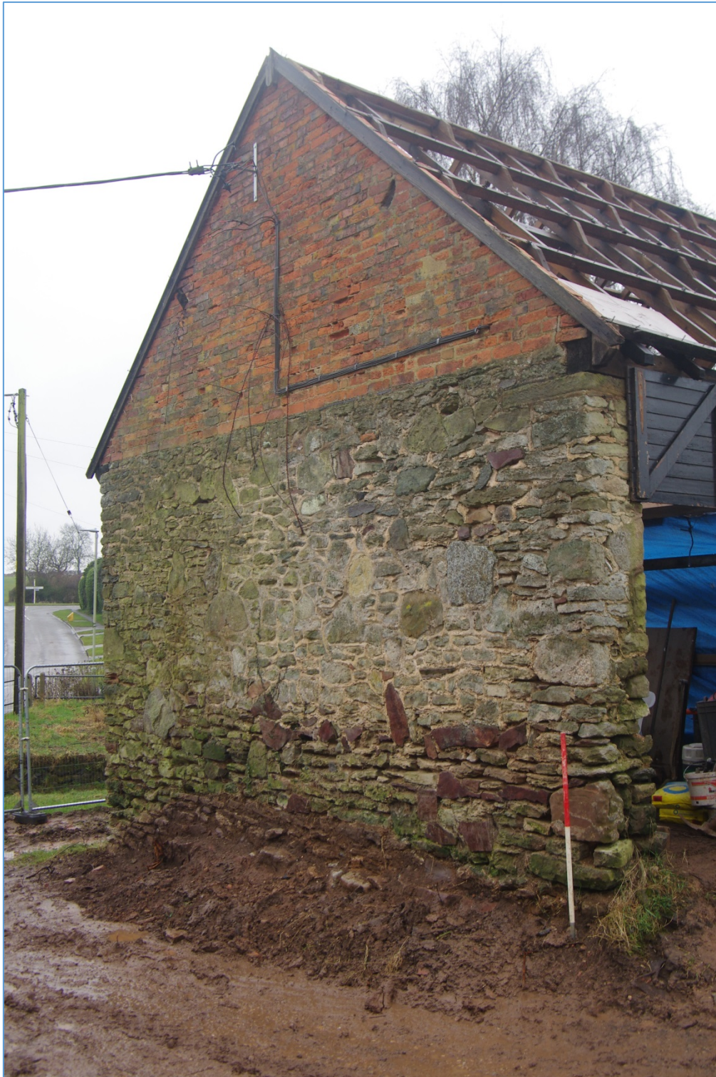
Figure 4 East wall. Note broken millstone centre left in the masonry
