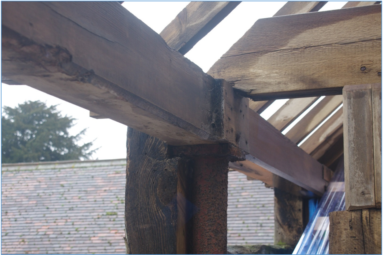
Figure 14 junction of tie beam, lintel, column
