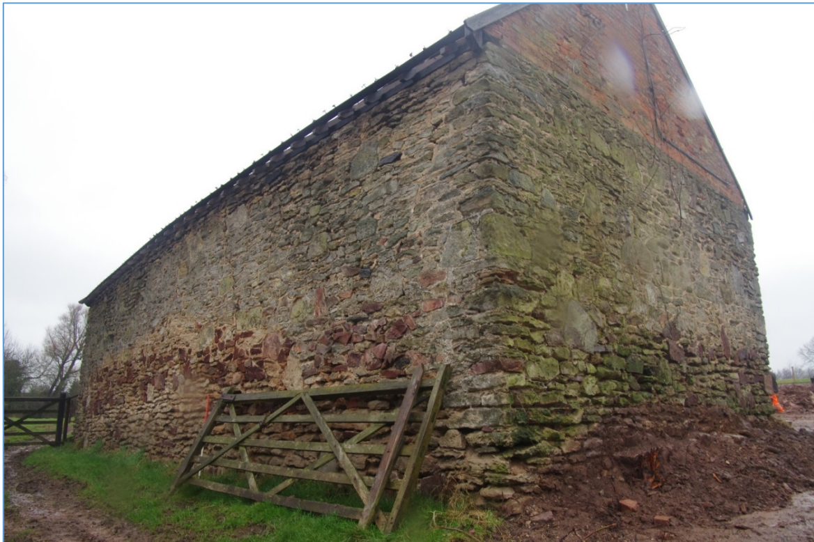
Figure 6 South, and east walls
