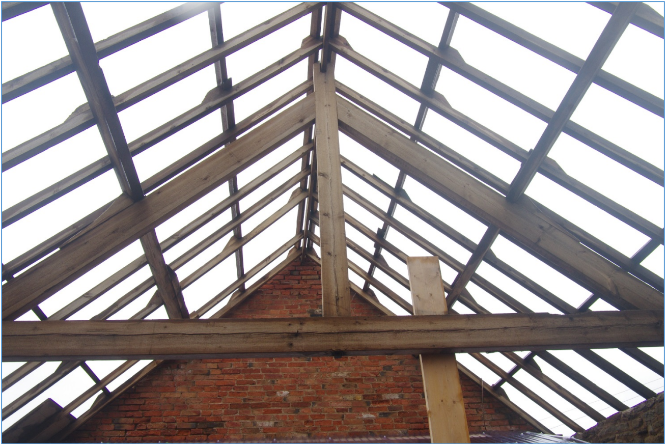
Figure 10 Roof structure, looking west
