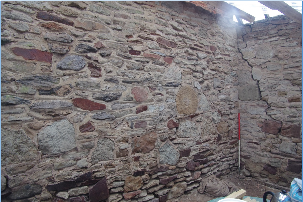
Figure 5 East wall, internal, looking south east
