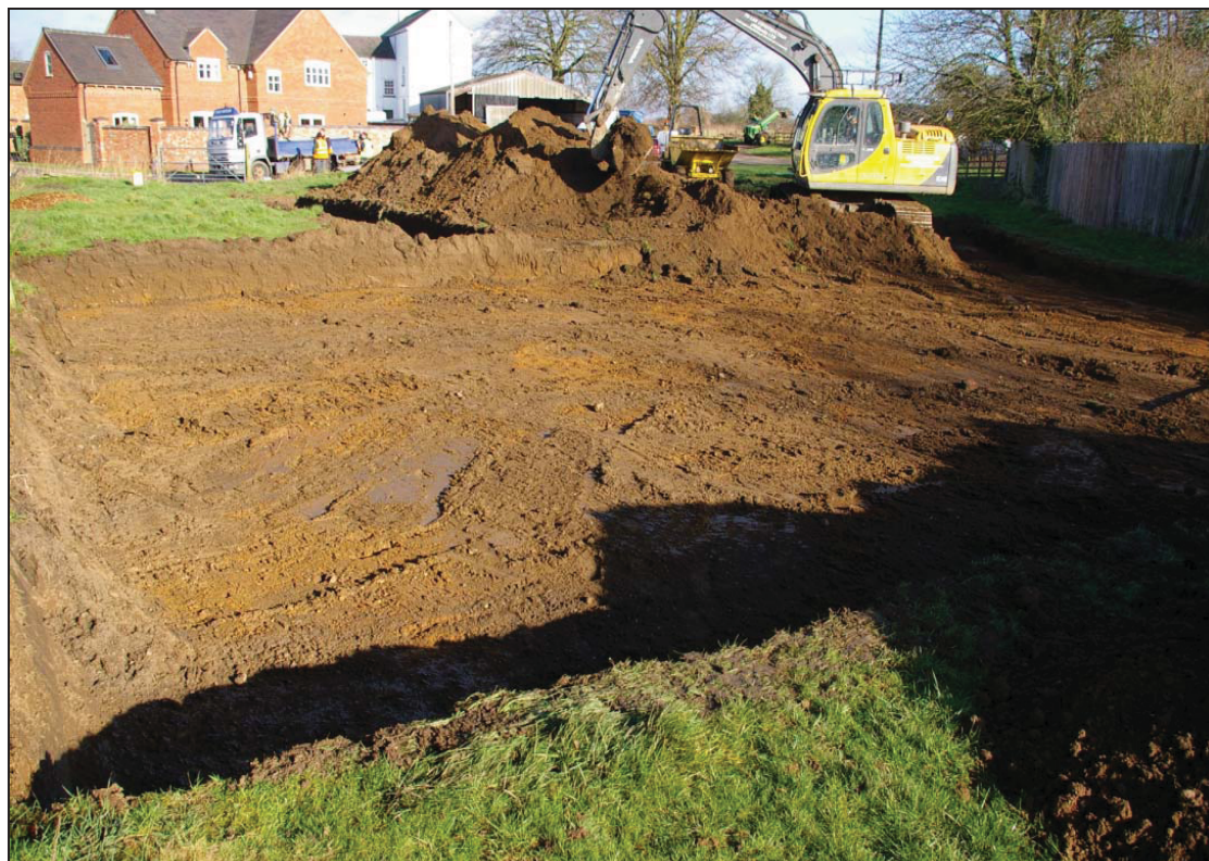
Figure 5: General view of ground reduction looking northeast
